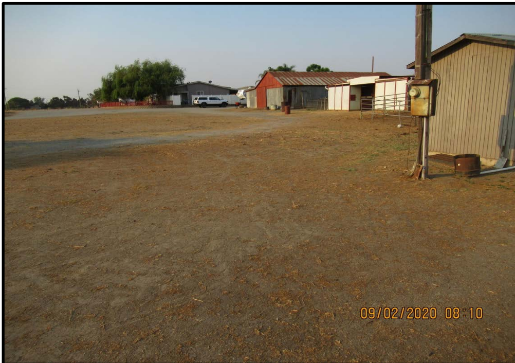
Home site and other structures in the west part of the site, looking south from the north part of the site; 09/02/20.
