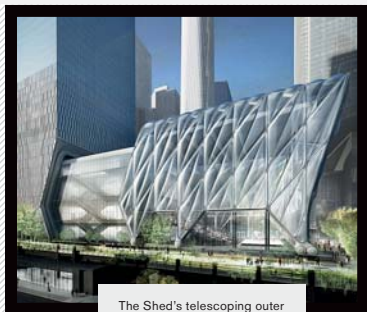
The Shed's telescoping outer shell sits on rails and can be expanded and contracted
