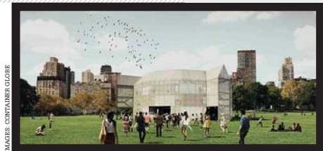
The galleries, stage and backstage areas will be built using shipping containers
