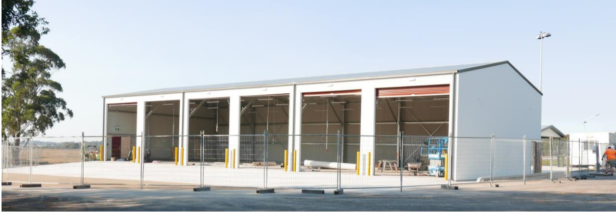
Image 5: CVRFS base at CVRA under construction (2018)
