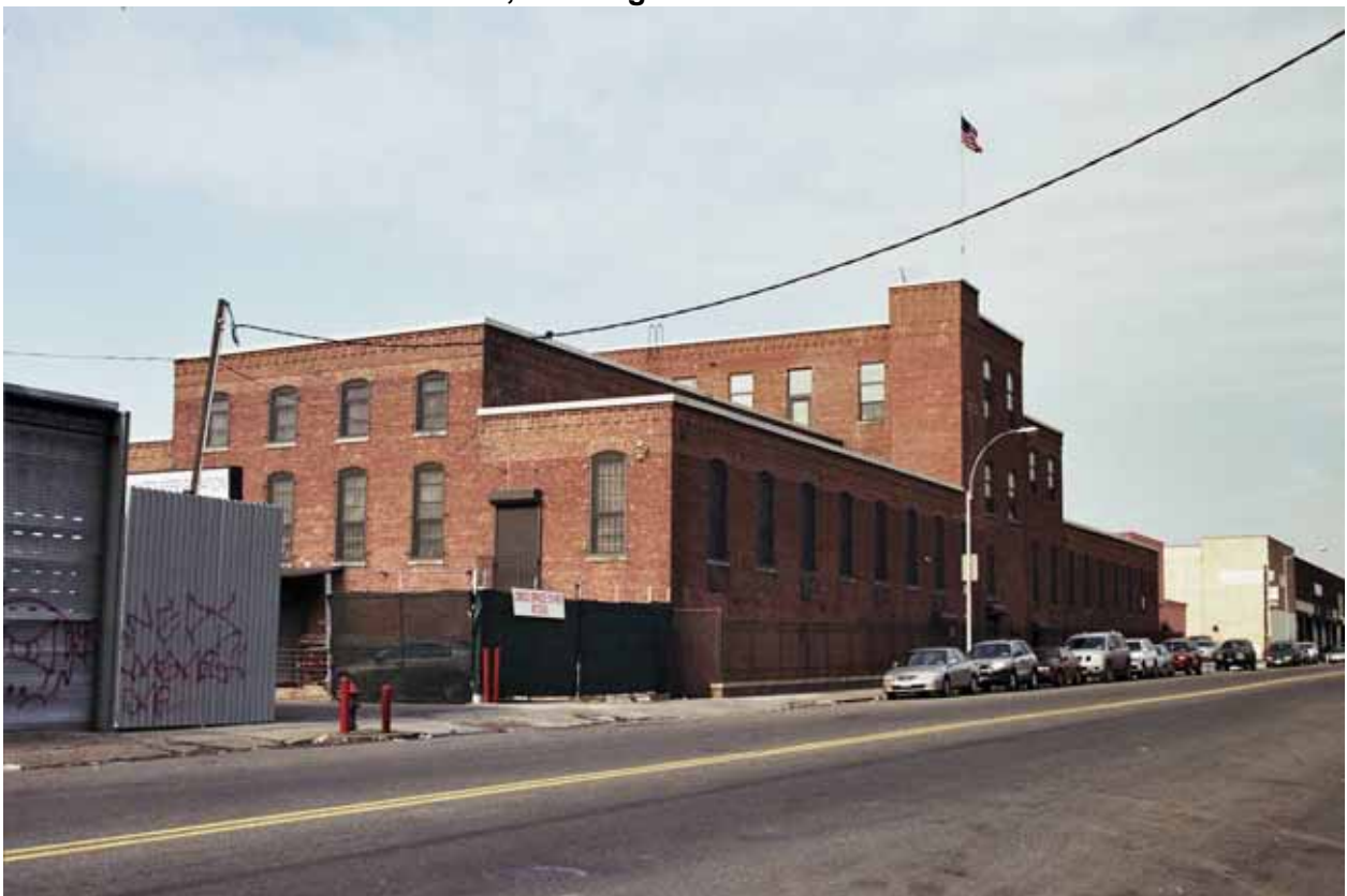
Photo V-82. 36-60 Review Avenue, Looking Northwest
