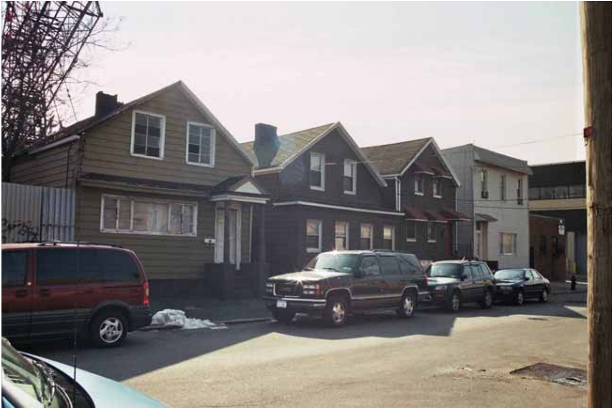
Photo V-93. 54-09, 54-11, 54-13, and 54-17 43rd Street, Looking Southeast
