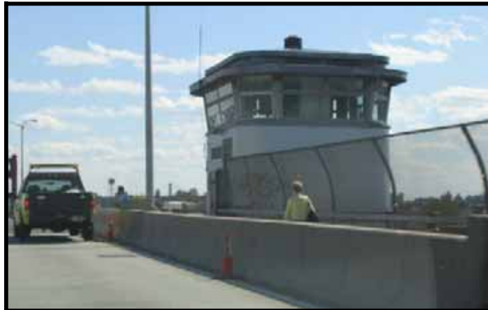
Image 16: Pulaski Bridge, Greenpoint, Brooklyn, New York
