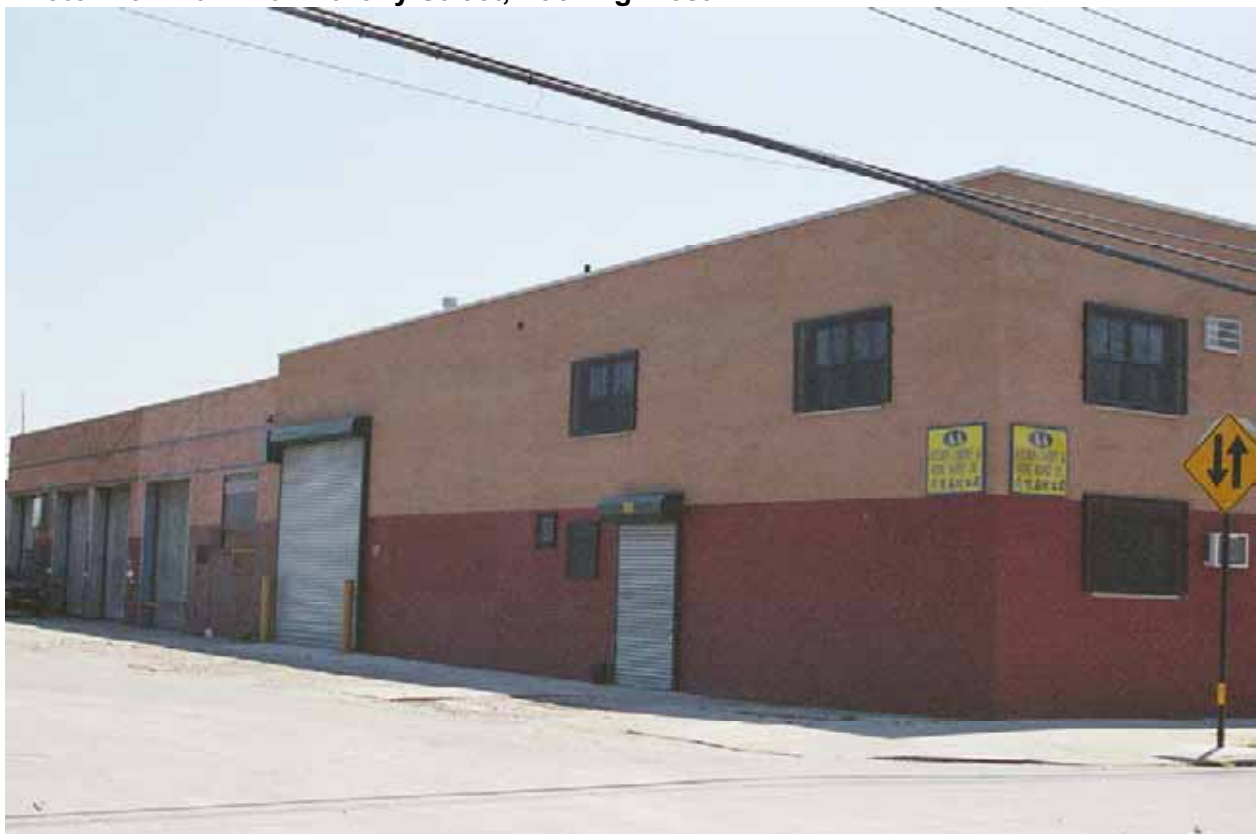
Photo V-62. 104-110 Anthony Street, Looking Southwest
