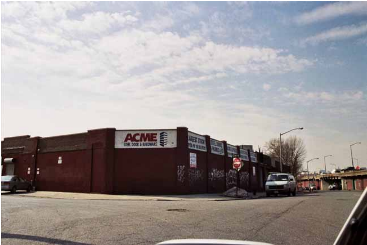
Photo V-65. 503-513 Porter Avenue, Looking Southwest Along Cherry Street
