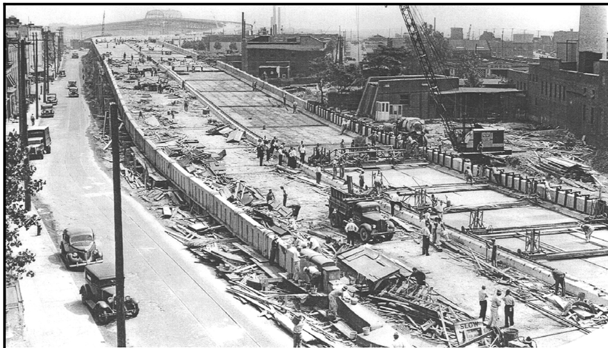
Image 7: Meeker Avenue Bridge Under Construction
