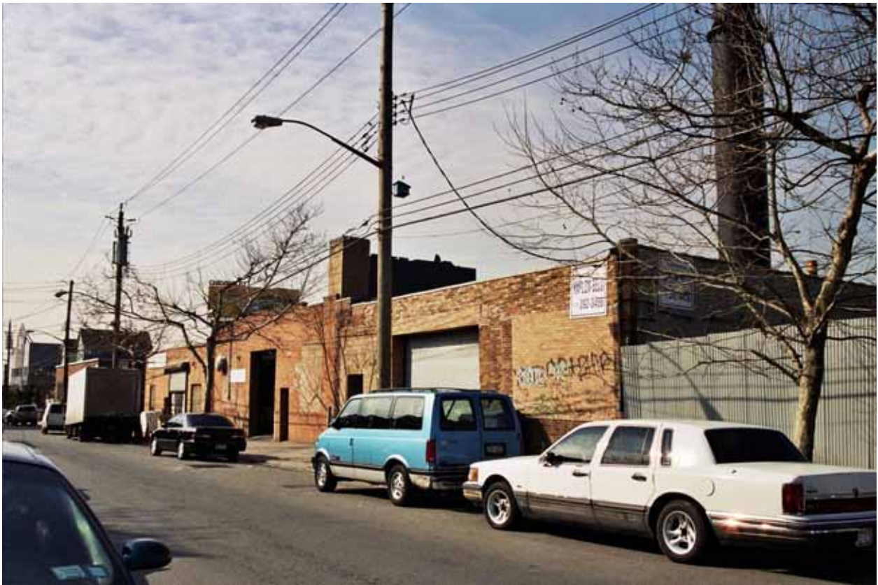
Photo V-95. 54-08, 54-14 and 54-18 43rd Street, Looking Southwest
