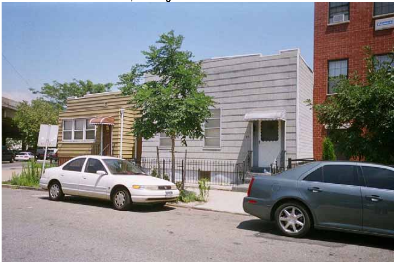
Photo V-25. 60 Monitor Street, Looking Northeast
