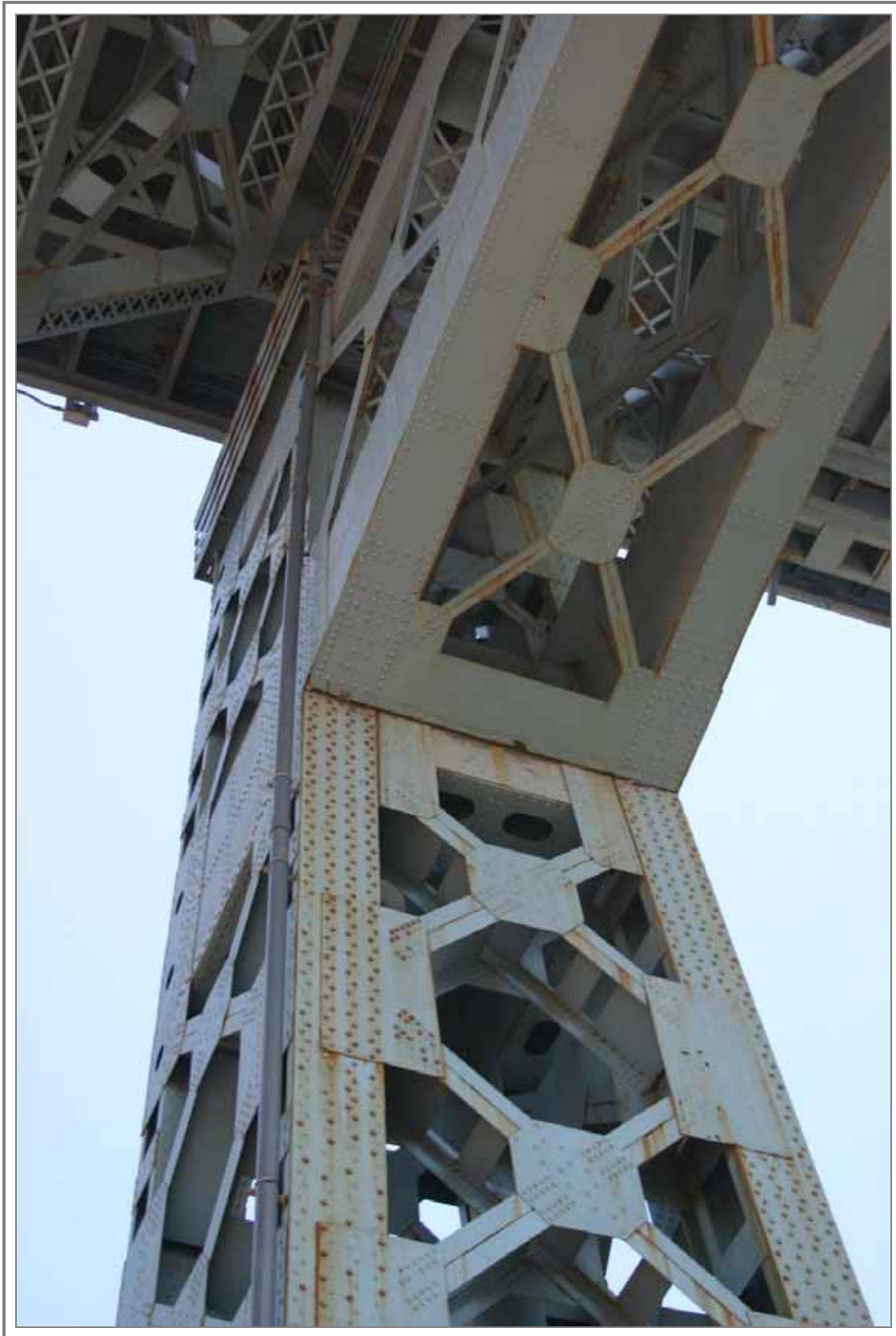
Detail of truss connection beneath Kosciuszko Bridge
