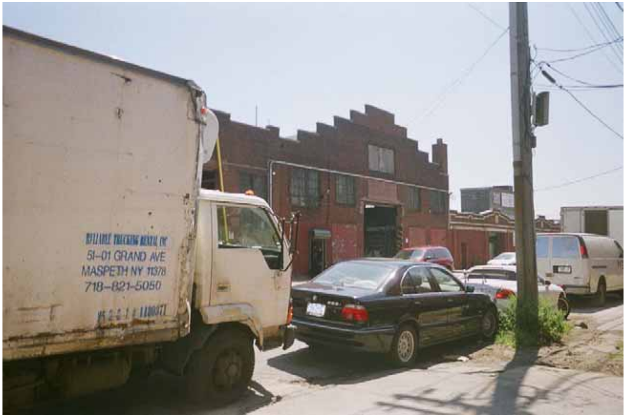
Photo V-55. 38 Anthony Street, Looking Southwest
