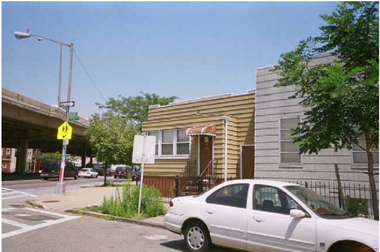
Photo V-24. 62 Monitor Street, Looking Northeast
