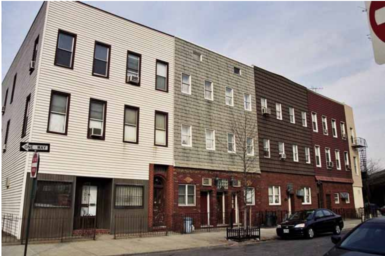
Photo V-22. 197-203 Engert Avenue and 621 Meeker Avenue, Looking North
