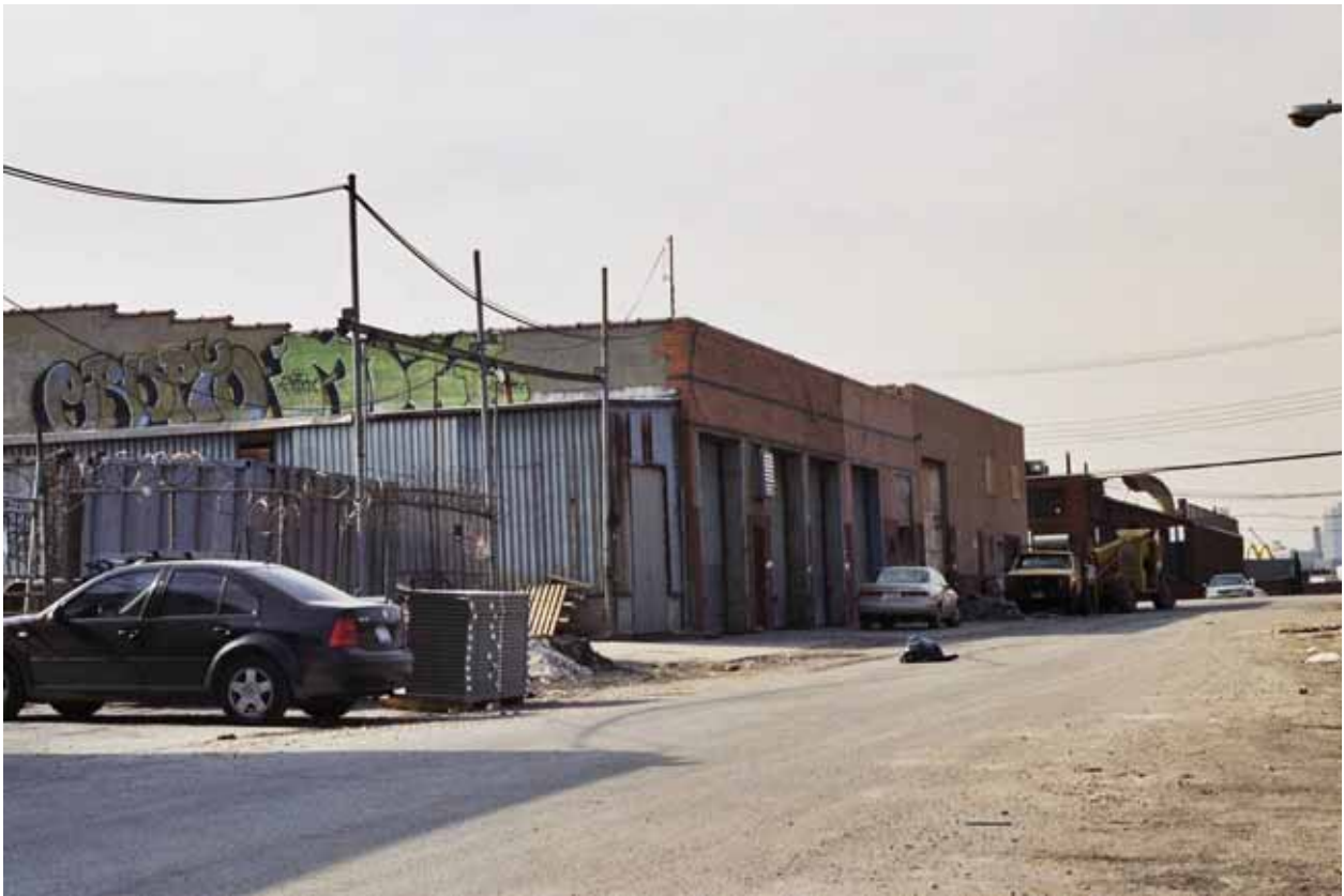
Photo V-59. 72 Anthony Street, Looking Southwest
