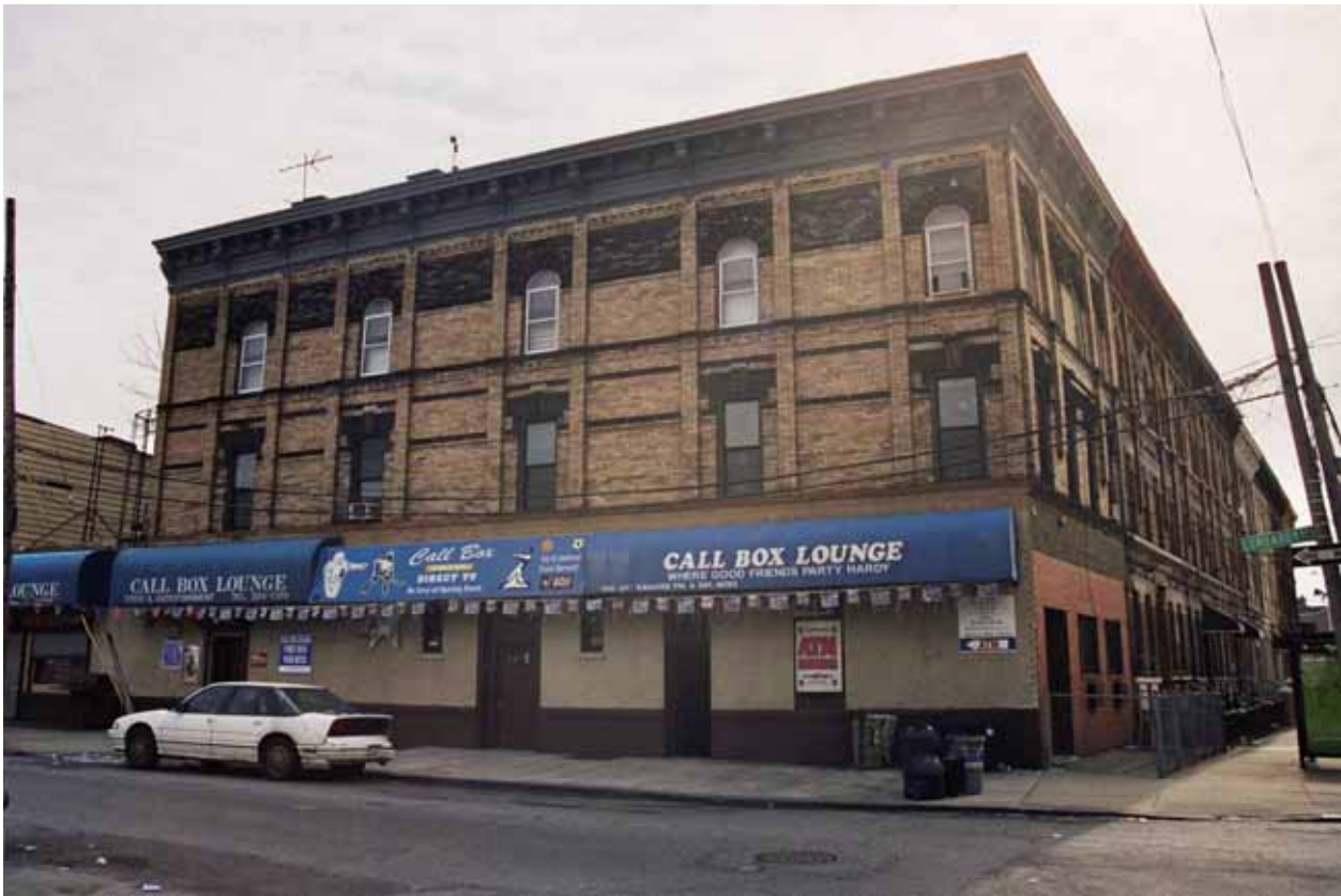
Photo V-47. 148 Kingsland Avenue, Looking South
