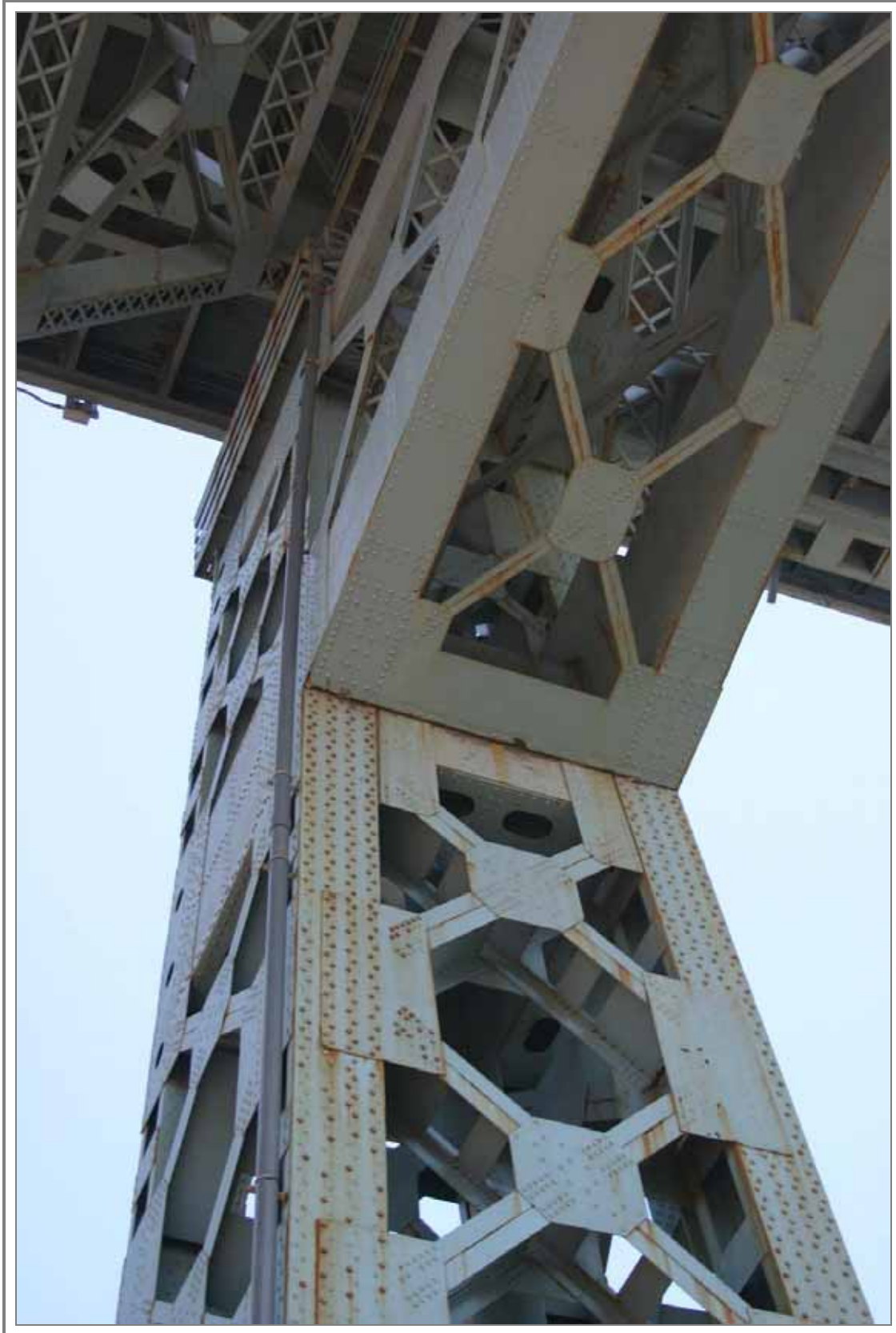
Photo V-20. Detail of truss connection beneath Kosciuszko Bridge
