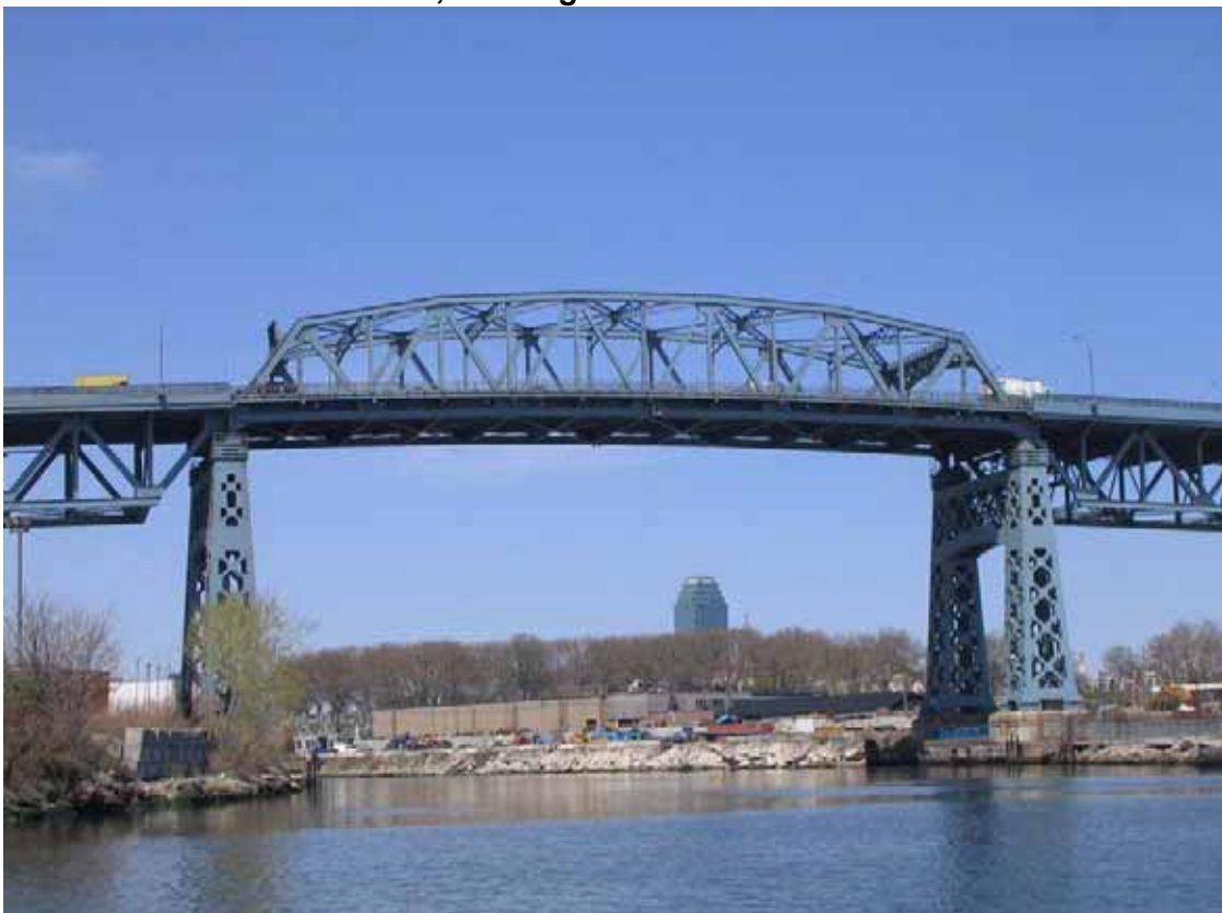
Photo V-98. Kosciuszko Bridge, Looking Northwest
