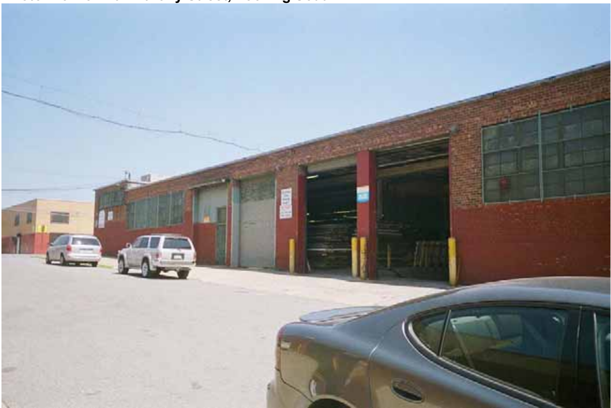
Photo V-58. 54-70 Anthony Street, Looking Southwest
