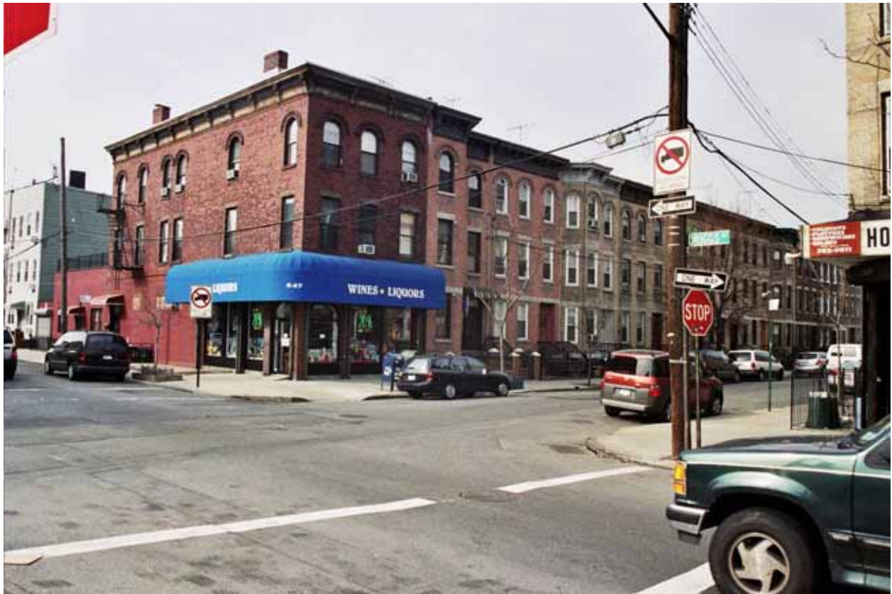
Photo V-43. 14-24 Driggs Avenue, Looking Northwest
