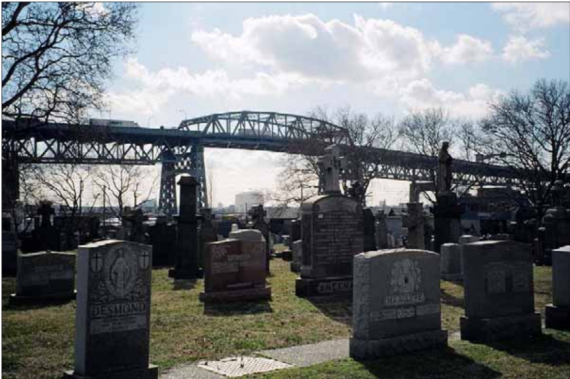
PHOTO 8: VIEW OF THE KOSCIUSZKO BRIDGE FROM CALVARY CEMETERY
