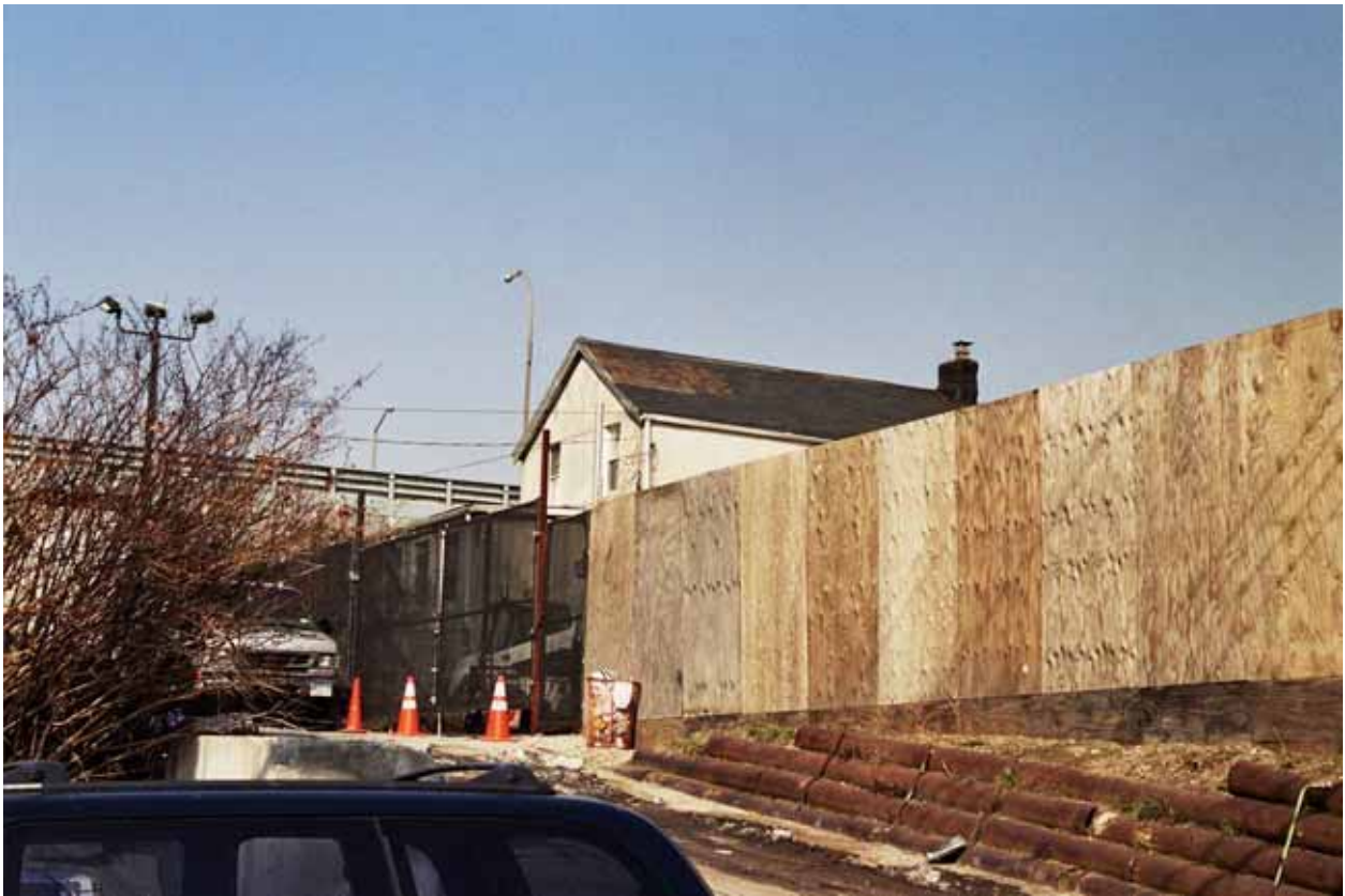
Photo V-97. 42-21 54th Drive, Looking West
