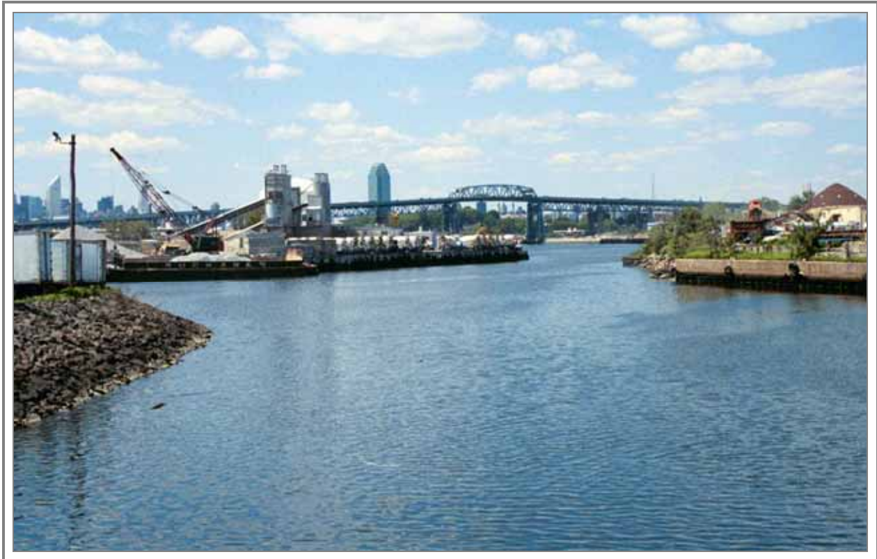
Kosciuszko Bridge, looking northwest from Grand Street Bridge
