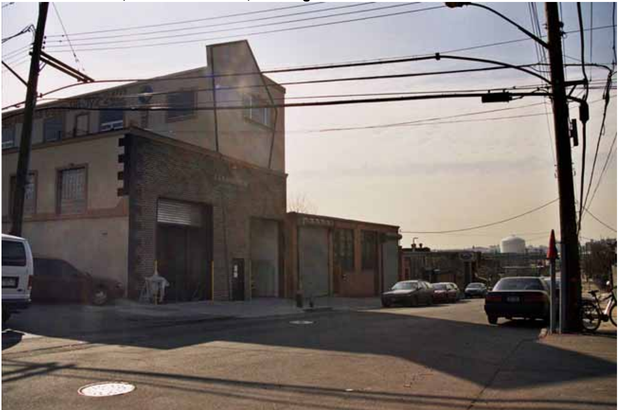
Photo V-90. 55-01 and 55-05 43rd Street, Looking Southeast
