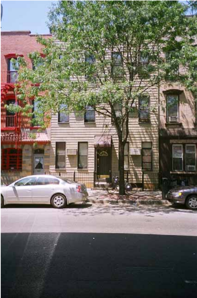
Photo V-26. 583 Meeker Avenue, Looking Northwest
