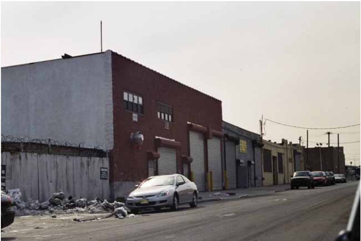
Photo V-38. 958-972 Meeker Avenue, Looking Southwest
