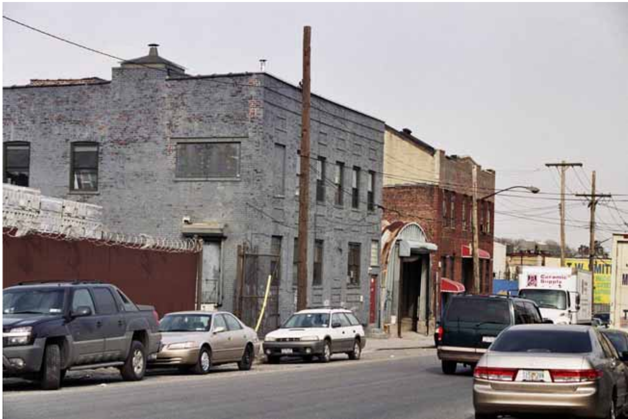
Photo V-34. 843-845, 855, and 857-869 Meeker Avenue, Looking Northeast
