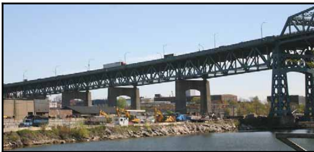
Image 24: Photo showing the multiple spans and deck truss of the Kosciuszko Bridge EHT Traceries, May 2006
