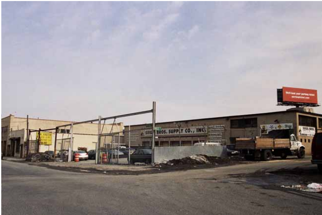
Photo V-36. 890-892 Meeker Avenue, Looking Southeast
