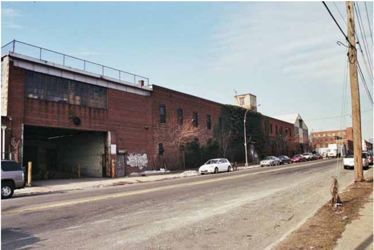
Photo V-81. 38-98 Review Avenue, Looking Southwest
