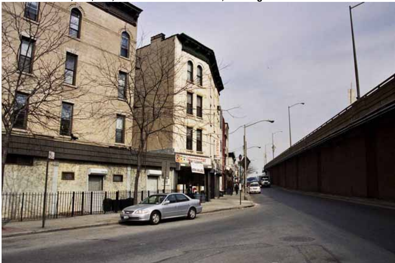
Photo V-29. 729, 733-735, and 737 Meeker Avenue, Looking Northeast
