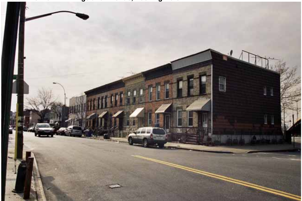
Photo V-46. 145-151 Kingsland Avenue, Looking South
