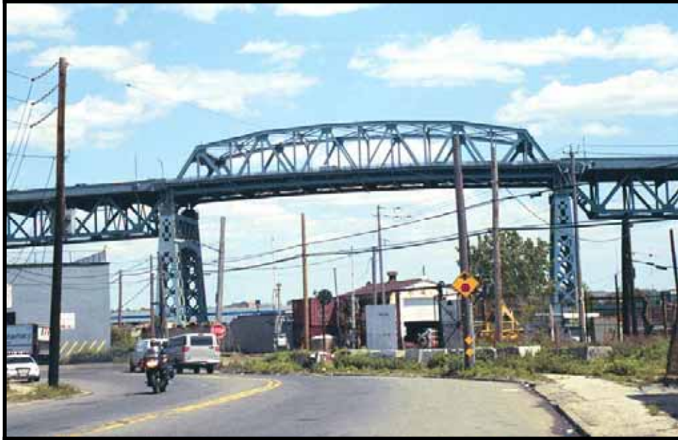
Image 26: Polygonal top chords and overhead bracing of the Kosciuszko Bridge EHT Tracerics, May 2006
