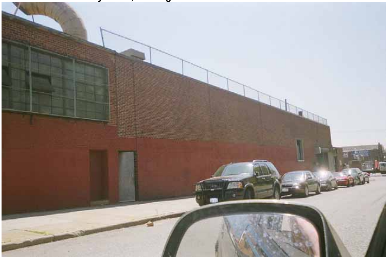
Photo V-56. 46-52 Anthony Street, Looking Southwest
