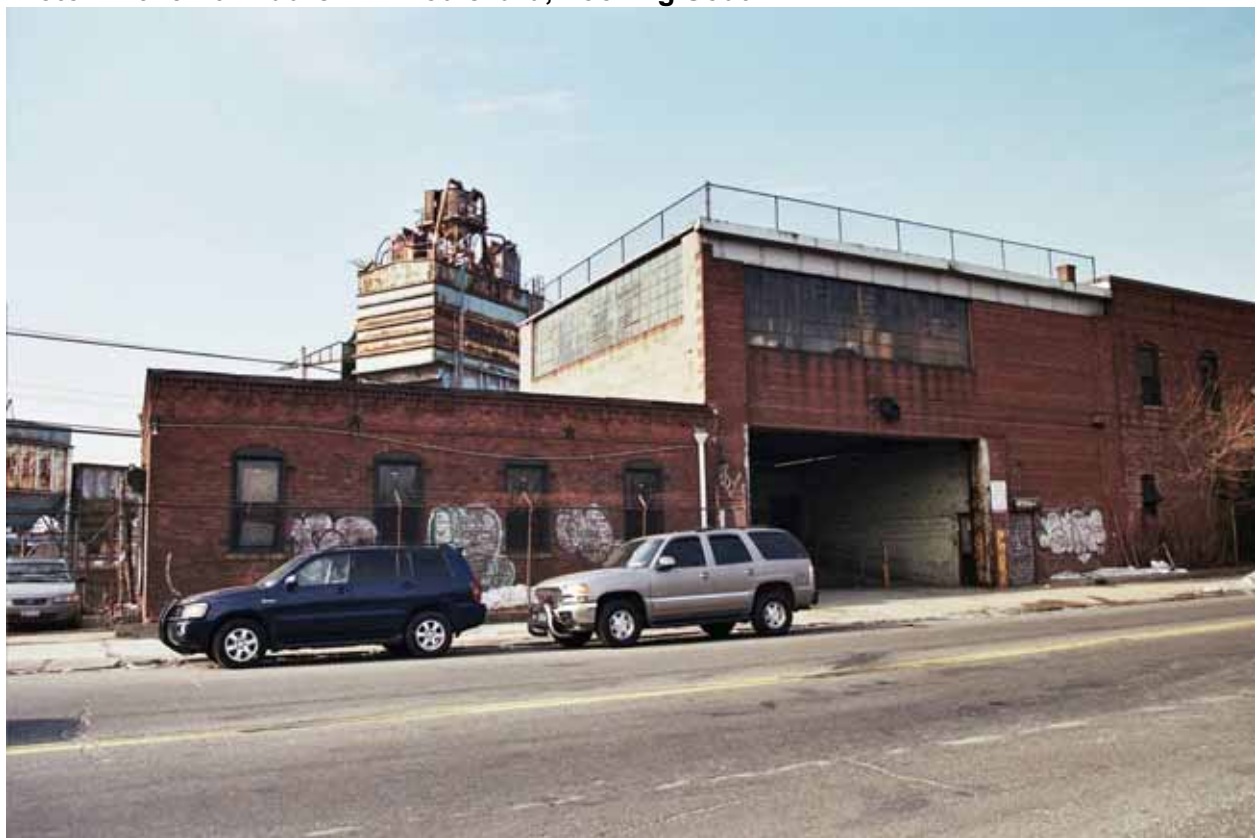
Photo V-80. 39-30 Review Avenue, Looking Southwest
