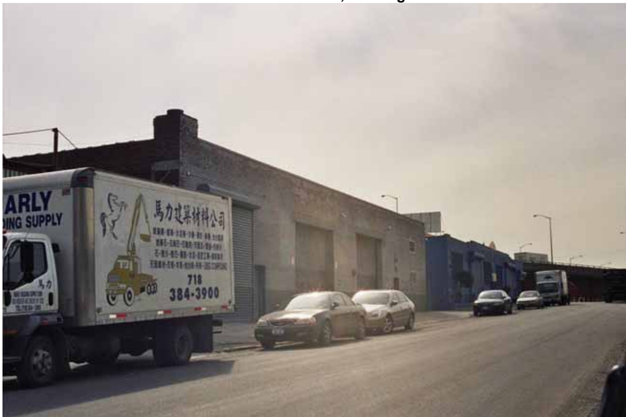
Photo V-33. 810-822 Meeker Avenue, Looking Southwest
