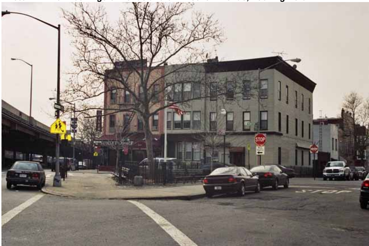
Photo V-23. 71-75 Monitor Street, Looking West
