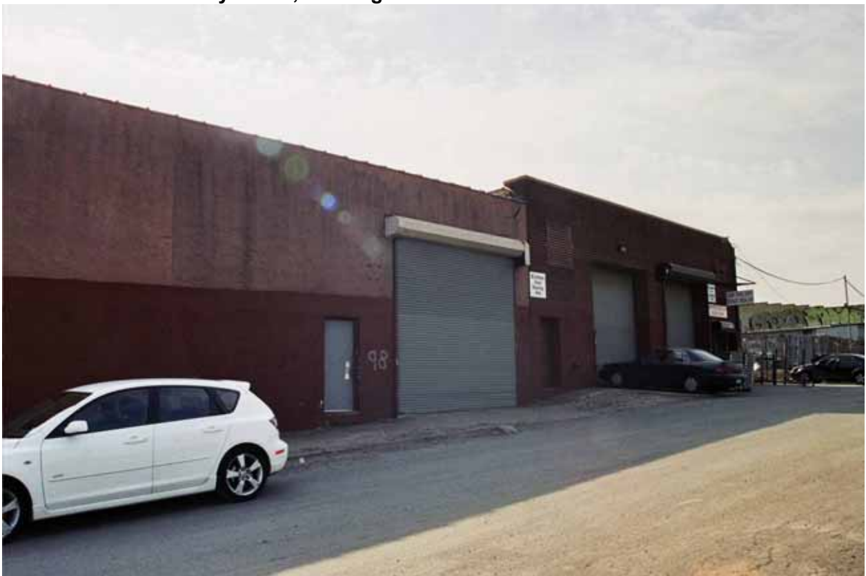
Photo V-60. 96-102 Anthony Street, Looking Southwest
