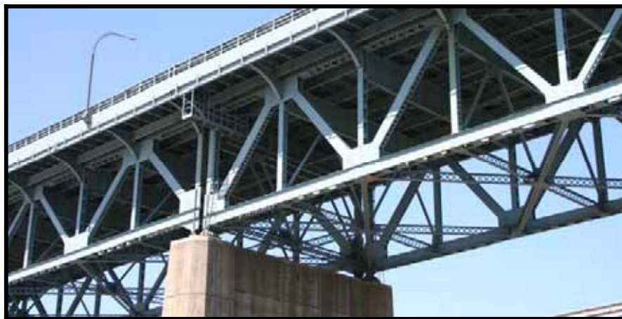
Image 25: Detail showing Warren deck truss of the Kosciuszko Bridge EHT Traceries, May 2006
