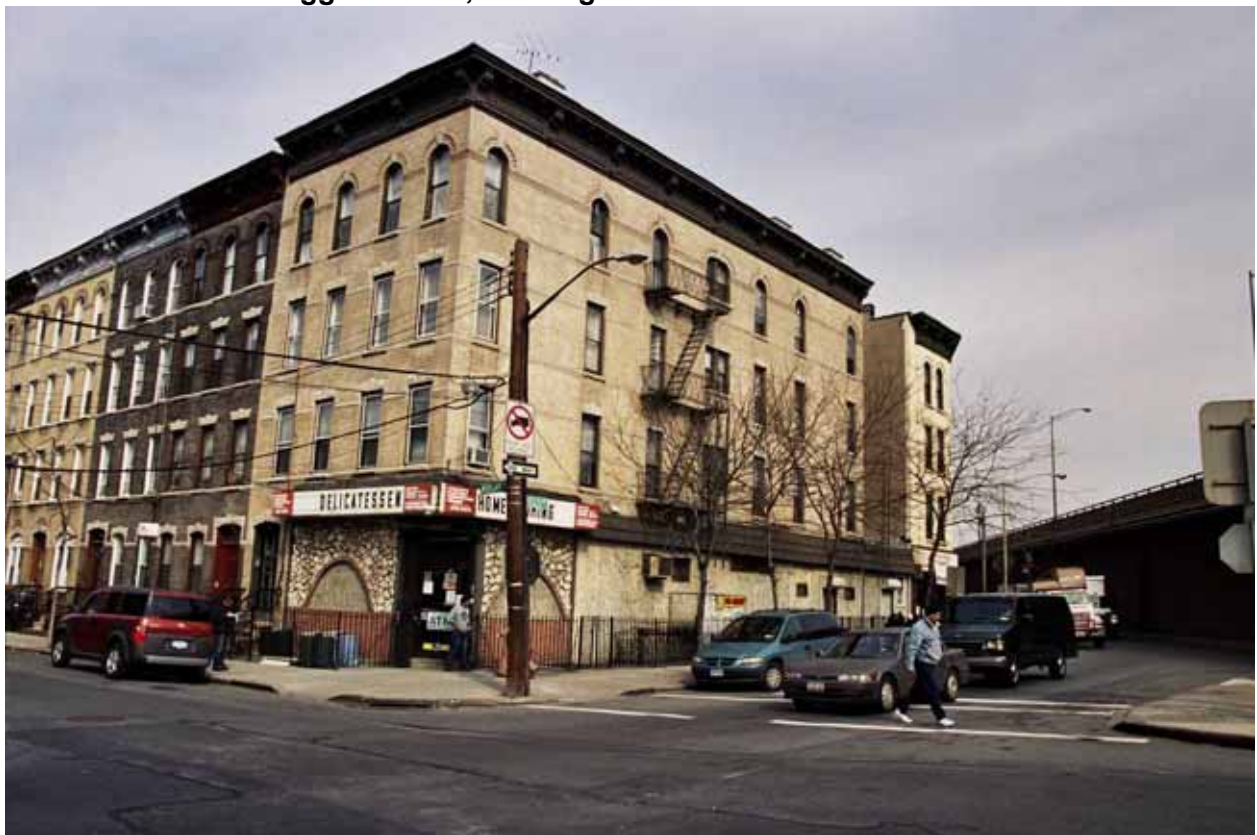
Photo V-44. 4 Driggs Avenue, Looking Northeast
