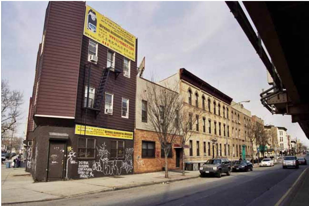
Photo V-28. 679, 685, 687, and 695 Meeker Avenue, Looking Northeast
