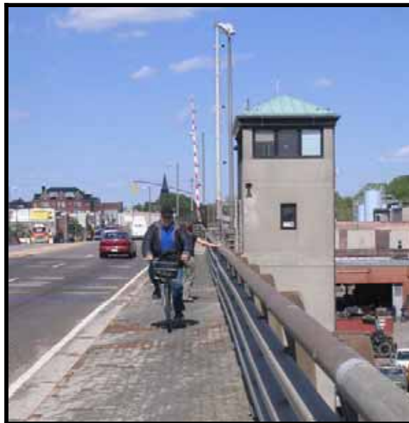
Image 18: Greenpoint Avenue Bridge, Greenpoint, Brooklyn, New York
