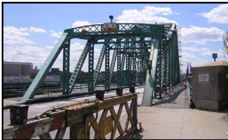
Image 17: Grand Street Bridge, Queens, New York
