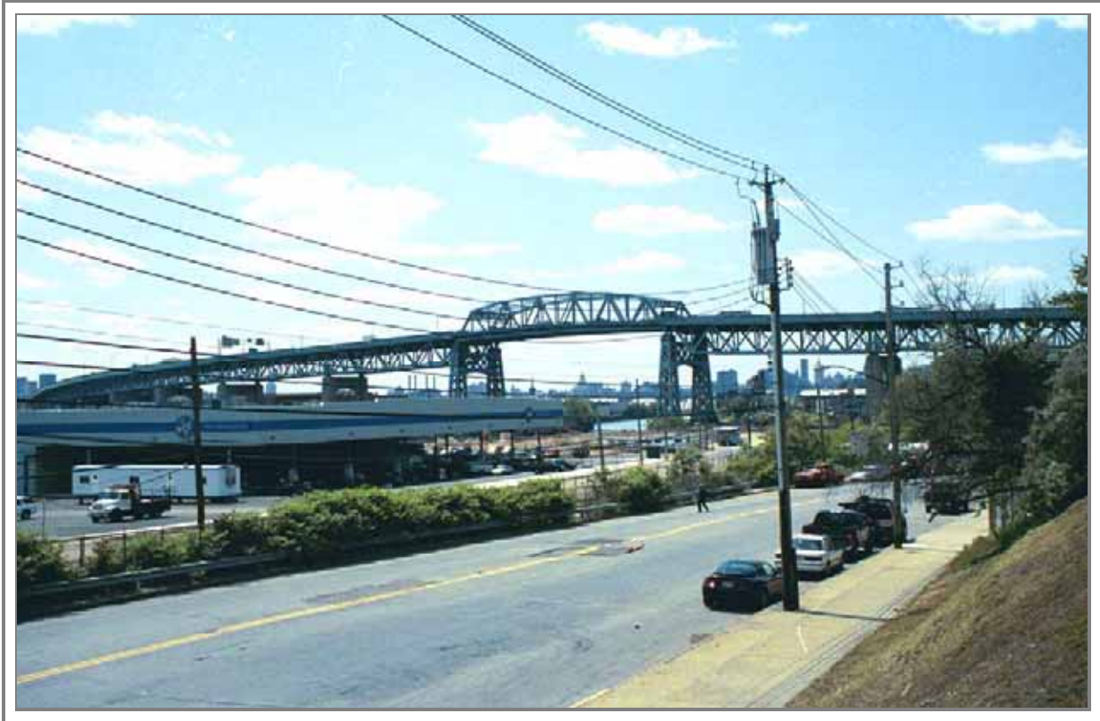
Kosciuszko Bridge, looking west from 56 th Road, Queens, New York
