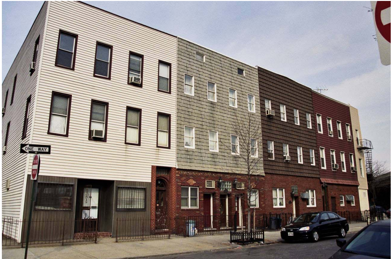
Photo V-22. 197-203 Engert Avenue and 621 Meeker Avenue, Looking North
