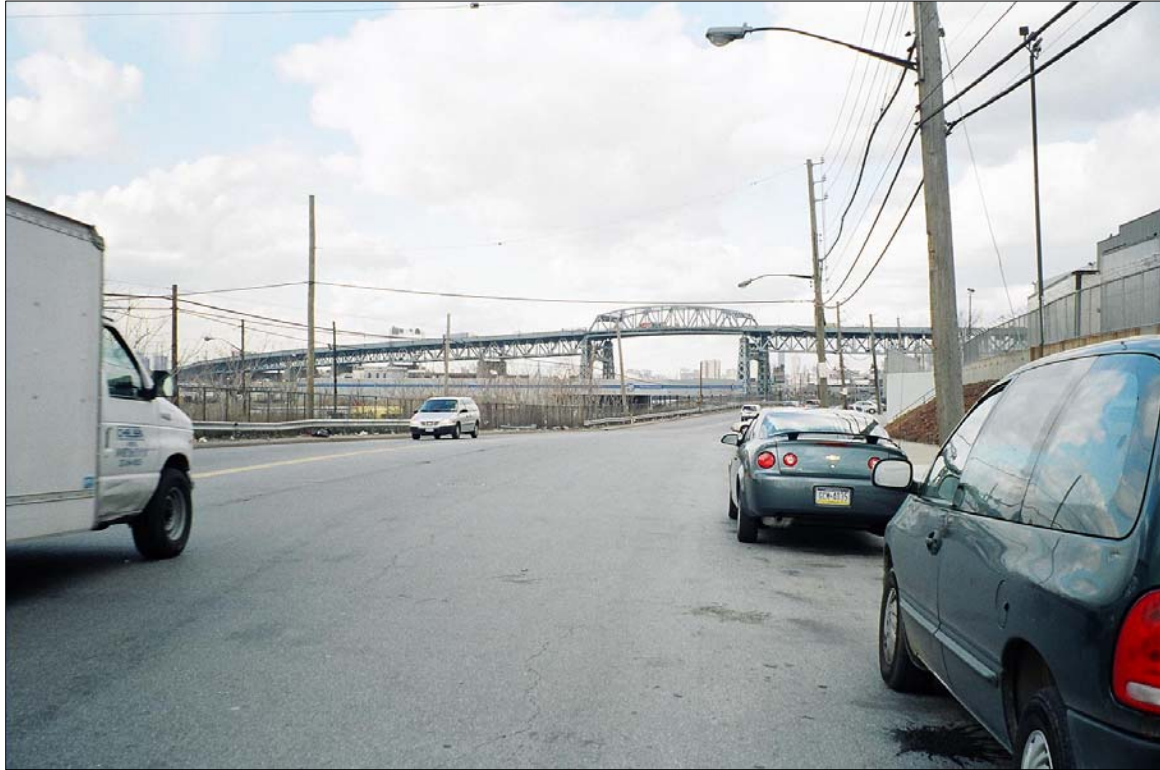
PHOTO 7: VIEW WEST ON 56 TH ROAD AT UPS FACILITY
