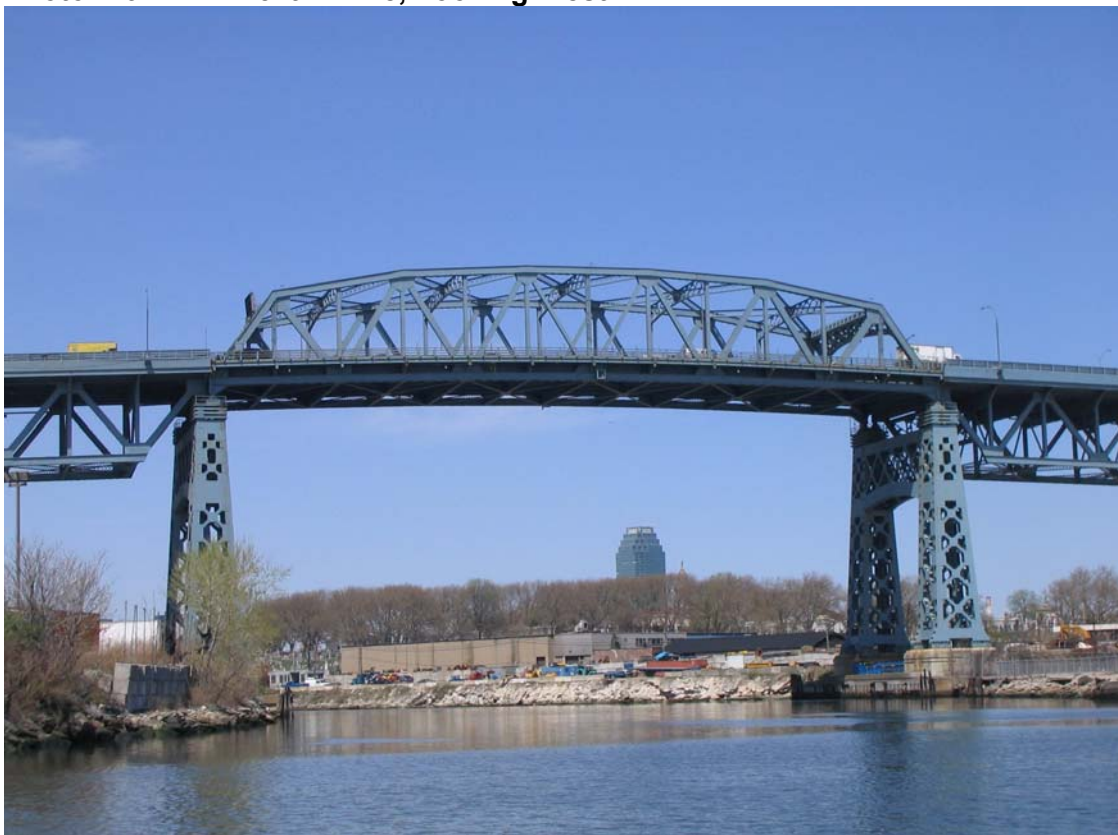
Photo V-98. Kosciuszko Bridge, Looking Northwest
