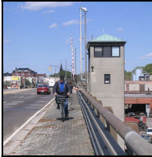
Image 18: Greenpoint Avenue Bridge, Greenpoint, Brooklyn, New York
