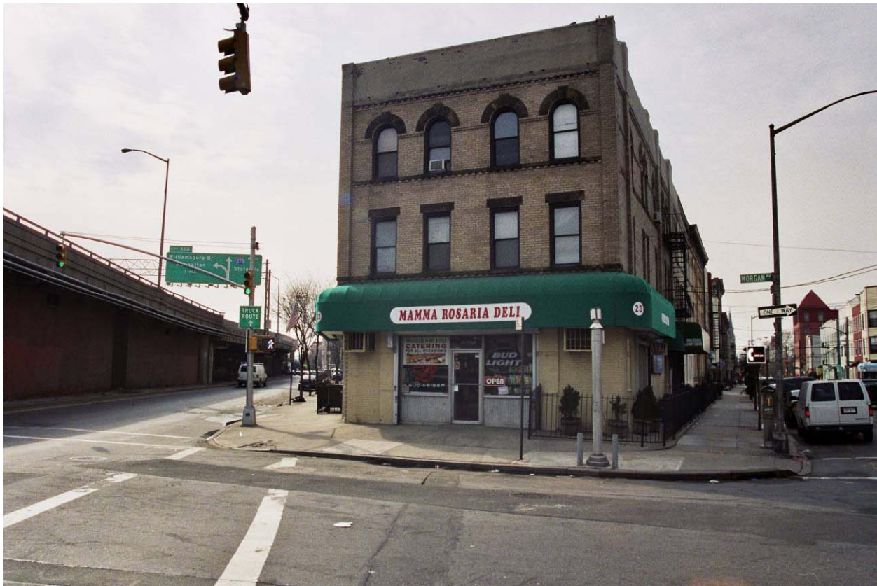
Photo V-40. 13-25 Driggs Avenue, Looking West
