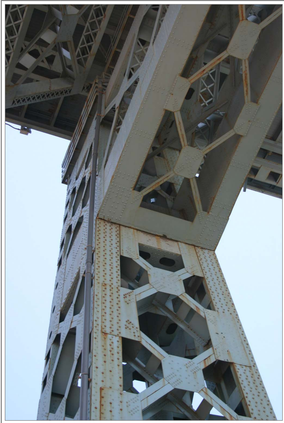
Photo V-20. Detail of truss connection beneath Kosciuszko Bridge
