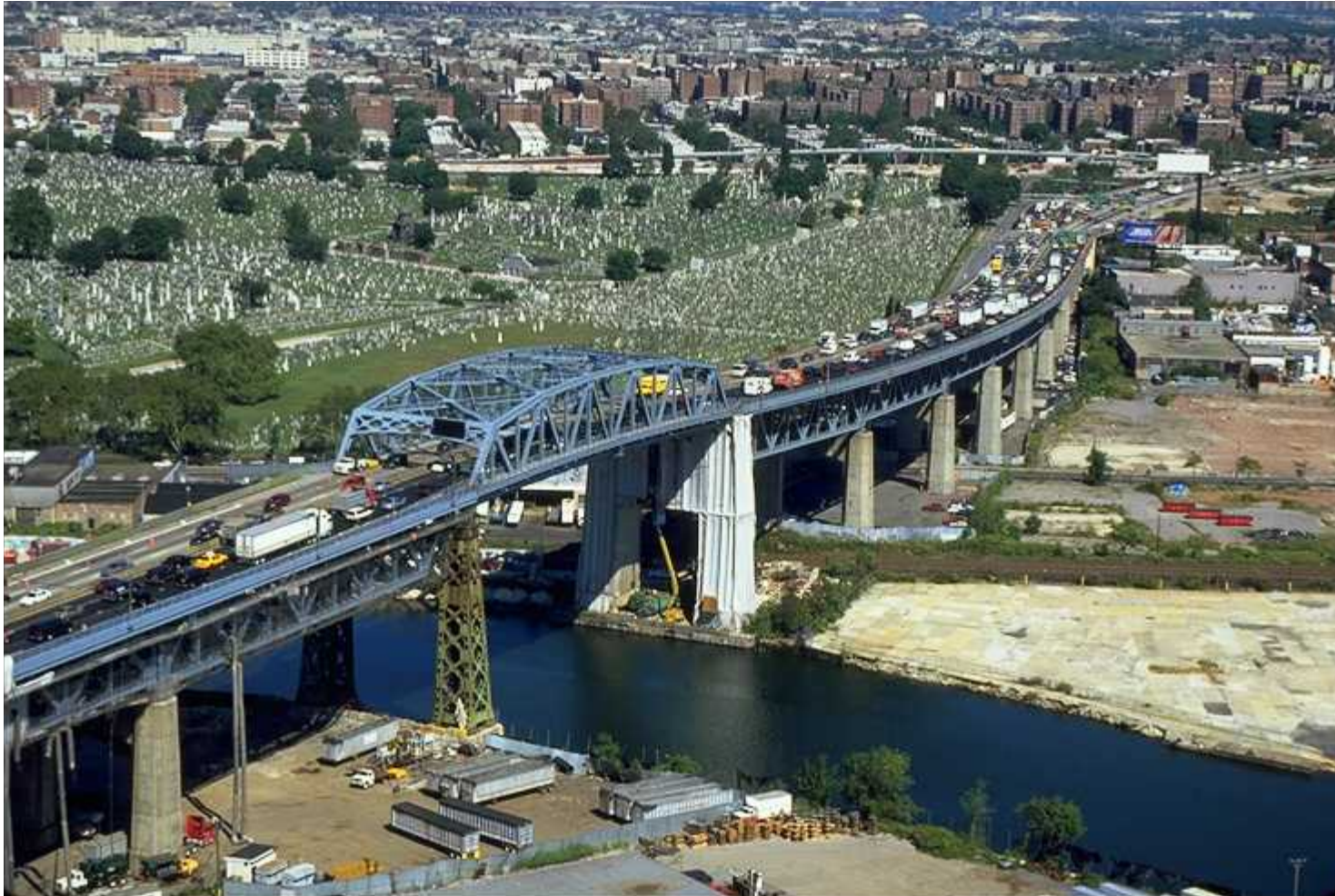
Figure IV-5: View of Main Span, Kosciuszko Bridge and Queens Approach, looking north (Calvary Cemetery and Sunnyside, Queens in background)
