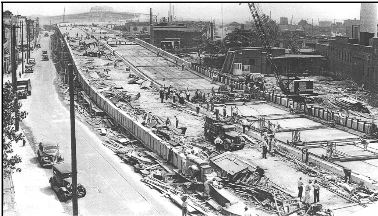
Image 7: Meeker Avenue Bridge Under Construction
