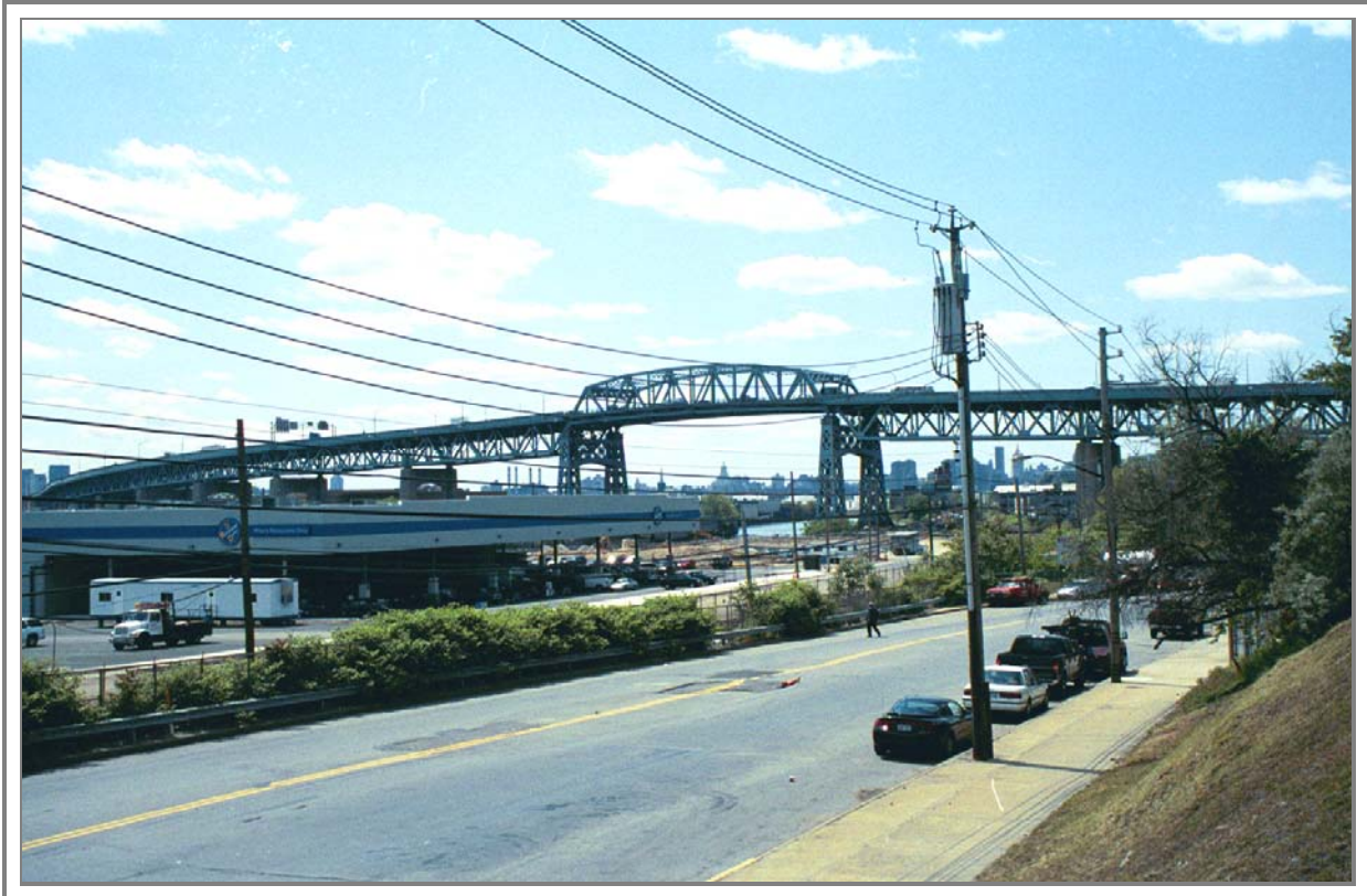
Photo V-14. Kosciuszko Bridge, looking west from 56th Road, Queens, New York
