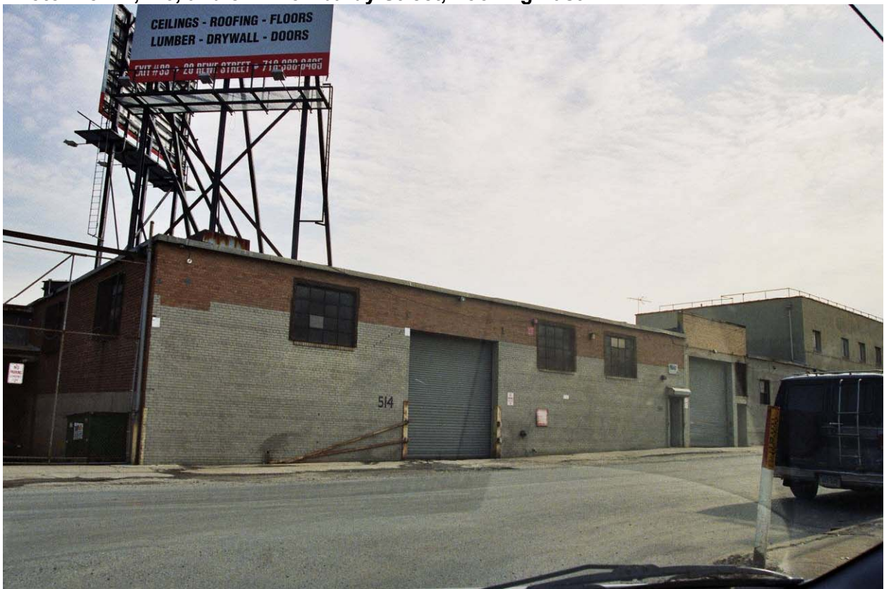
Photo V-52. 171-179 Lombardy Street, Looking Northwest
