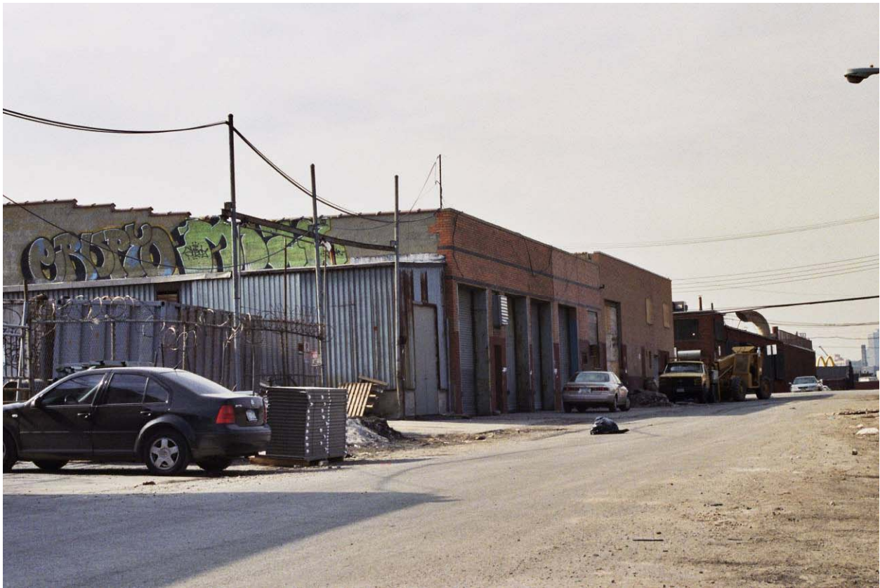
Photo V-59. 72 Anthony Street, Looking Southwest
