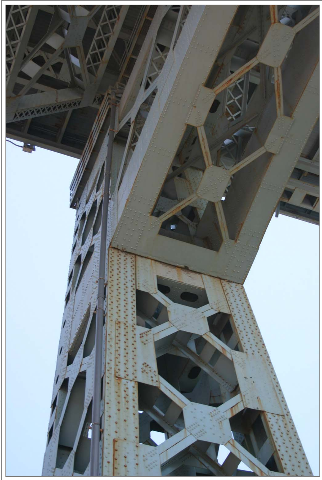
Detail of truss connection beneath Kosciuszko Bridge
