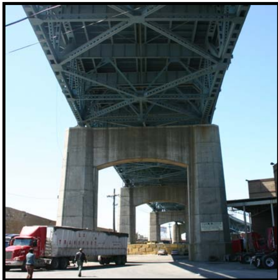
Image 1: Detail of bridge piers Image Courtesy of EHT Tracerics, May 2006
