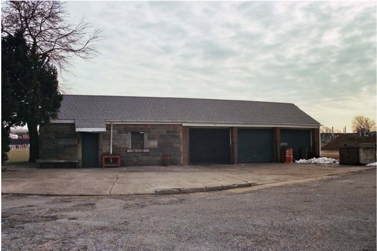
Photo V-8. Old Calvary Cemetery Equipment Shed, Looking Northeast
