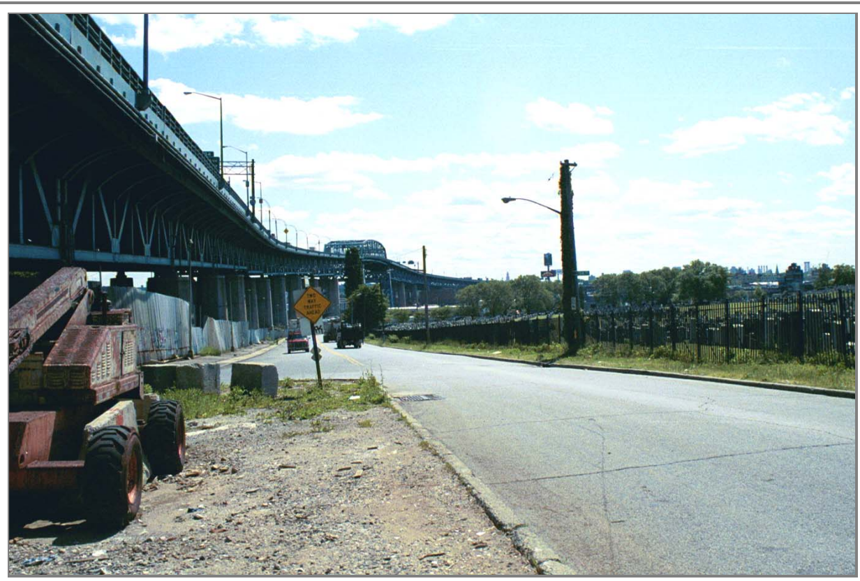
Photo V-13. Extent of Kosciuszko Bridge looking south from Laurel Hill Boulevard, Queens, New York
