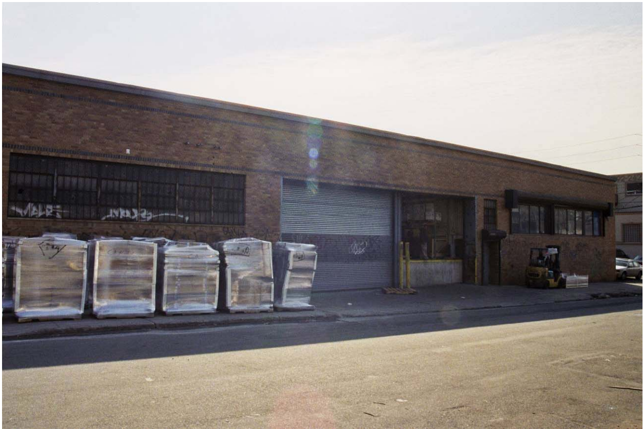
Photo V-91. 54-59 43rd Street, Looking Southeast
