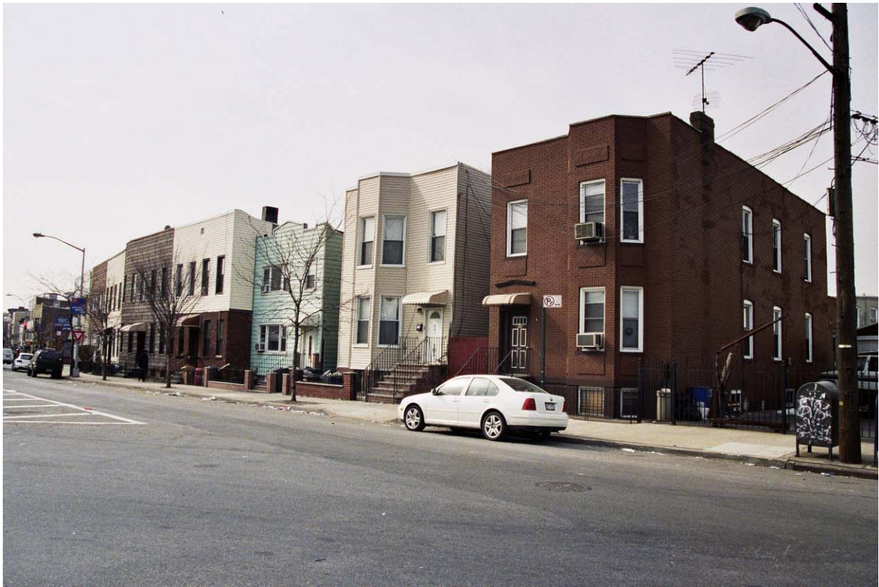
Photo V-32. 787-795 and 797-805 Meeker Avenue, Looking West
