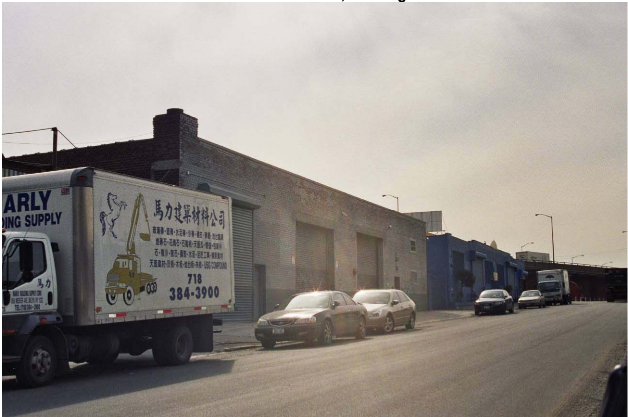
Photo V-33. 810-822 Meeker Avenue, Looking Southwest
