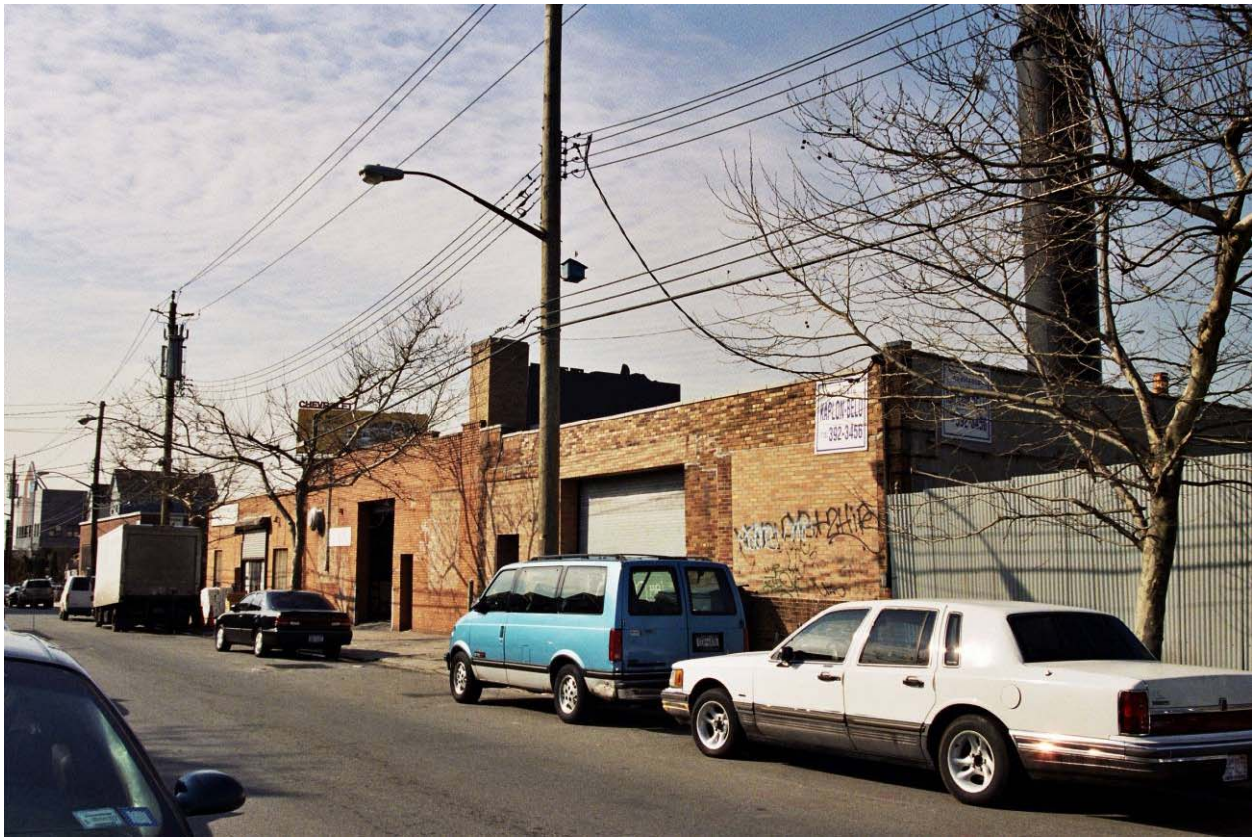
Photo V-95. 54-08, 54-14 and 54-18 43rd Street, Looking Southwest
