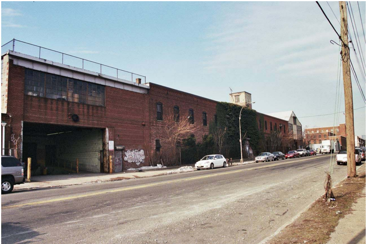
Photo V-81. 38-98 Review Avenue, Looking Southwest
