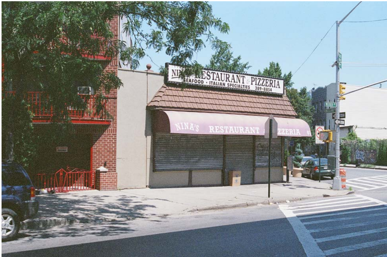
Photo V-45. 167-171 Kingsland Avenue, Looking North
