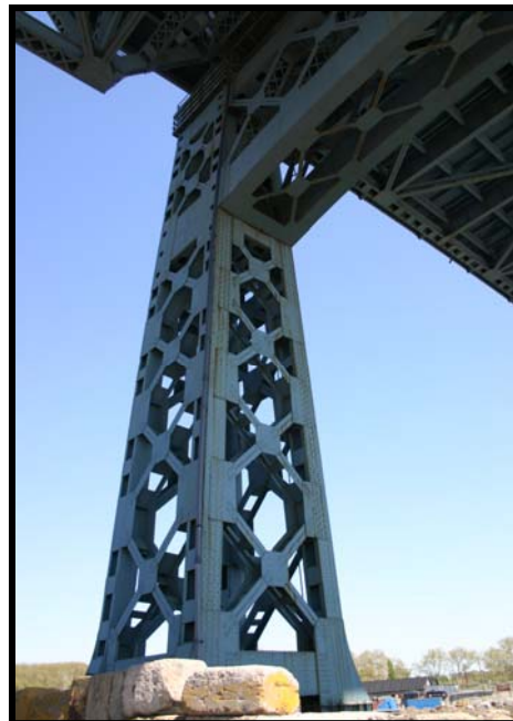
Image 2: Detail of main span piers Image courtesy of EHT Tracerics, May 2006
