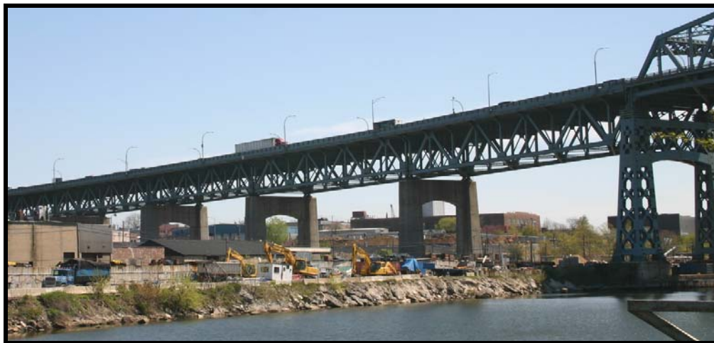
Image 24: Photo showing the multiple spans and deck truss of the Kosciuszko Bridge EHT Traceries, May 2006
