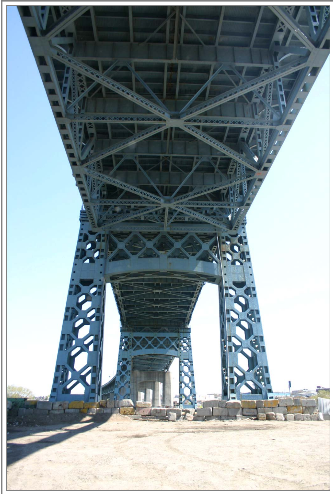
Detail of steel substructure looking southwest from Greenpoint, Brooklyn, New York
