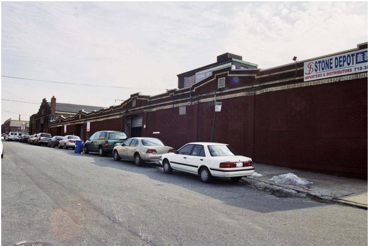
Photo V-53. 2-18 Anthony Street, Looking East
