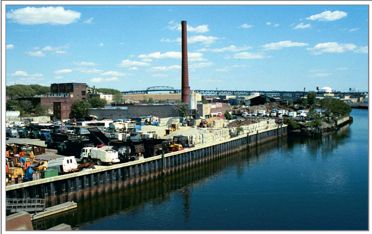
View of Kosciuszko Bridge, looking east from Greenpoint Avenue Bridge
