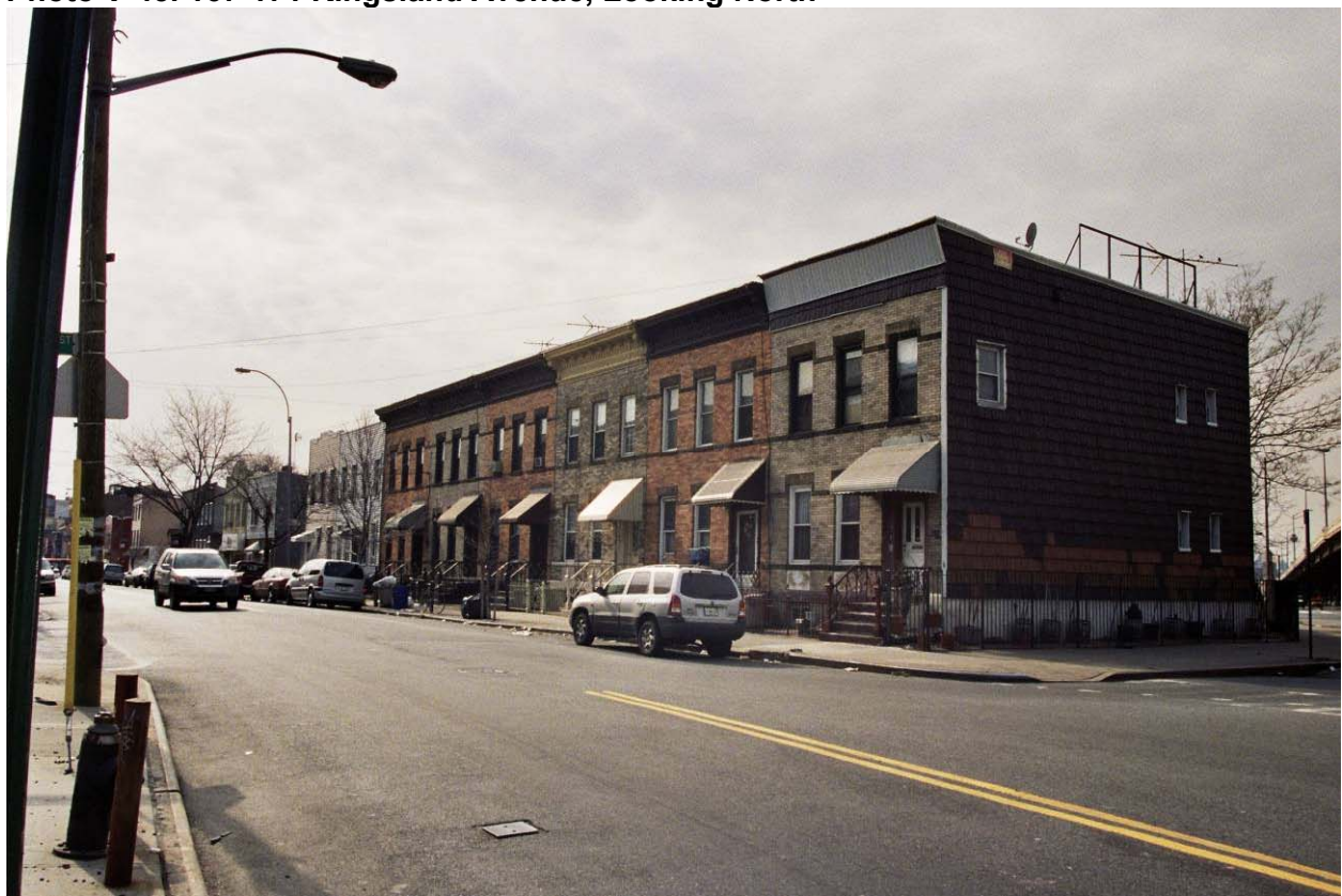
Photo V-46. 145-151 Kingsland Avenue, Looking South
