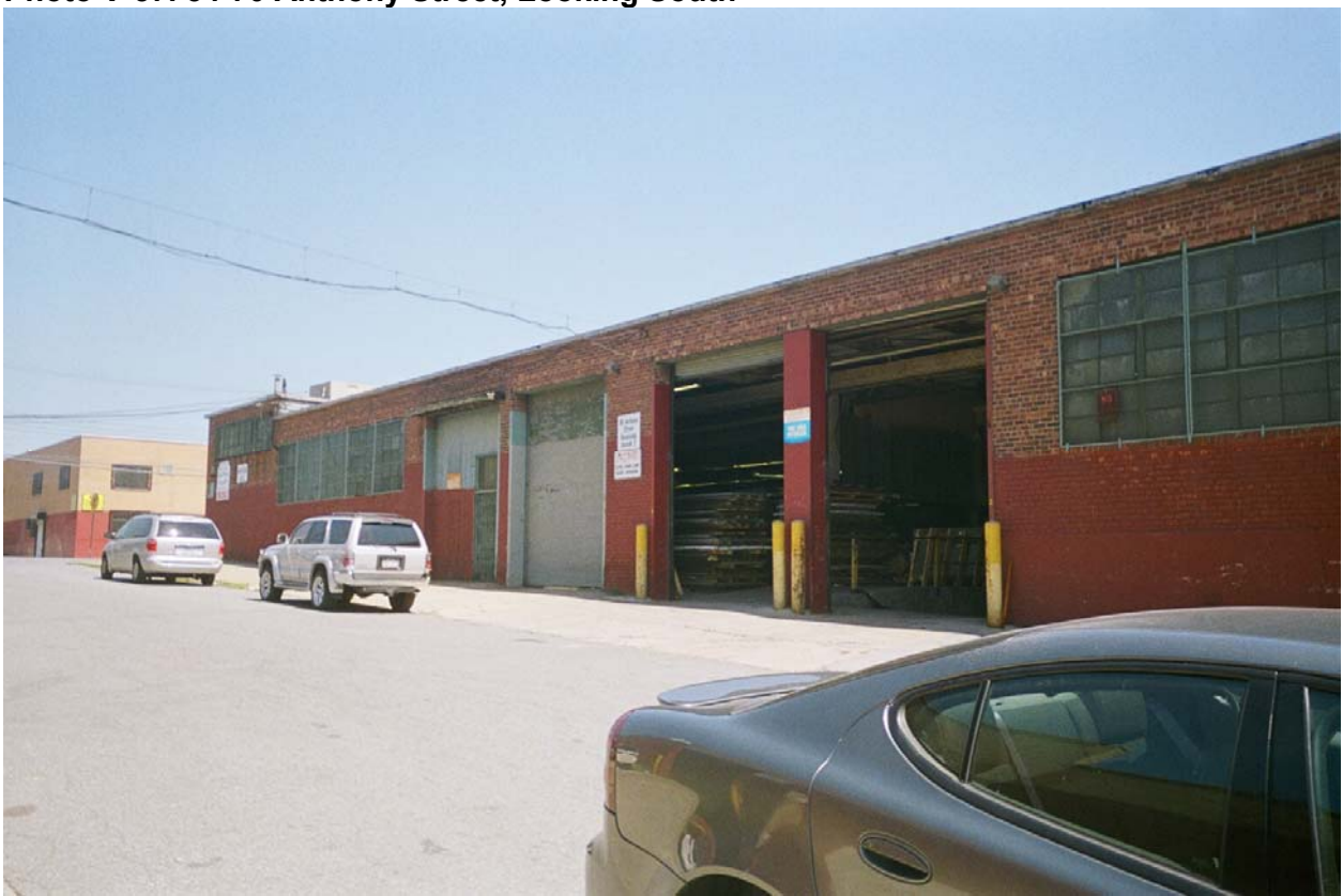
Photo V-58. 54-70 Anthony Street, Looking Southwest
