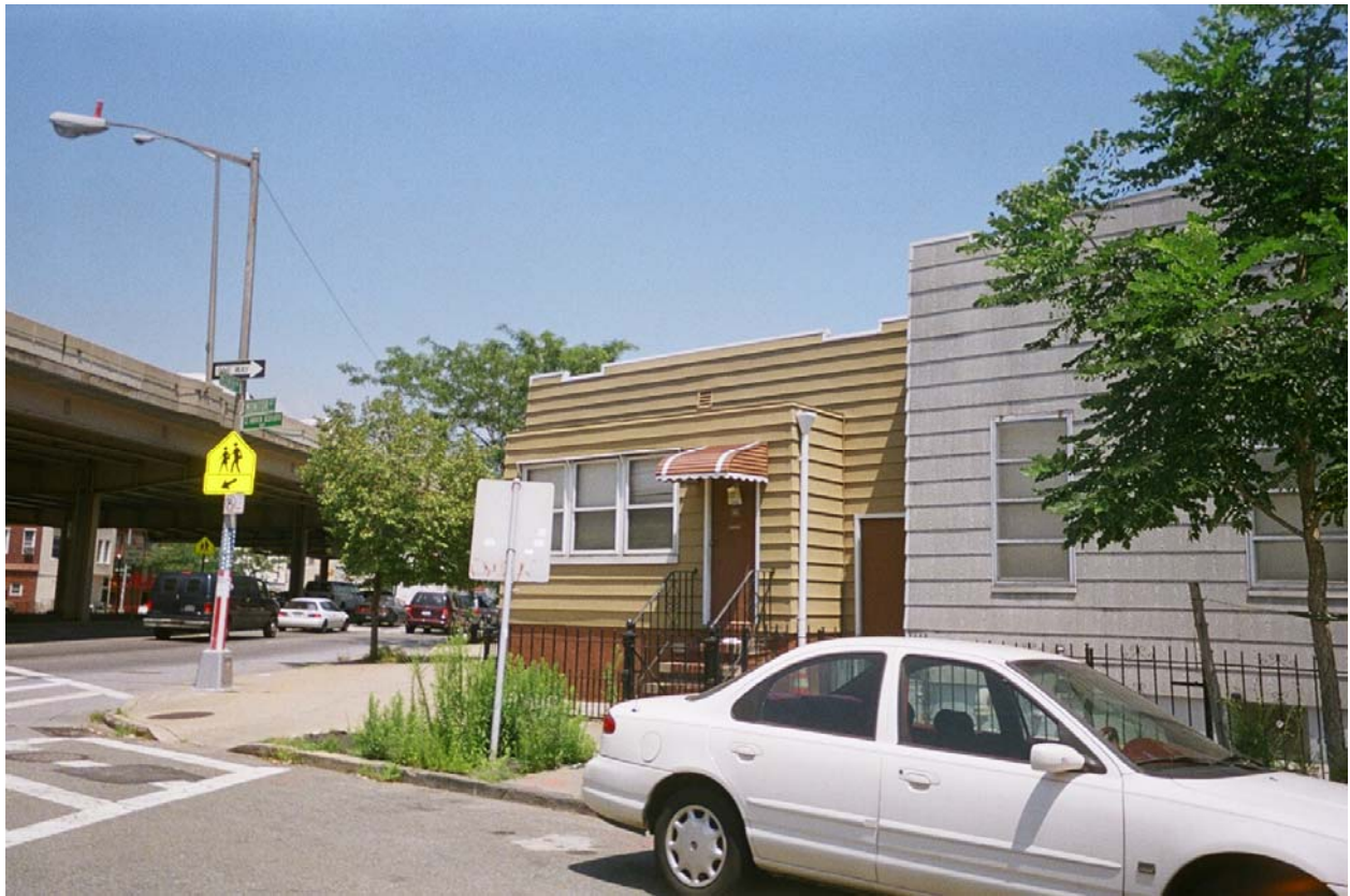
Photo V-24. 62 Monitor Street, Looking Northeast
