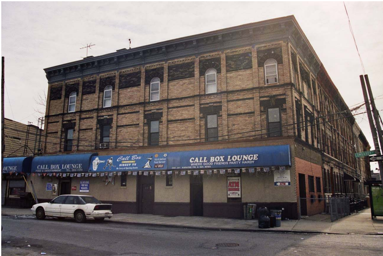
Photo V-47. 148 Kingsland Avenue, Looking South
