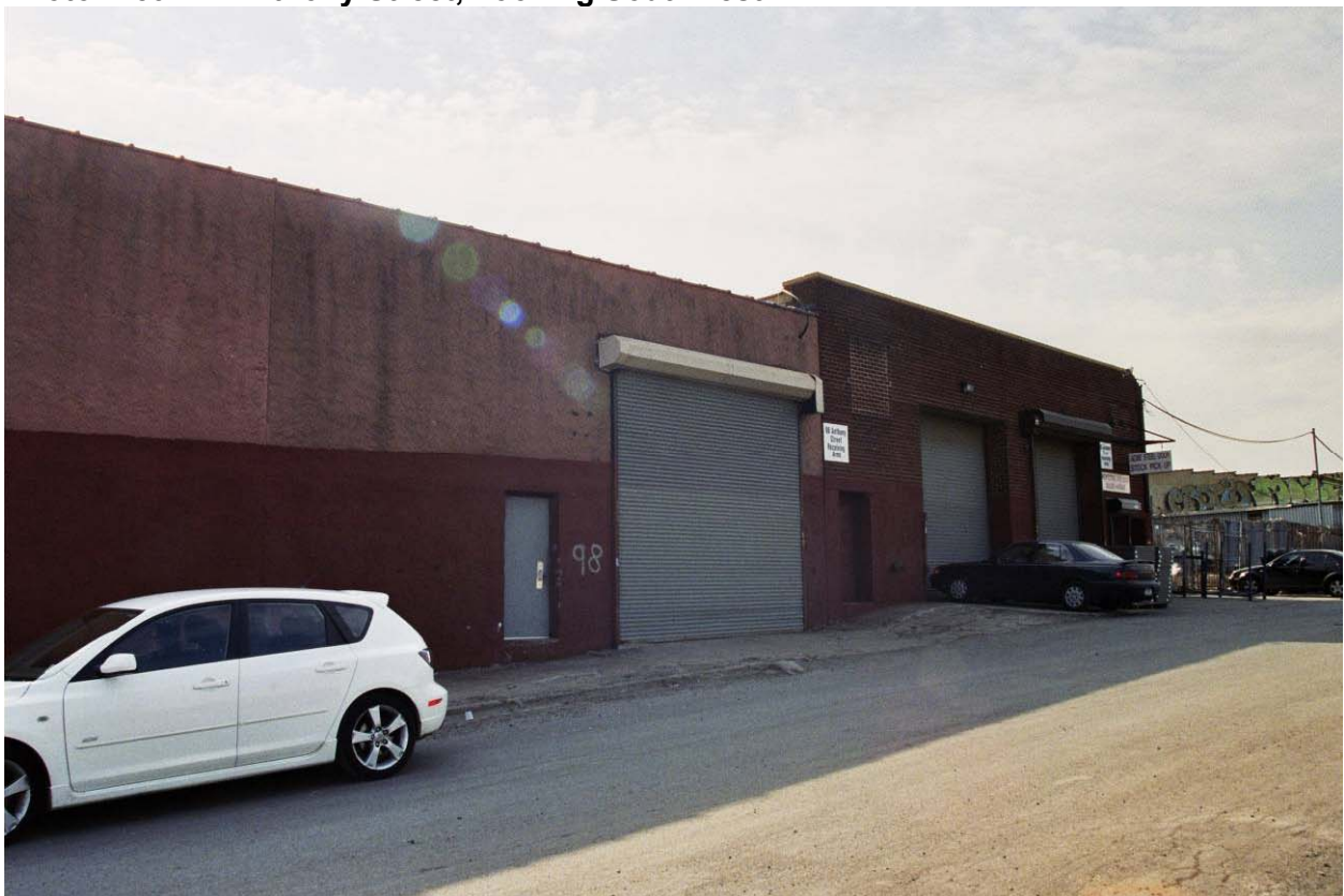
Photo V-60. 96-102 Anthony Street, Looking Southwest
