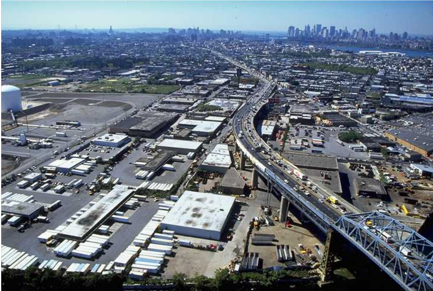
Figure IV-4: View of the Brooklyn Approach and the BQE, looking Southwest (Downtown Brooklyn and Lower Mahattan in background)
