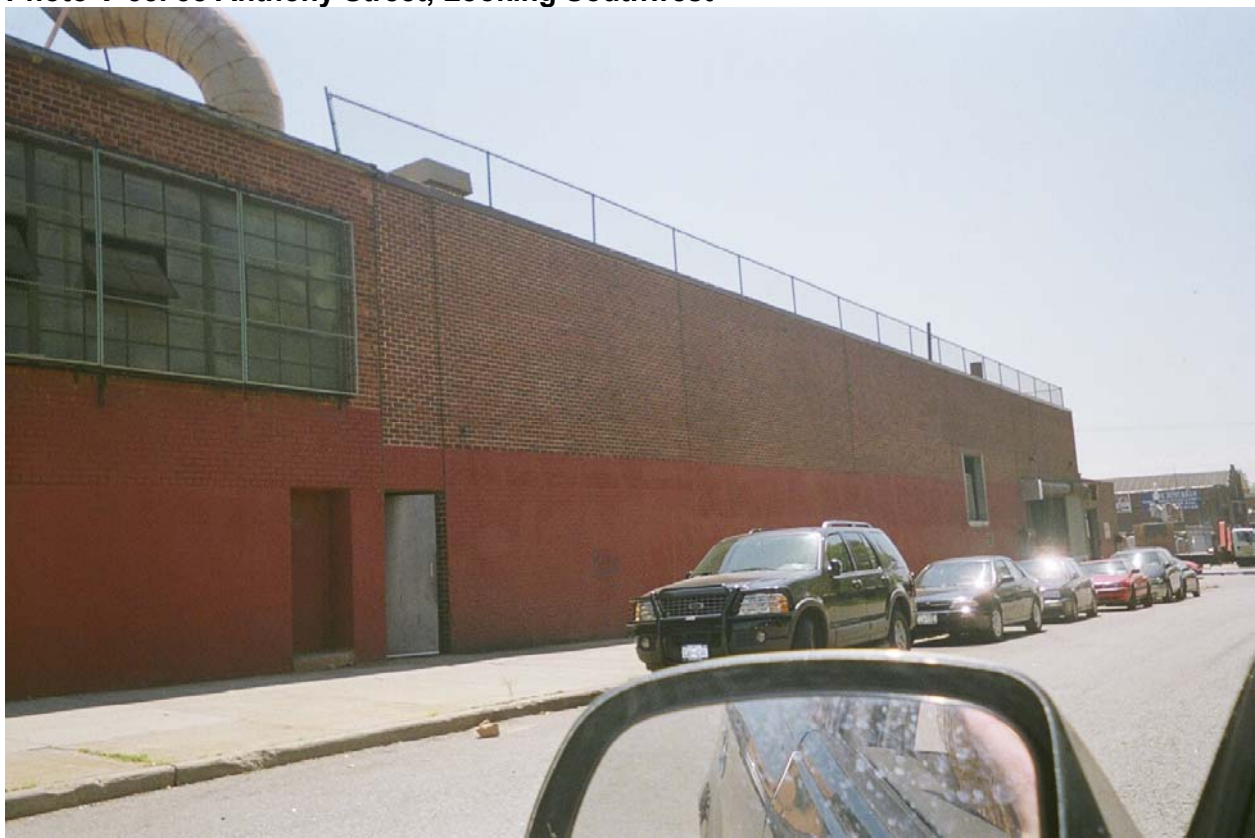
Photo V-56. 46-52 Anthony Street, Looking Southwest
