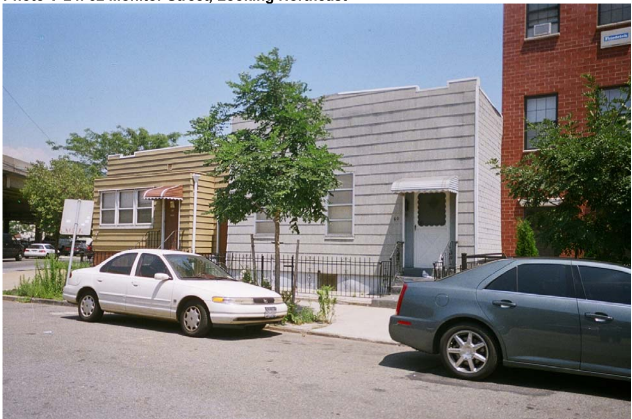
Photo V-25. 60 Monitor Street, Looking Northeast
