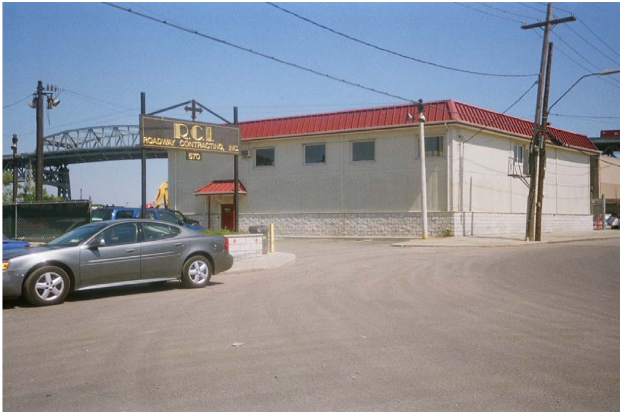
Photo V-75. 570 Gardner Avenue, Looking Southeast
