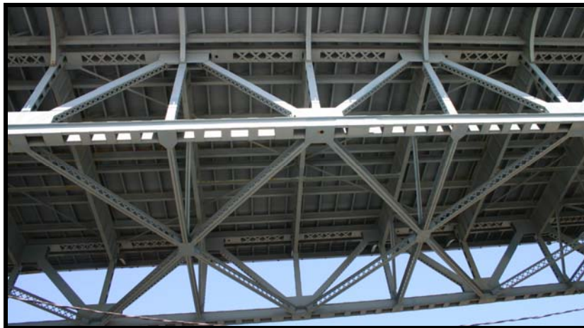
Image 4: Detail of Warren deck truss and I-beam grating, Image courtesy of EHT Tracerics, May 2006
