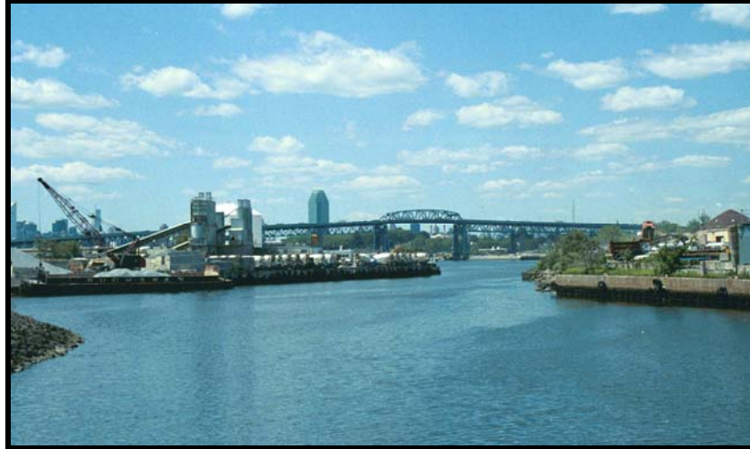
Image 11: Kosciuszko Bridge from the Grand Street Bridge, with a view of the Newtown Creek
