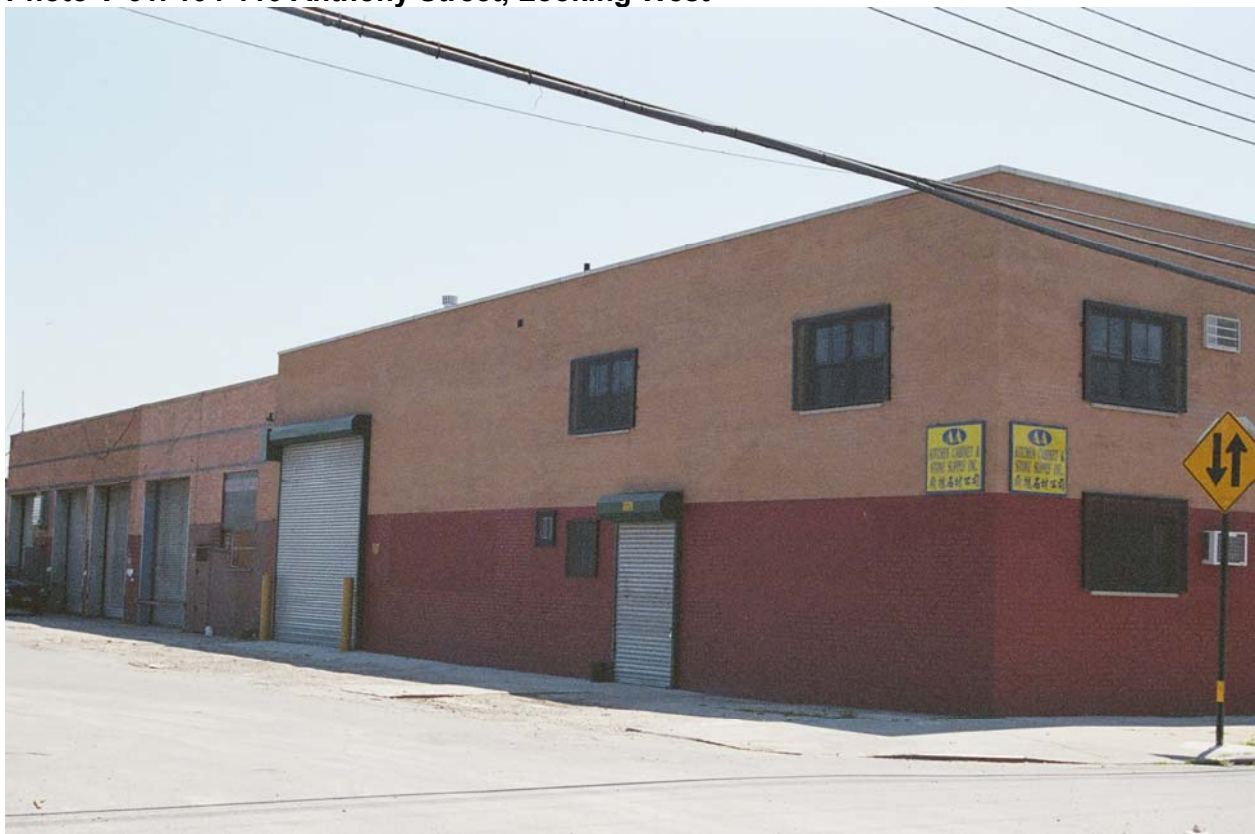
Photo V-62. 104-110 Anthony Street, Looking Southwest
