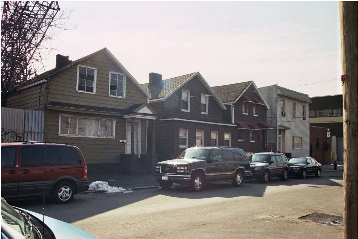
Photo V-93. 54-09, 54-11, 54-13, and 54-17 43rd Street, Looking Southeast
