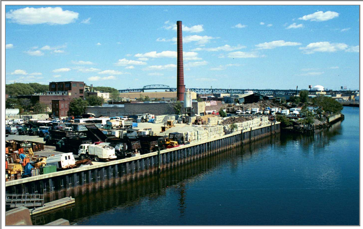
Photo V-12. View of Kosciuszko Bridge, looking east from Greenpoint Avenue Bridge
