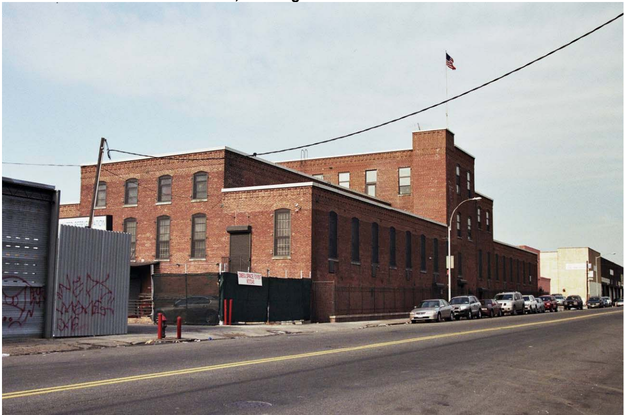
Photo V-82. 36-60 Review Avenue, Looking Northwest
