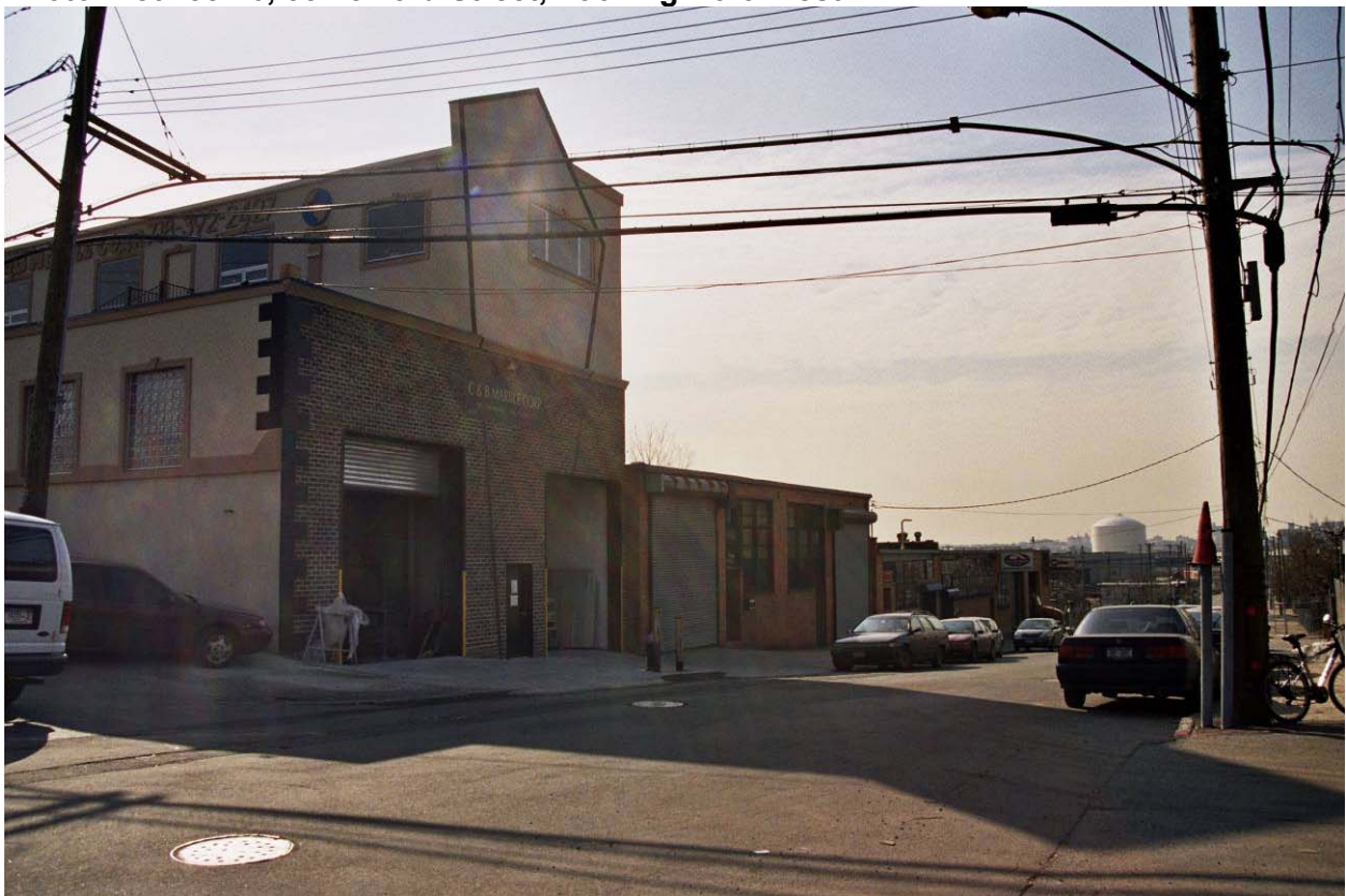
Photo V-90. 55-01 and 55-05 43rd Street, Looking Southeast
