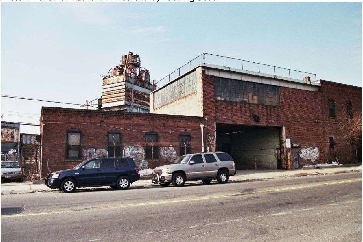
Photo V-80. 39-30 Review Avenue, Looking Southwest
