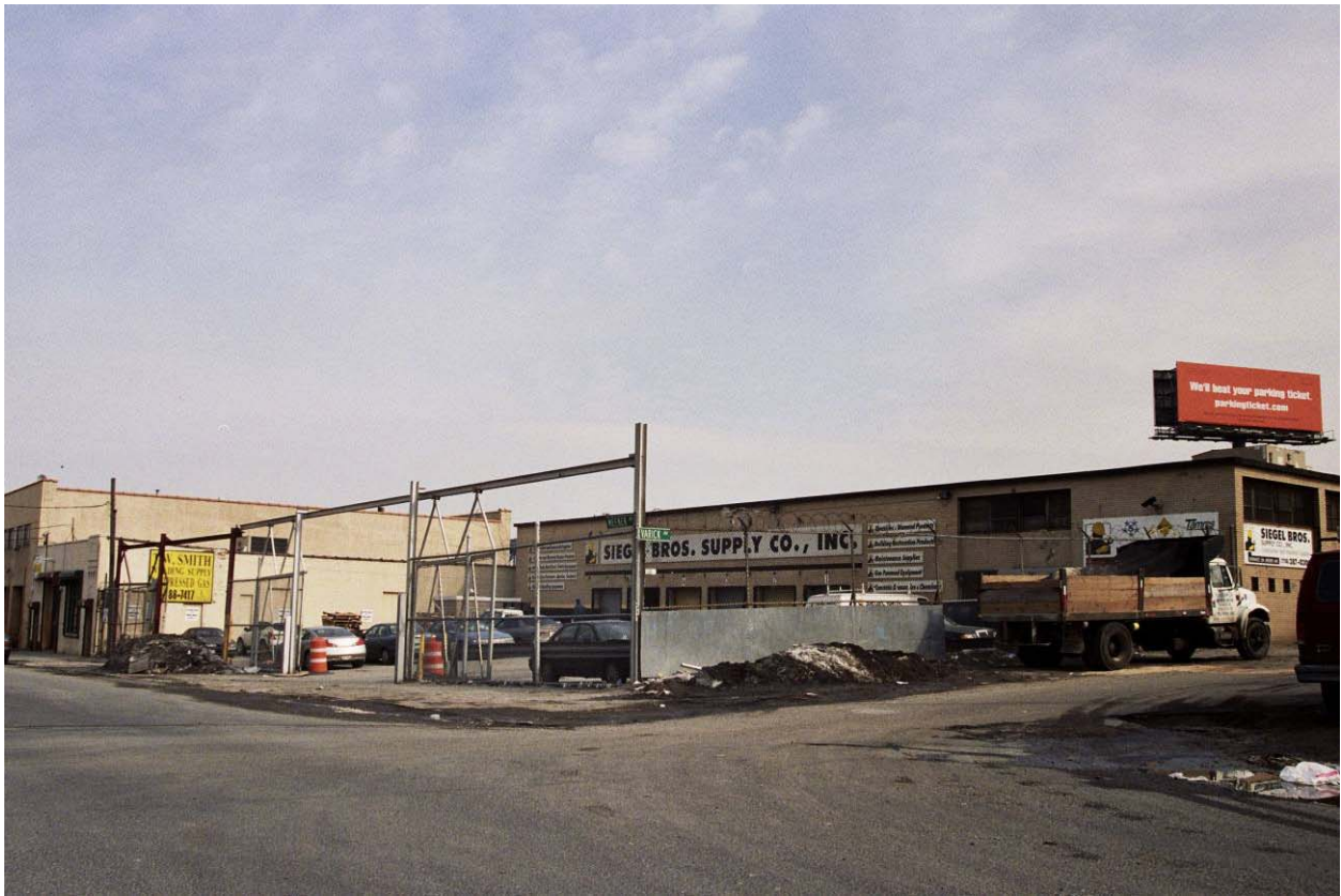
Photo V-36. 890-892 Meeker Avenue, Looking Southeast
