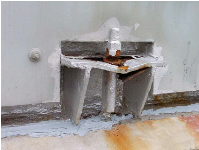
Figure 7.6: Kashiwazaki Port - Anchorage of asphalt storage tank (Located near Site RK25, N37.36713° E138.53210°, photo taken 7/22/07 12:37).
