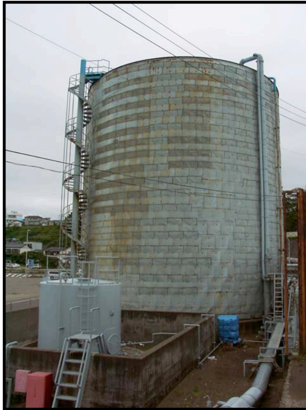
Figure 8.7: Kashiwazaki Port - Asphalt storage and transport facility located in the western portion of the port (Located near Site RK25, N37.36713° E138.53210°, photo taken 7/21/07 15:58).
