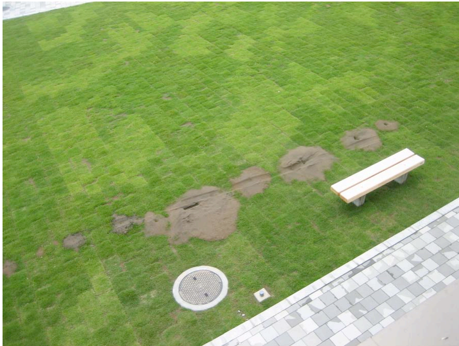
Figure 4.26: Kashiwazaki Harbor - South area exhibited surficial features of liquefaction on all sides of the port building. (Site RK25, N37.36713° E138.53210°, 7/20/2007).
