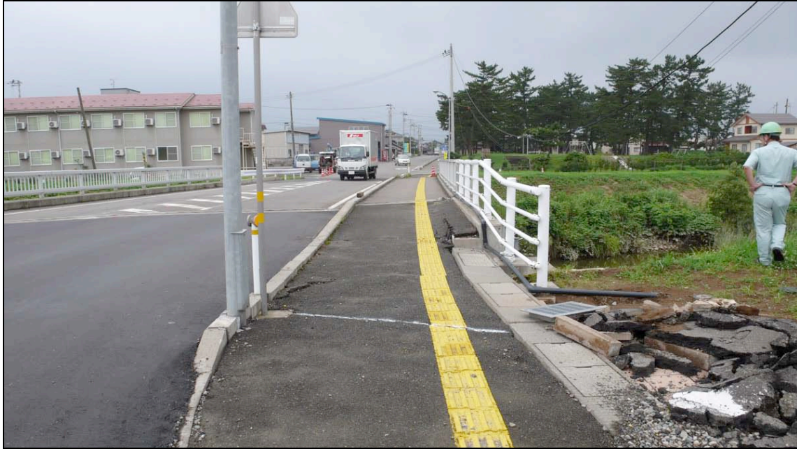
Fig. 6.33. Looking north from island at Hashi bridge deck.
