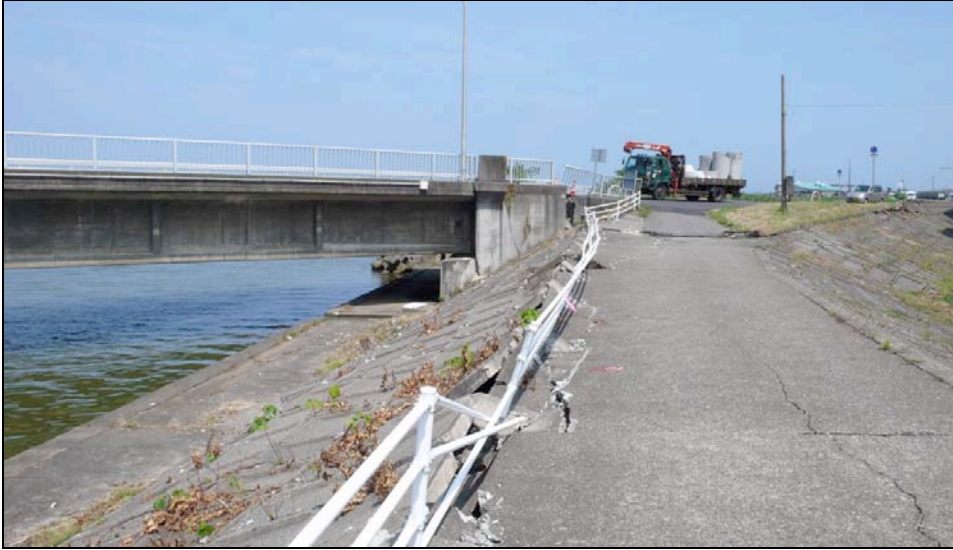
Fig 6.50. Rinko Yasaka Bridge at the mouth of the Ugawa.
