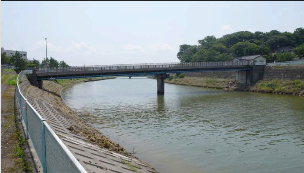
Fig. 6.59. Looking east (upstream) at the Osu Bashi.
