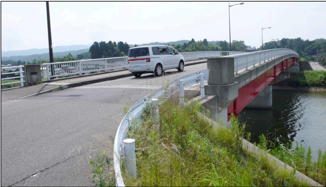
Fig. 6.66. Looking at the north approach.
