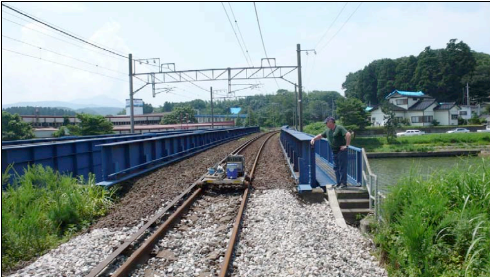
Fig. 6.64. Looking at rails on the west bridge where rail crew had left their tools.
