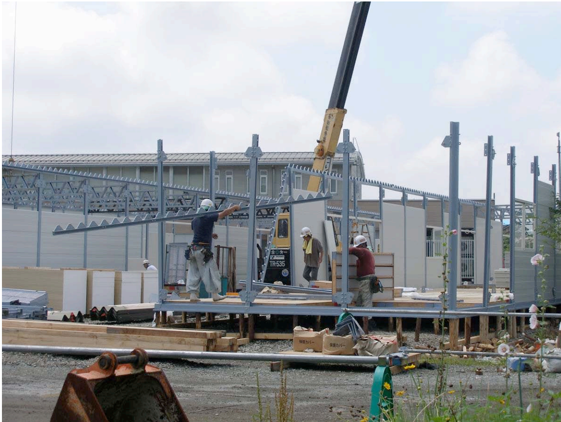
Figure 11.6: Construction of temporary housing underway in the Kashiwazaki area, July 27.
