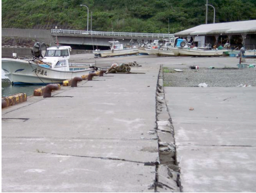
Figure 8.2: Kasashima Harbor - Ground settlement and minor lateral deformation adjacent to quay walls (Site RK21, N37.33702° E138.46680°, photo taken 7/21/07 14:40).
