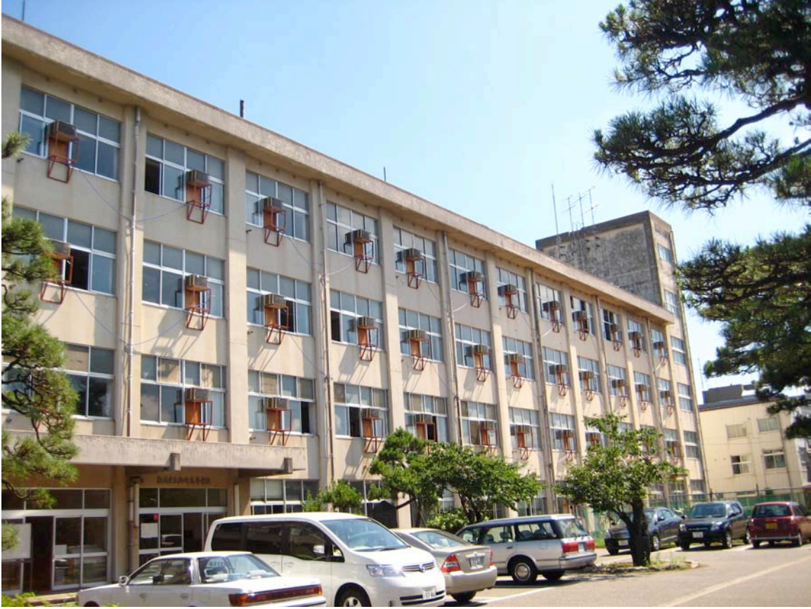
Figure 5.16: Kashiwazaki High School, south building (Site SP11, N37.3721° E138.5569°).
