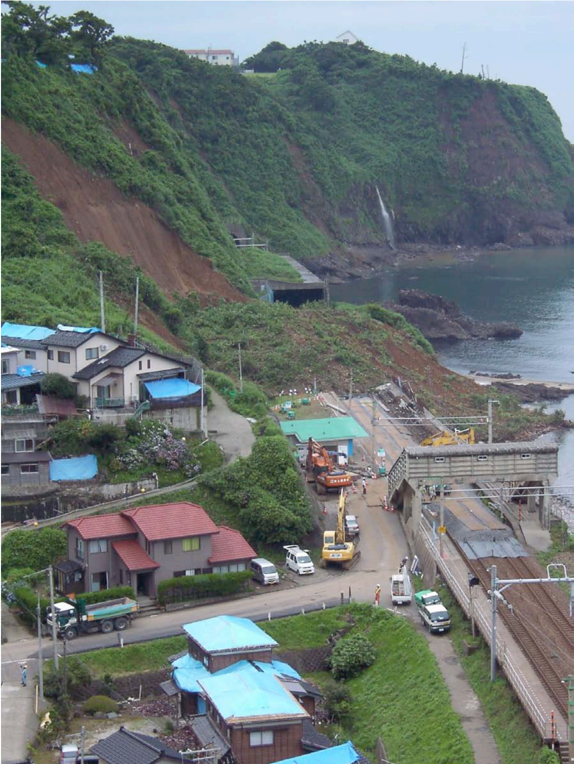
Figure 9.10: Landslide at Oumigawa Train Station impacted Shin-etsu line railway (Sites RK20/YT16/SA9, N37.34490° E138.48435°, 7/21/07 13:52).
