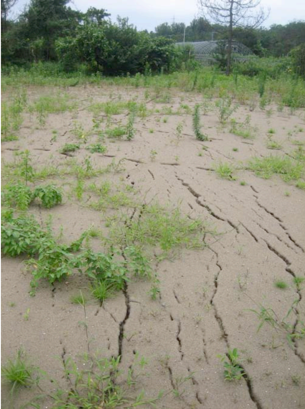
Figure 4.34: Lateral spreading in dune sand down slope of high voltage power transmission tower. We measured 0.6% of ground strain at the site. (Site RK40, N37.41633° E138.60792°, 7/22/2007).
