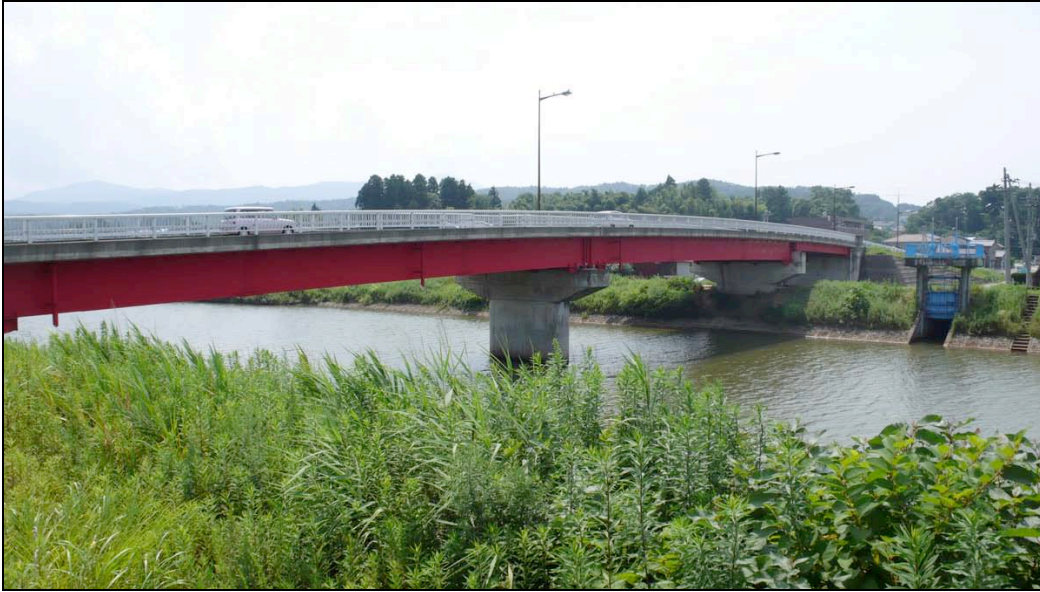
Fig. 6.65 View looking south across the Ugawa River at this steel bridge.
