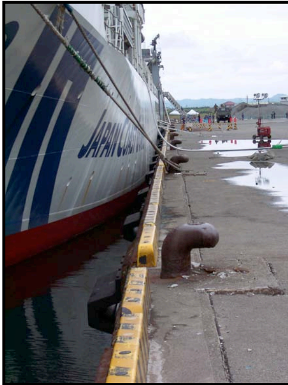
Figure 8.23: Kashiwazaki Port - Evidence of very minor lateral movement of quay walls and minor settlement located along the northern face of the terminal used as the berth for the Japan Coast Guard (Site SD8, N37.36680° E138.53825°, photo taken 7/22/07 15:22).
