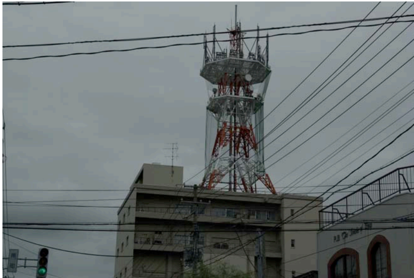
Figure 10.8: NTT communications building in downtown Kashiwazaki (Site SD20, N37.36847° E138.55813°, photo taken 7/23/07). No evidence of major structural damage to the tower was observed however no information on the performance of the electronics was available at the time of the investigation.
