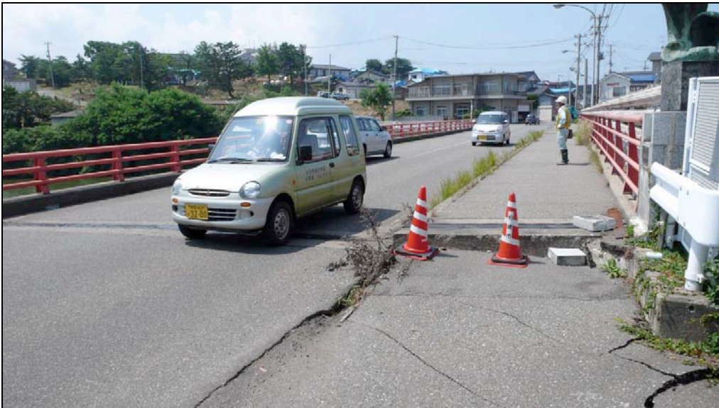
Fig. 6.56. Approach and deck of Yasaka Bridge.
