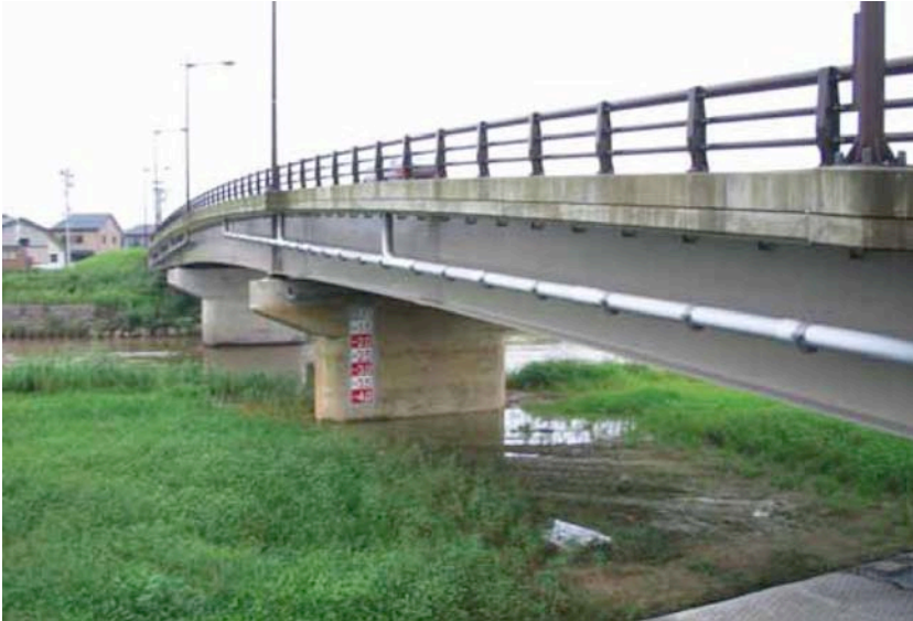
Fig.44. Nagomi Bridge (photo courtesy of Scott Brandenburg).
