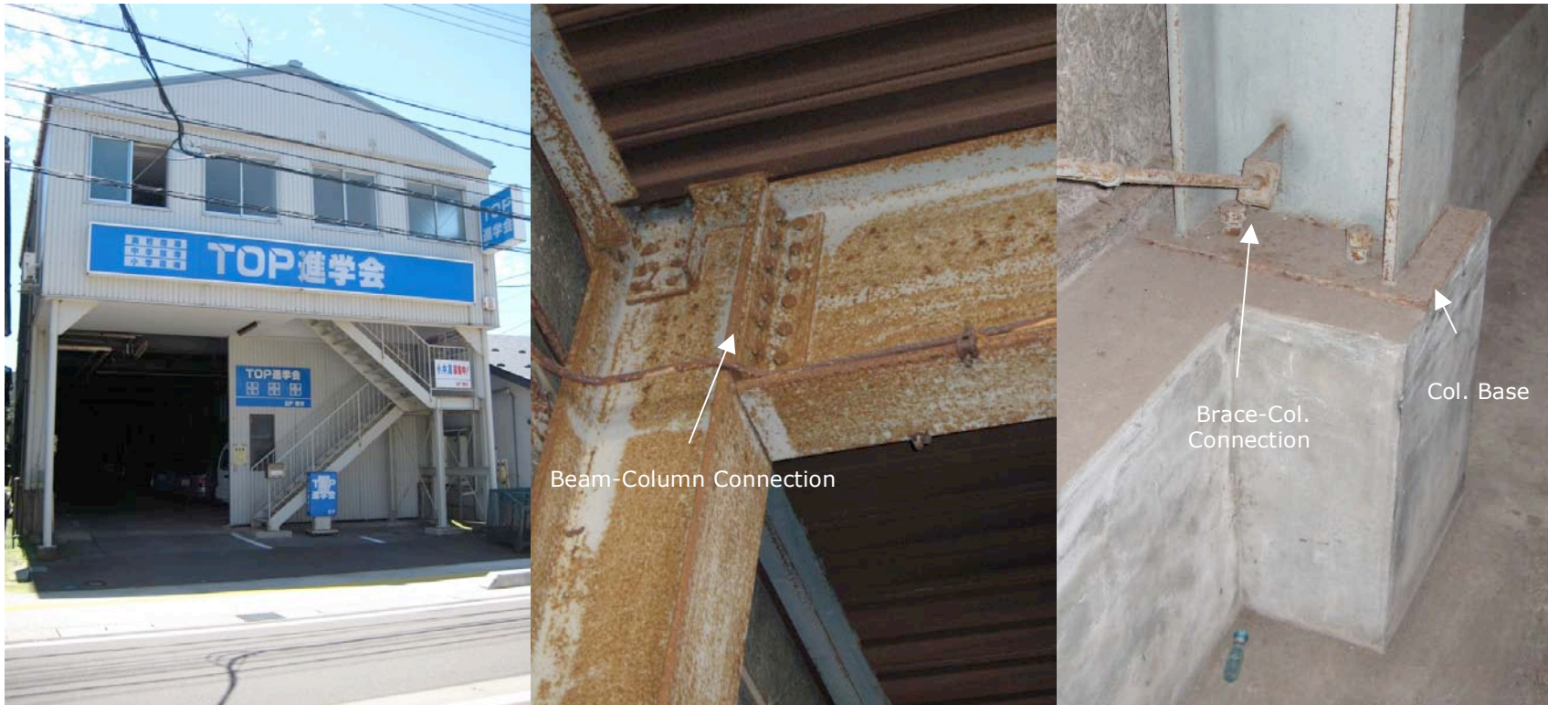
Figure 5.13: Parking structure in Kashiwazaki (Site SP29, N37.3707° E138.5566°).
