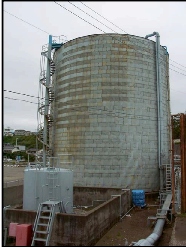
Figure 7.5: Kashiwazaki Port - Asphalt storage and transport facility located in the western portion of the port (Located near Site RK25, N37.36713° E138.53210°, photo taken 7/21/07 15:58).
