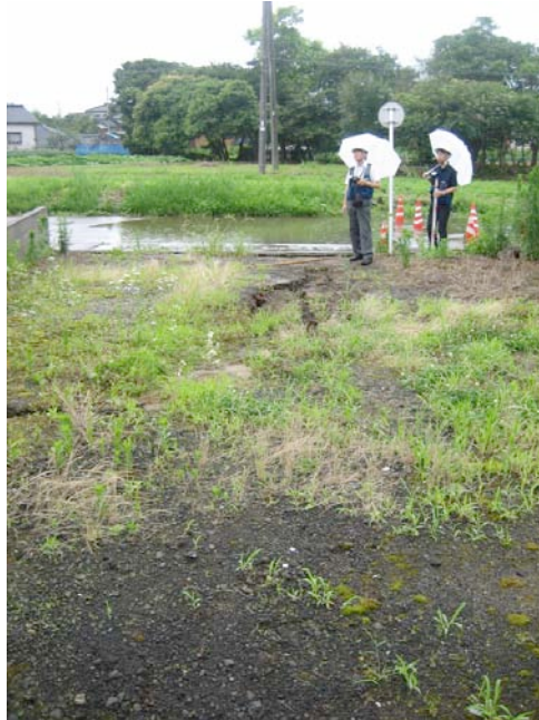
Figure 4.8: Kai-Un Bridge area Sabaishi River (Site RK4 N37.39233° E138.58063°, 7/19/2007, 1:40 p.m.). A sub-linear zone of lateral spreading, sand boils and settlement that may be associated with a buried shoestring sand deposit from the former channel of the Sabaishi River resulted in damage in the neighborhood immediately south of the Kai-Un Bridge.
