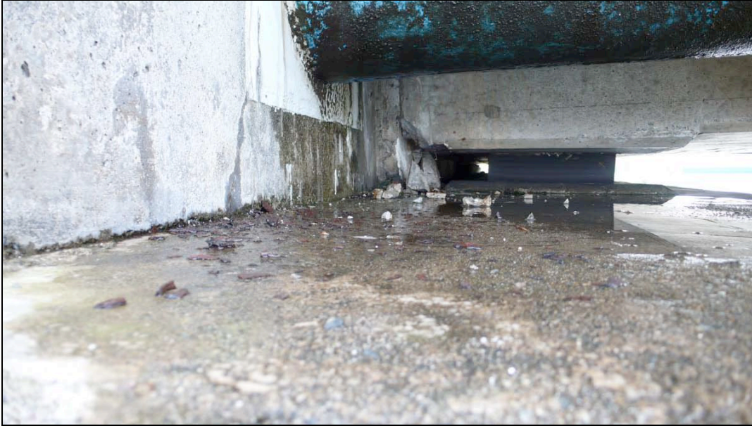
Fig. 6.61. The superstructure is supported on a single bearing (note waterline).
