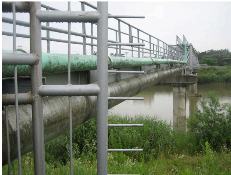
Figure 4.3: Kai-Un Bridge over Sabaishi River (Site RK4 N37.39233°,E 138.58063°, 7/19/2007, 1:40 p.m.). A water pipeline rupture was found with pipe offsets of 13 cm in the horizontal direction, 10 cm in the vertical direction, and with 40 cm of associated nearby settlement between the pipeline and the ground.
