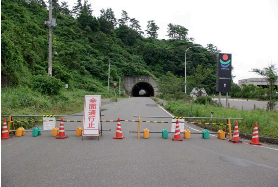
Figure 9.8: Tunnel was initially open to traffic following earthquake, but subsequently closed as of July 22 nd (Site SD4, N37.38439° E138.60083°, photo taken 7/22/07 13:36). Damage to tunnel was not observed, but landsliding and toppled monuments on top of the tunnel was observed.
