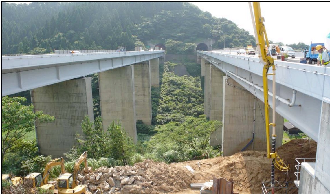
Fig. 6.2. Looking south at the Hachisaki Bridges.
