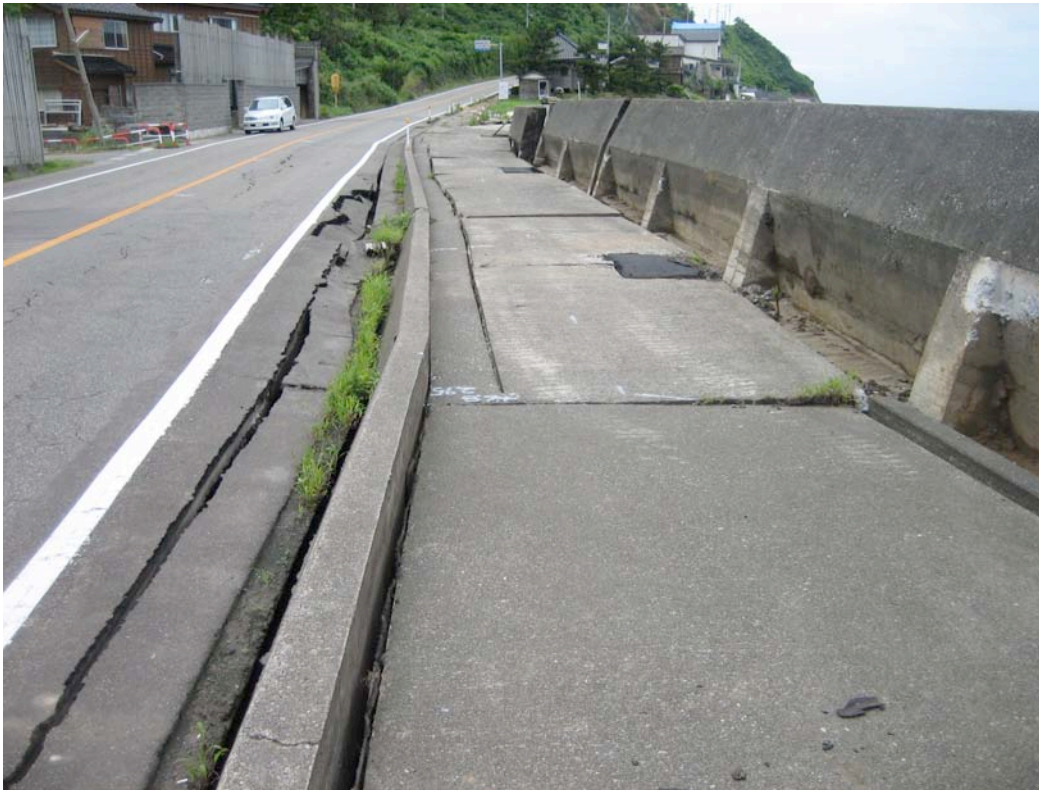
Figure 4.27: Liquefaction of beach sand led to lateral spreading of a road embankment and both rotation and translation of a 30-meter-long segment of concrete seawall. (Site RK35, N37.48497° E138.62645°, 7/22/2007).
