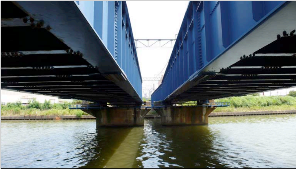
Fig. 6.63. Looking under the Railway Bridges.
