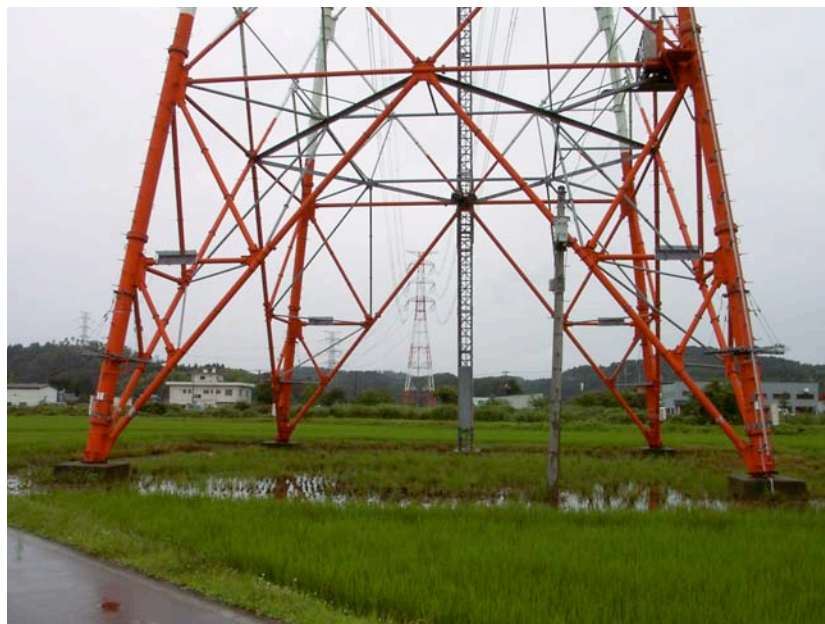
Figure 10.6: High voltage power line towers located in the Kashiwazaki area (Site RK12, N37.44113° E138.63390°, photo taken 7/21/07). No evidence of structural damage to the towers was observed.
