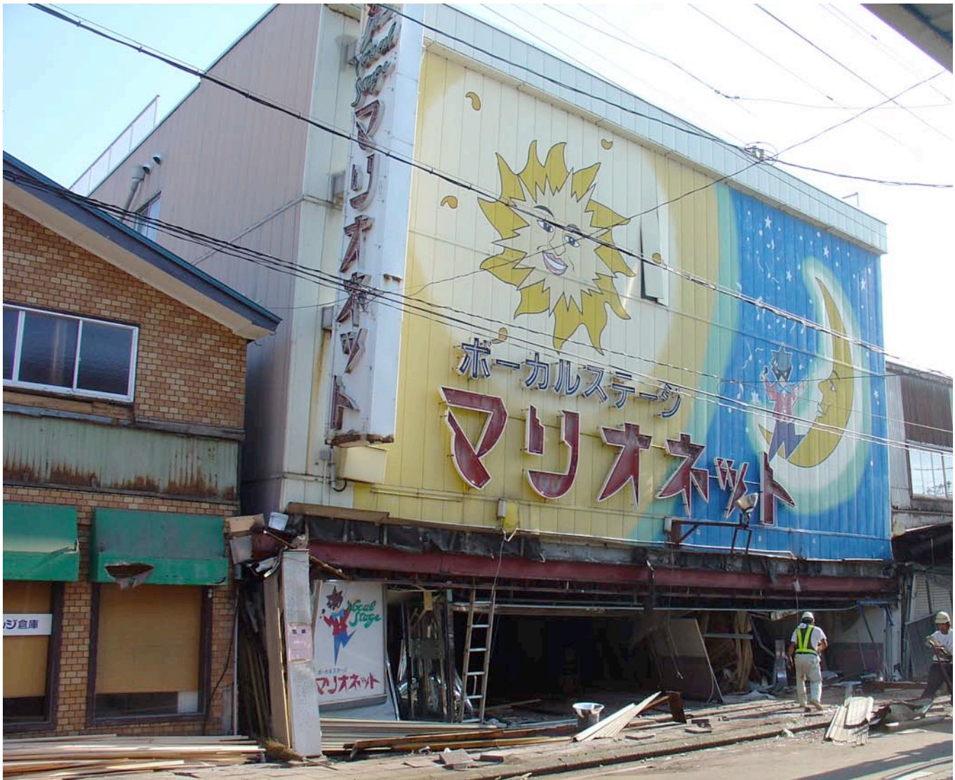
Figure 5.23: Karaoke parlor (Site NIT-81, N37.37000° E138.55825°, photo by Peter Yanev)
