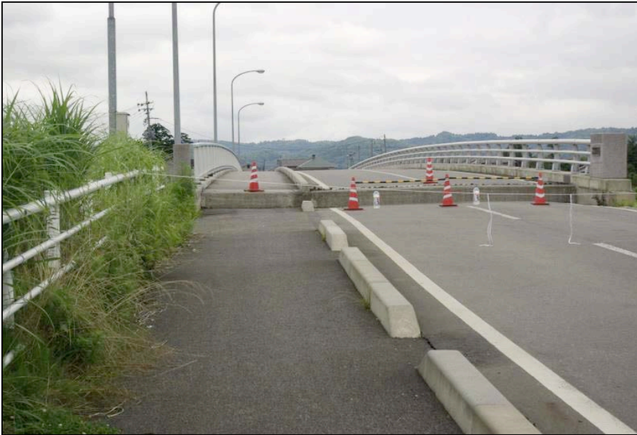
Fig 6.48 Genji Bridge (photo courtesy of Scott Brandenburg).
