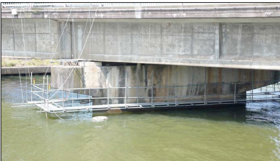
Fig. 6.54. Pier supporting Rinko Yasaka Bridge.
