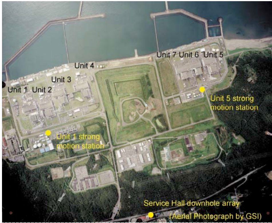
Fig. 2.10: Aerial Photograph of Kashiwazaki-Kariwa Nuclear Power Plan Area (GSI, 2007)
