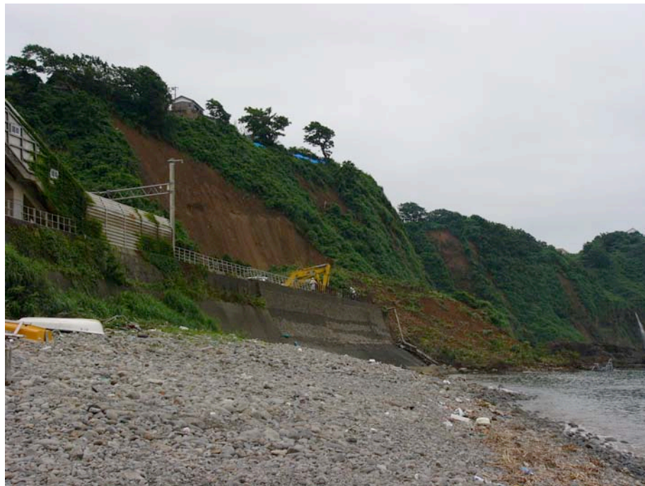
Figure 3.5: Landslide at the Oumigawa Train Station on the Shin-etsu Line (Site RK20/SA9/YT16; N37.34200° E138.48888°, photos taken 7/21/07 12:48 (top) and 7/24/07 15:00 (bottom)). This was among the larger of the coastal landslides to the south of Kashiwazaki. Site access was not possible due to construction repairs. Note that slope stability in this area has been a problem, as seen by the railway tunnel protection structure immediately behind (to the south) of this landslide. Many more smaller landslides were observed to the north and south of this location.
