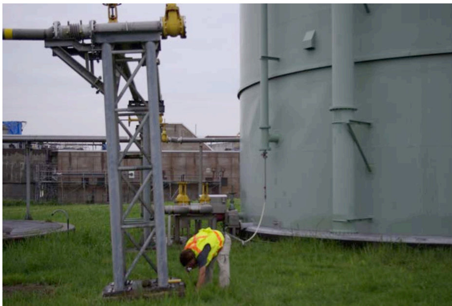
Figure 7.2: Steel tank at the Ansei-Chou waste water treatment plant (Site RK9, N37.38748°, E138.56587°, photo taken 7/20/07 16:40). Minor distress to the wall was observed roughly 3 m above the base of the tank.
