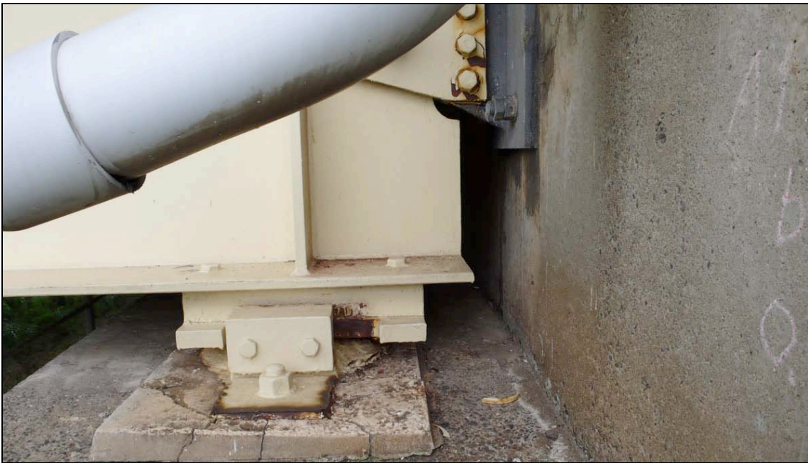
Fig. 6.9. Bearing at south abutment of Yoshiigawa Bridges.
