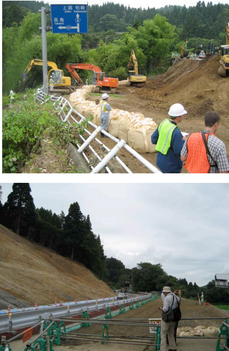
Figure 9.1: The Ozumi Senbon Landslide (Site RK1, N37.41422° E138.71347°), located along Highway 8 just north of the intersection with Route 252, closed both lanes of traffic. The upper photo, taken 7/20/07 at 11:30, four days after the earthquake, shows the displaced roadway which ran from the distance vehicles to the upper right of the photo to just in front of the investigation team members in the lower right. The bottom photo, taken 7/23/07 at 13:00, shows the nearly completed landslide and roadway repair, complete with guard rails, pavement, and center striping, just three days later.
