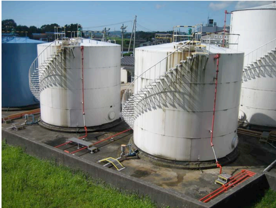
Figure 10.10: Oil storage and distribution facility (Site RK55, N37.38917° E138.63377°, photos taken 7/23/07 12:30). No damage was observed at this site.
