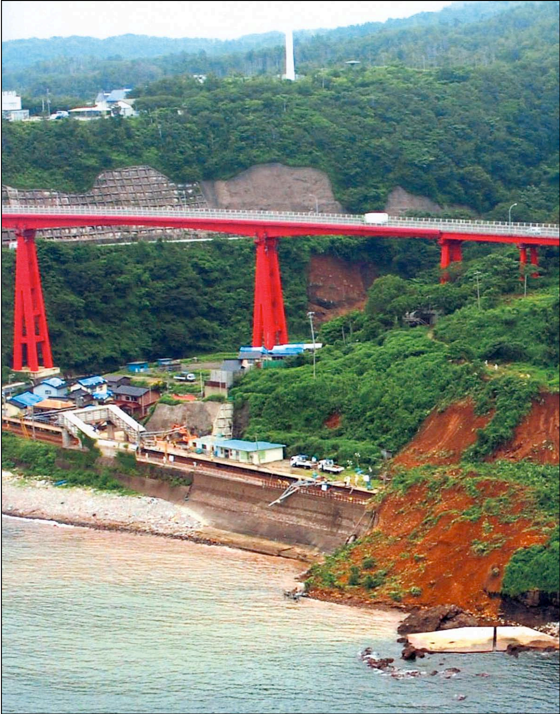
Fig. 6.21. Yoneyama Bridge and landslide.
