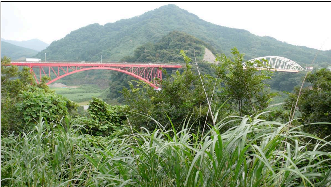
Fig. 6.28. Undamaged Agewa (Deck Arch) Bridge just north of damaged Yonahime Bridge.
