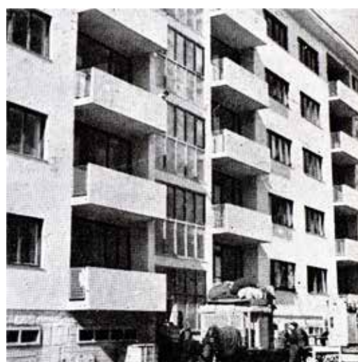
Fig. 1.: The settling in of one of the workers' families into the one of yet unfinished four CHBs (7s, 4aps) in the first "collective estate" in Zagreb after the WWII, 1947? The main transport vehicle is the horse carriage. 5-8 resp. Gaje Alage St, Frana Bošnjakovića St, Ivana Stožira St, Fausta Vrančića St. Arch.: Vladimir Potočnjak, Zlatko Neumann, Stjepan Gomboš, Mladen Kauzlaric (Source: [2], p. 25)
