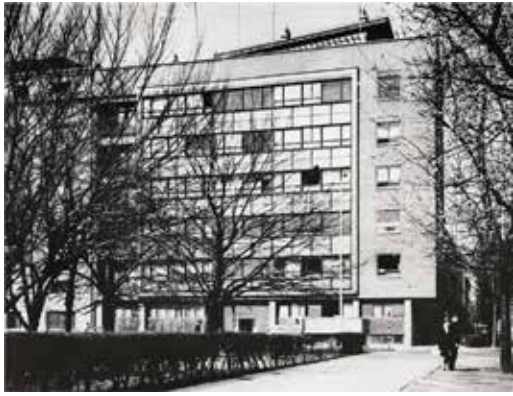
Fig. 12.: 3Aps corner attached apartment building, a convincing method of extrapolating meshes and frames in historicist environment of the time between 1890 and 1918. 7s CHB, 14 King Peter Svačić Sq. Arch.: Prof. Drago Galić, 1953 (Source: [17], p. 142)
