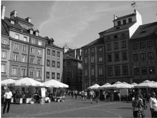
Fig. 1.: Warsaw. Old town market. An example of reconstruction of tenement houses with post-war art forms. (Source: Author 2014.)
