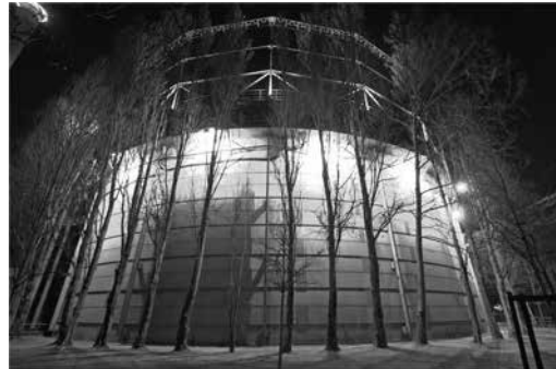
Fig. 5.: Duisburg gas tank, where underwater space was built, (Source: http://www.tauchrevier-gasometer.de )
