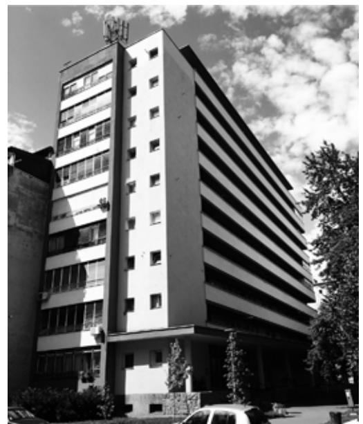
Fig. 11.: The compound of gallery CABs at the perimeter of the block Crvenog Križa St-Vrbanićeva St-Nodilova St-Kneza Ljudevita Posavskog St, modulated with the CAB tower, 6 Vrbanićeva St. A successful derivation of the famous "Bergpolder" apartment tower, in reinforced-concrete instead of metal skeleton. NE corner, recently refurbished in accordance with EU Directives. Arch.: Peroslav Ilijić, 1953-56? (Photography: Darko Kahle)
