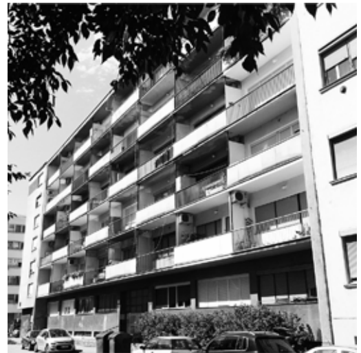
Fig. 10.: The gallery attached apartment building, 24 Crvenog Križa (Red Cross) St, well preserved street front. Arch.: Peroslav Ilijić, 1953-56? (Photography: Darko Kahle)
