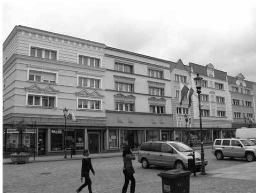
Fig. 3.:Zary - old town district. Southern frontage of main market square. Styrofoam and acrylic decorations made to hide the modernist character of post-war architecture. An example of wrong actions to bring back the character of historical area. (Source: Author 2013.)
