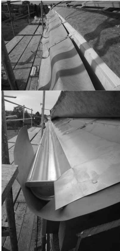
Picture 4,5.: Photos of construction progress (Source: 3AE s.r.o.)
