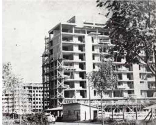
Fig. 8.: 11s, 2Aps, "Exportdrvo" CHB in the building phase: the pre-WWII building process of reinforced-concrete construction and brick filling, with scaffoldings and without the cranes. 62A-D Grada Vukovara St. Arch.: Prof. Božidar Rašica, 1953-54? (Source: [15], p. 33)
