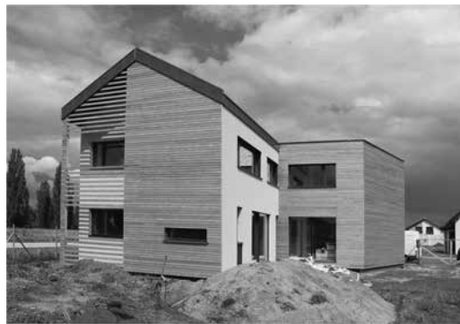
Picture 1: Actual photo of facade and gutter (Source: M. Pavlas)
