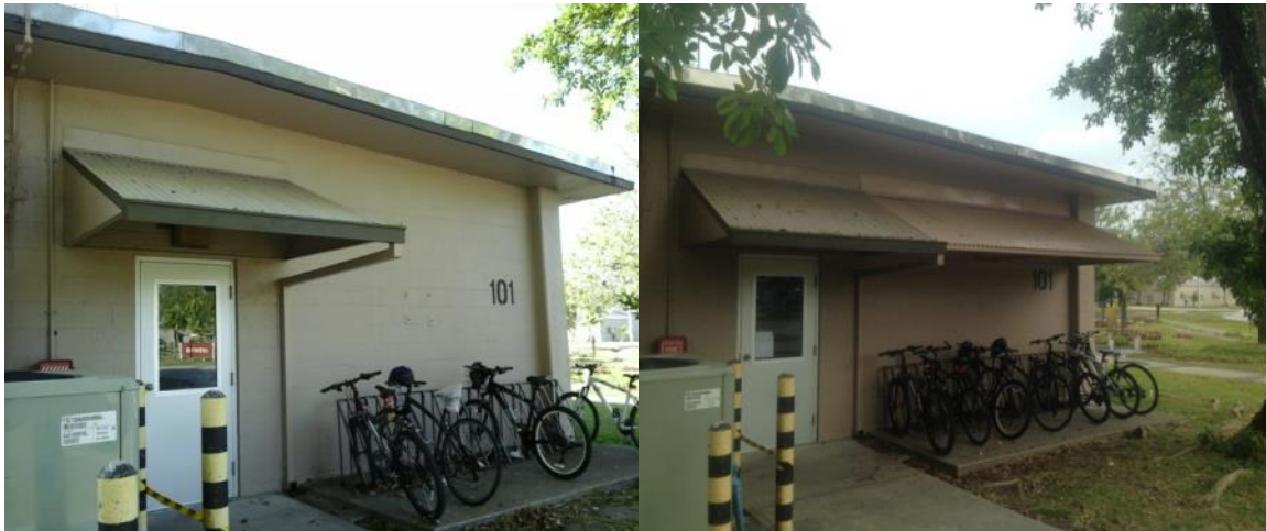
Prior to Installation
