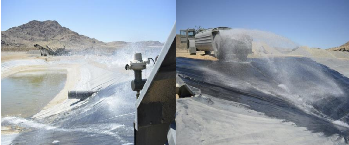
One of the ponds being filled showing connecting pipe
