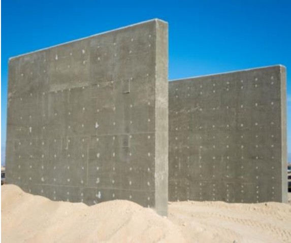
View of headwall prior to demolition
