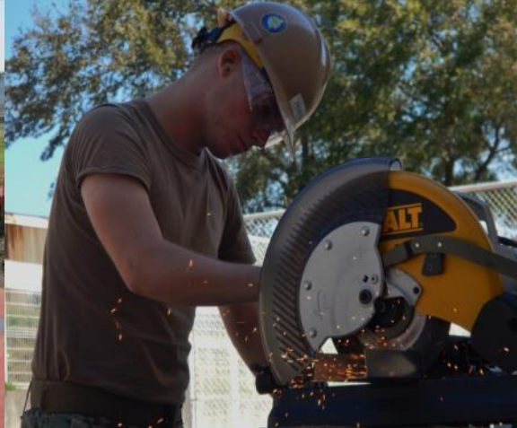
BUCA Pedersen cuts metal track
