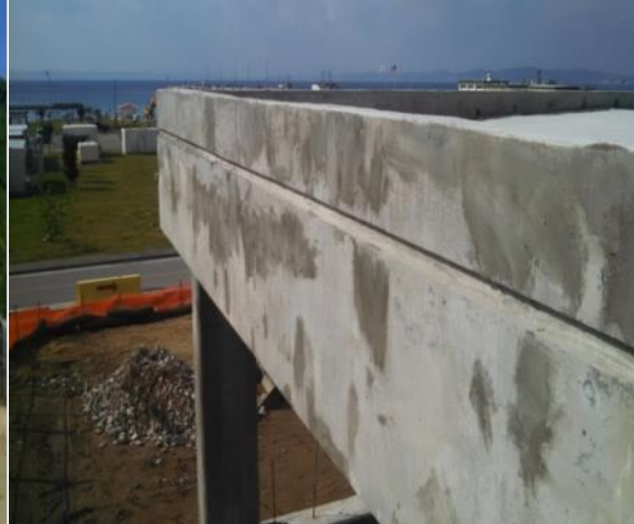
Repaired parapet
