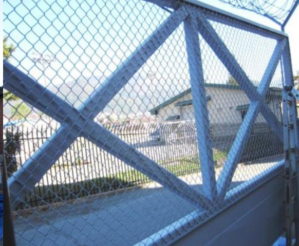
Front side of Finished Gate
