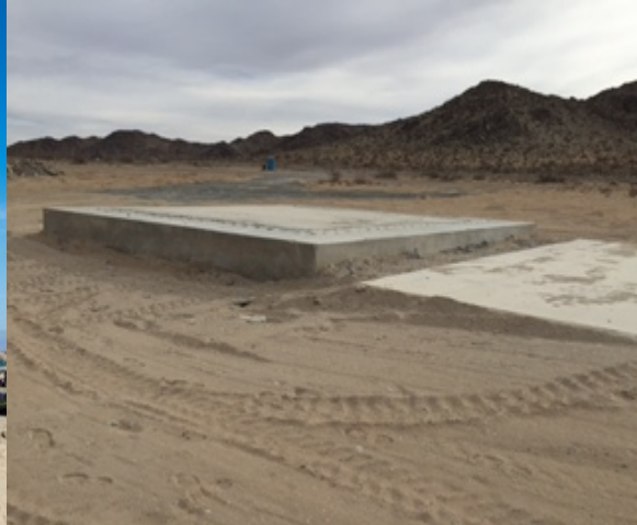
View of existing pad after demolition of Headwall
