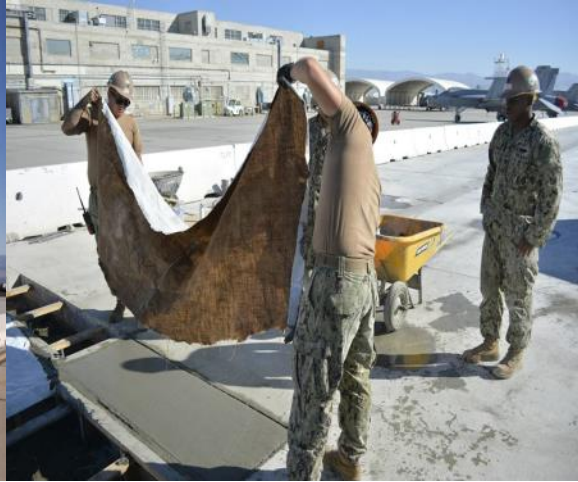
Concrete placement in northwest corner
