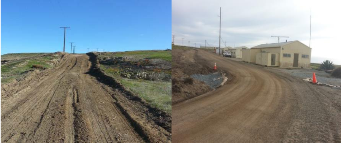
Typical Road Prior to Grading
