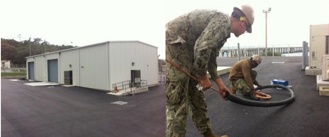
Tengan Pier Facility site overview
