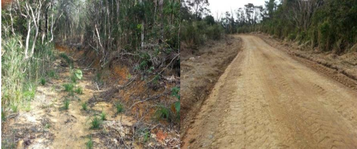
Range 10 road prior to construction
