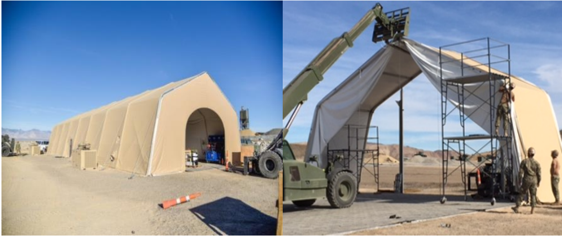
View of Tension Fabric Structure Prior to Disassembly
