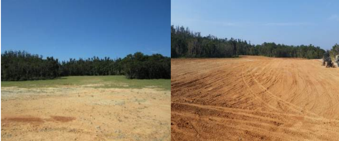
LZ Falcon before earthwork
