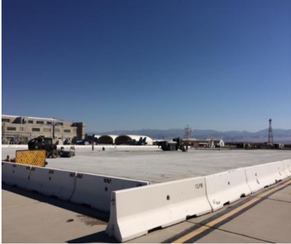
View of Apron from the southwest corner
