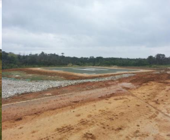
Landing pad after AM2 placement
