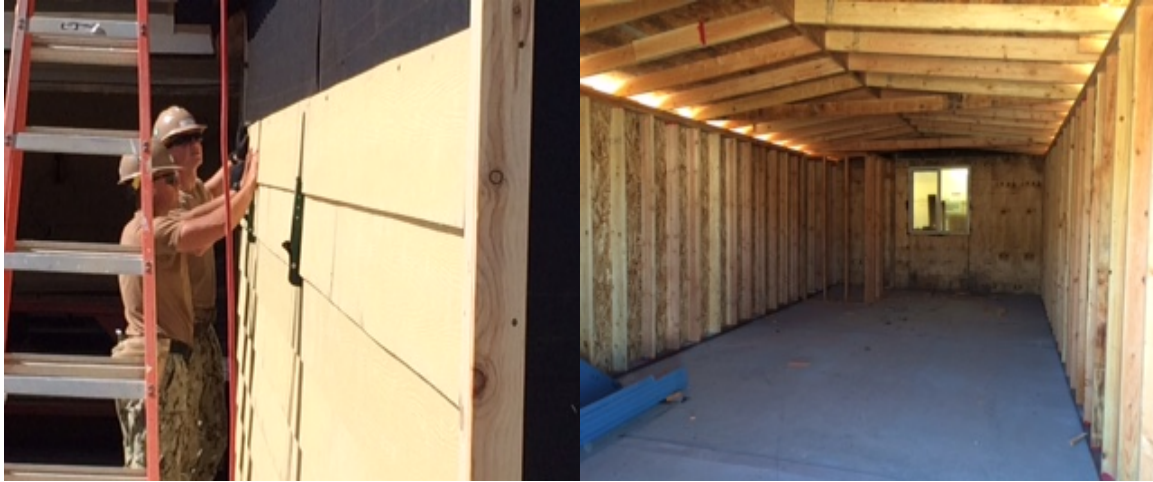
Siding to the Builder shop build out for MAROPS.
