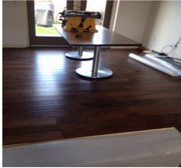
The inside of the CPO mess completed wood floor.
