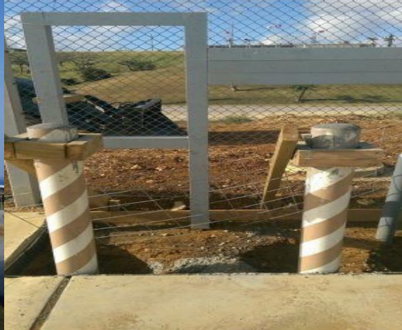
Bollard Installation
