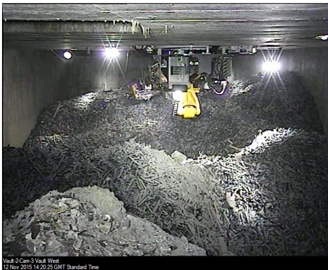
Figure 3. Berkeley Fuel Element Debris Vault 2: Beginning of retrieval operations (left) and after removal of 88 Te of FED (right).
