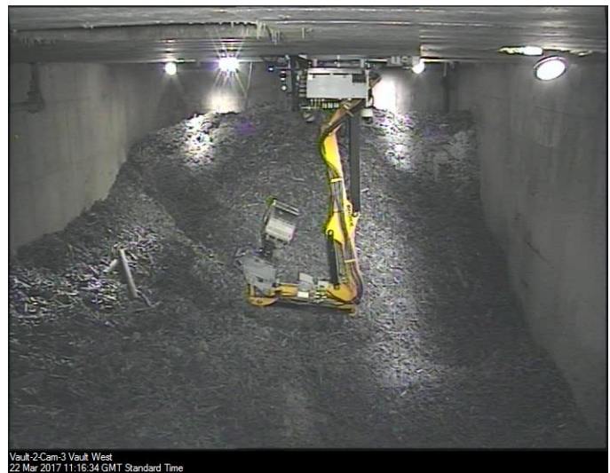
Figure 3. Berkeley Fuel Element Debris Vault 2: Beginning of retrieval operations (left) and after removal of 88 Te of FED (right).
