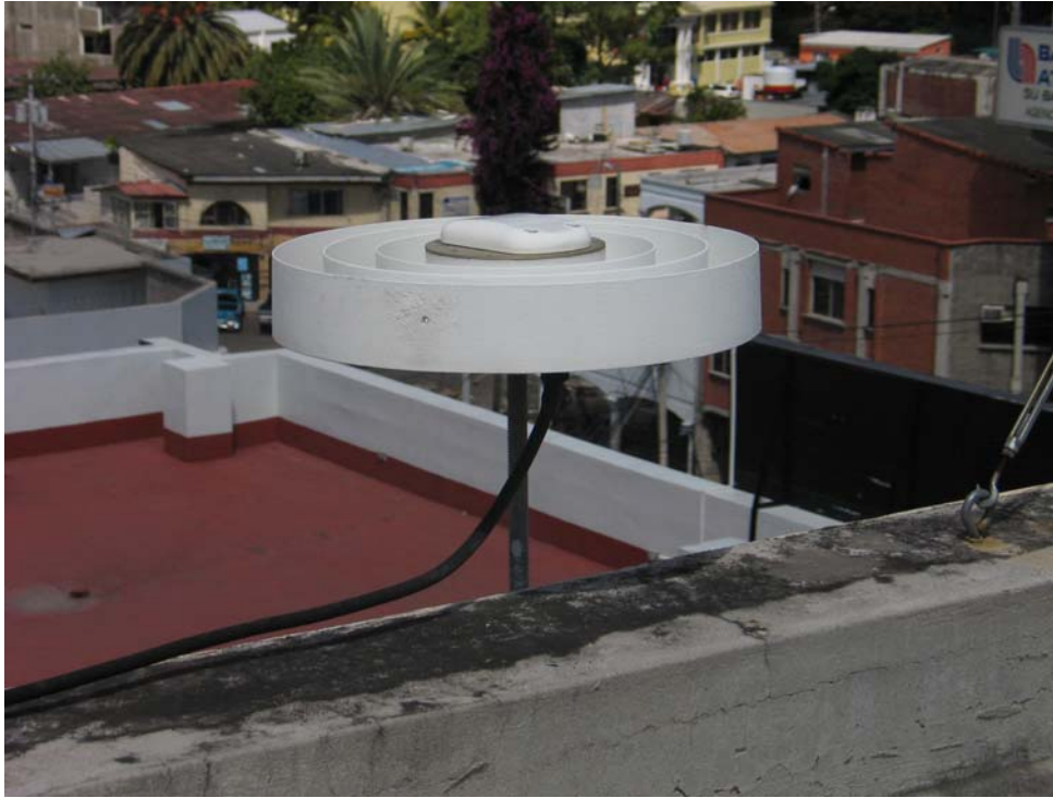
GPS Antenna Tegucigalpa Honduras
