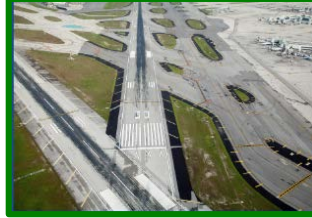
Miami International Airport Runway Rehabilitation
