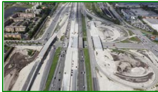
SR 836 WESTBOUND BRIDGES AT 87TH AVENUE
