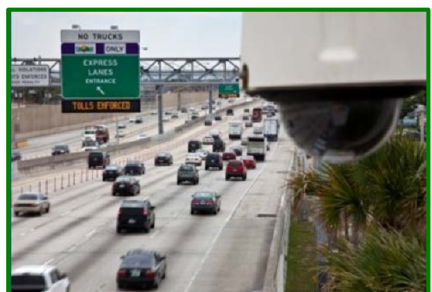
I-95 Express Lane Toll Sign
