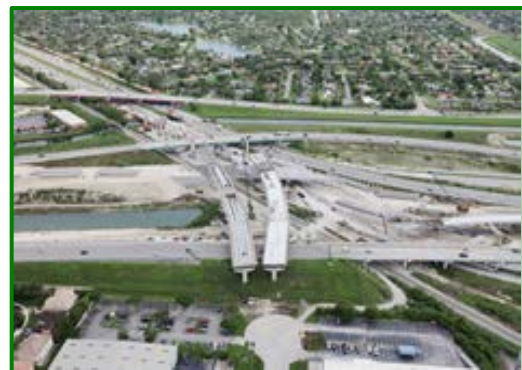
SW 128TH STREET APPROACHING SR 874 RAMP CONNECTOR
