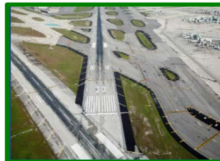
Miami International Airport Runway Rehabilitation
