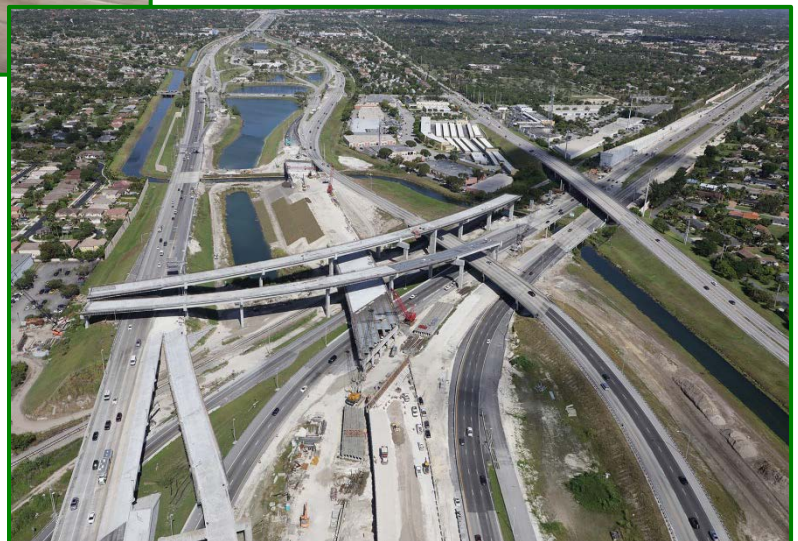
Widen SR 821 Eureka Drive to Killian Pkwy – Design Build
