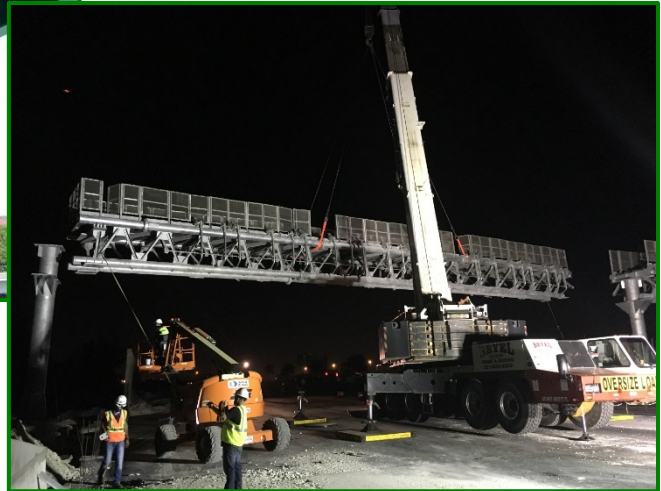
SR 821 Toll Gantry Installation North of Bird Road
