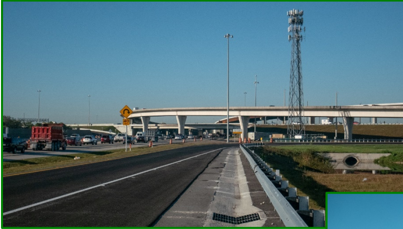
Widening SR 821/Turnpike's Extension @ I-75
