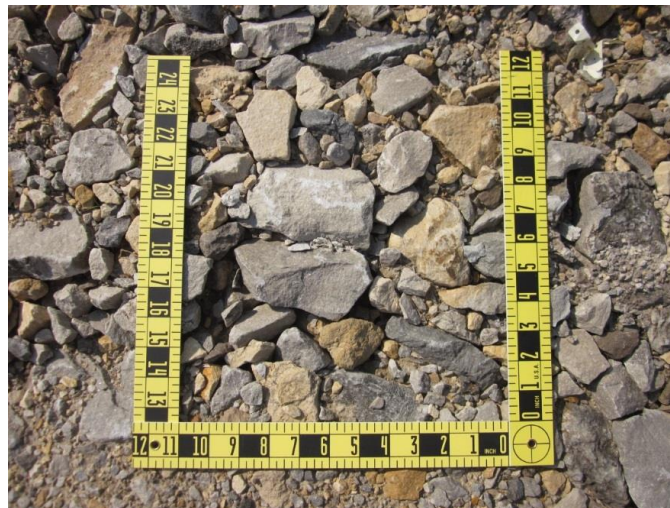
Figure 17. Macadam subbase material (picture from County Road D20 in Hamilton County, April 2012)
