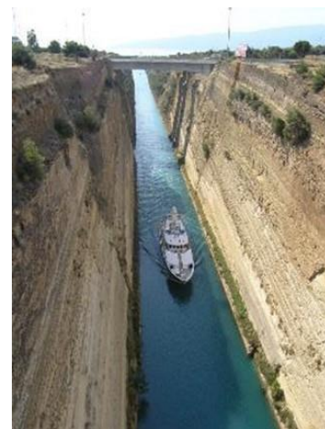
Fig. 4.14. Corinth Canal in Greece (completion in 1893).
