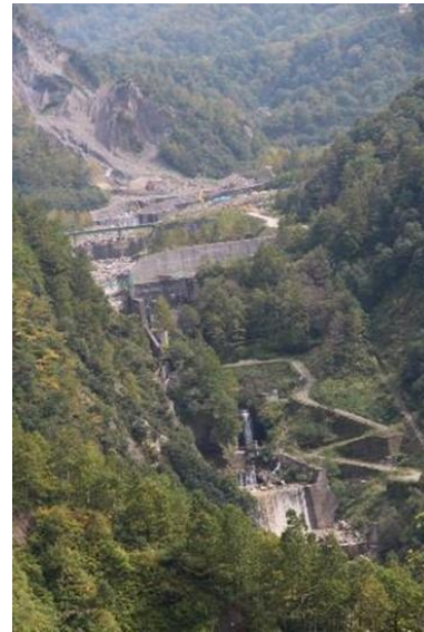
Fig. 4.13. Shiraiwa erosion control dam in Tateyama Caldera, Japan (completion in 1939).
