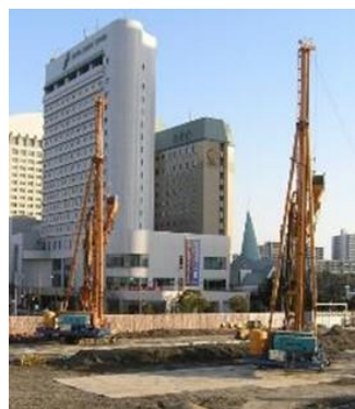
Fig. 4.45 (a). Contrast between densified and untreated parts of a sand compaction project (2011). Machines for densification of loose sandy subsoil
