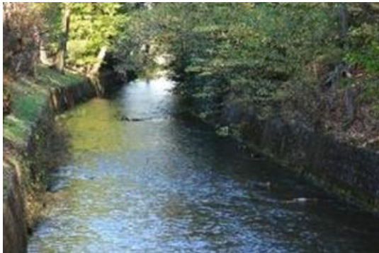
Fig. 4.3. Tamagawa canal that provided water to present Tokyo, constructed in 17th Century
