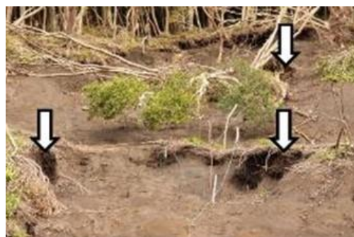
Fig. 6.3. Many piping holes from which ground water was ejected during heavy rainfall-induced landslide (Izu Oshima Island, Japan, in 2013), indicating complex geological-geotechnical-geo-hydrological system.
