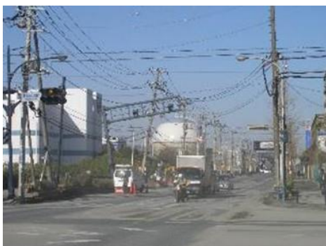
Fig. 4.44. View after liquefaction disaster; see road undulation, ejected sand on pavement and tilting of structures (after 2011 Tohoku earthquake).
