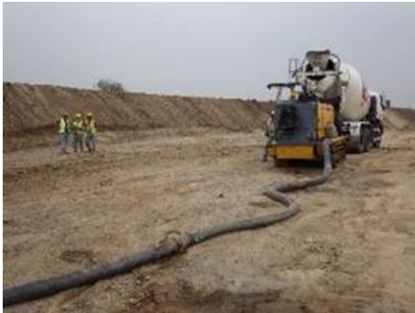
Fig. 4.31. Ground improvement for expansion of the international airport in Jakarta, Indonesia.
