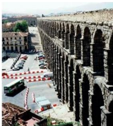
Fig. 4.22. Masonry aqueduct crossing a valley in Segovia, Spain (early AD 2nd Century, Roman Period).
