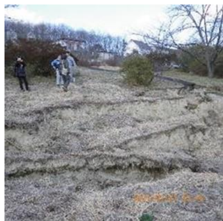
Fig. 4.42 (a). Effects of drainage of ground water (removal of water) from an unstable slope during the 2011 Tohoku earthquake of Mw=9.0 in Shiroishi, Japan. Failure of slope without geotechnical mitigation
