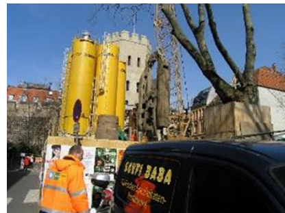
Fig. 4.37. Ground improvement prior to excavation (Köln, Germany).
