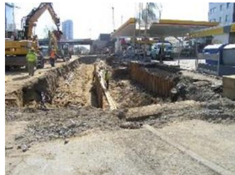
Fig. 4.36. Construction of new underground tram (Köln, Germany).
