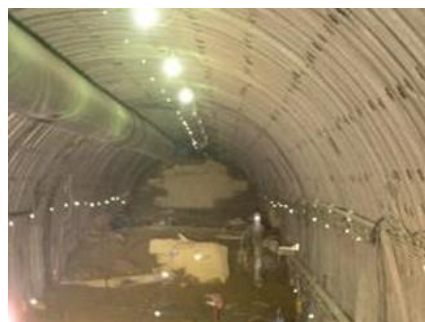
Fig. 4.28. Seikan submarine railway tunnel with total length = 53.85 km (completion in 1988).
