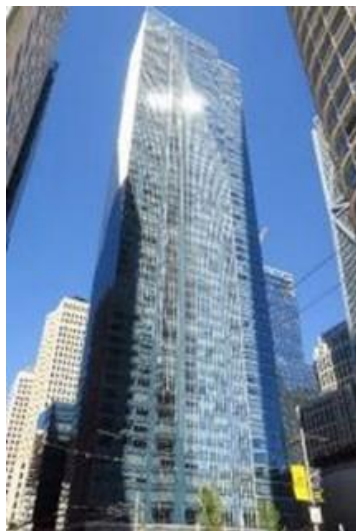
Fig. 3.1. Leaning of a skyscraper in the center of a mega city.
