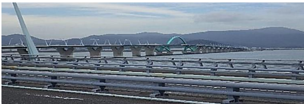
Fig. 3.9. Bridge connecting the Kitakyushu Airport Island with the mainland.
