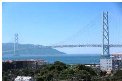
Fig. 4.25. Akashi Strait Bridge with its central span = 1991 m (completion in 1998).
