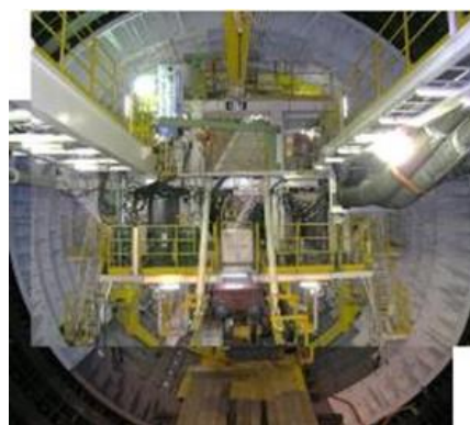
Fig. 4.27. Shield tunnelling for urban motorway in Tokyo.
