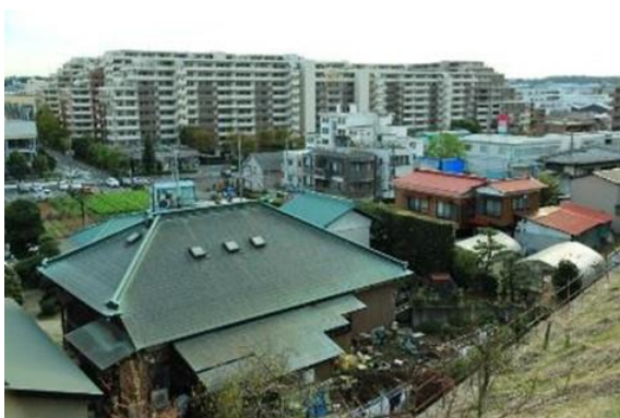
Fig. 3.2. Minor tilting of a condominium building whose reconstruction cost US 400 million $ to the contractors and the developers.
