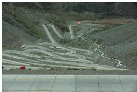
Fig. 4.21. Highway crossing Los Andes at Portillo in Chile.
