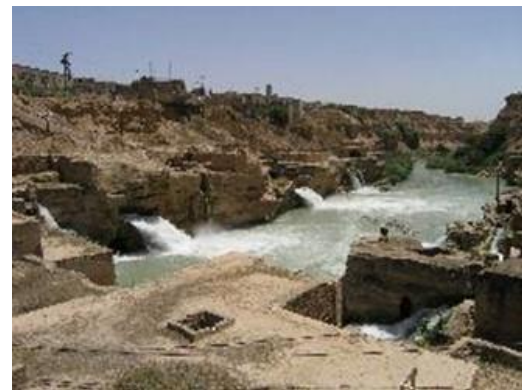
Fig. 4.6. Shushtar Irrigation Hydraulic System, Khuzestan, Iran (AD 3rd Century).
