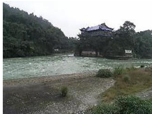
Fig. 4.5. Spillway at water intake of Dujiangyan, Sichuan Province, China (BC 3rd Century), from River Minjian
