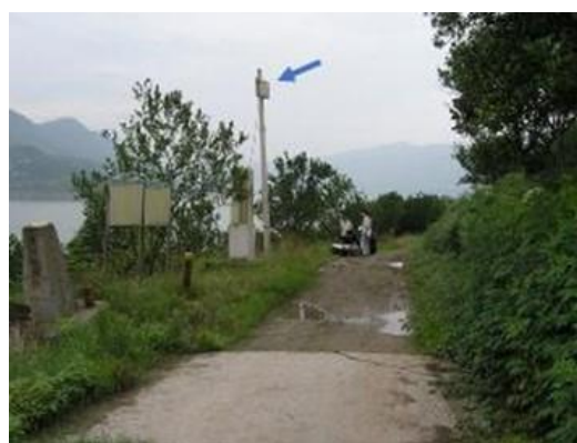
Fig. 4.50. Slope monitoring with sensor atop the pole, aiming to foresee landslide and promote emergency evacuation (China).
