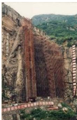
Fig. 4.48. Rock mass reinforcement prior to construction of Three Gorge Dam, China.
