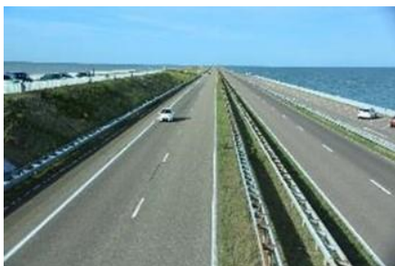
Fig. 4.38. Afsluitdijk in the Netherlands that produced a fresh-water lake disconnected from the North Sea (32 km long and completion in 1932).
