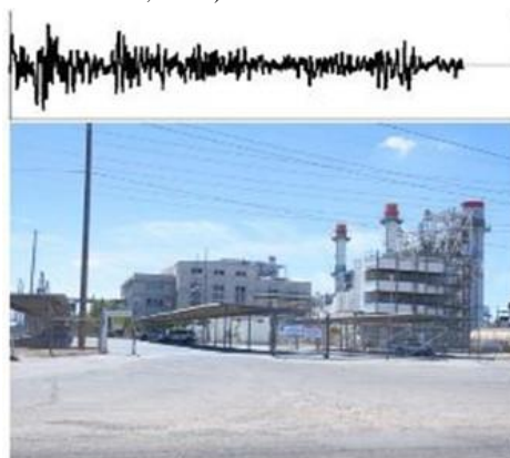
Fig. 6.5. Site of famous strong earthquake motion records in El Centro, USA
