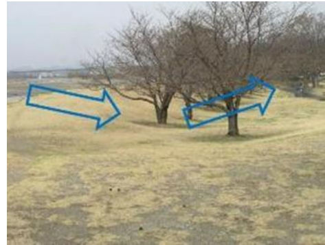
Fig. 4.40. Intention of overtopping of flood water into a retention basin schematically illustrated by arrows (Midai River, Japan, 16th Century).
