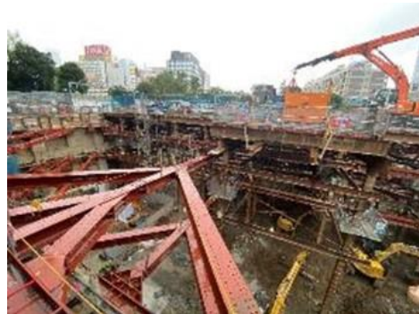
Fig. 4.34. Deep excavation for foundation of a new building (Yokohama, Japan).
