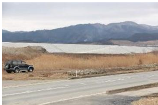
Fig. 4.54. High sea wall in Rikuzen Takata constructed after the disaster in 2011 (2 km long and 12 m high).
