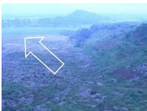
Fig. 5.7. Municipal waste landfill of Leuwigajah in Bandung, Indonesia, that failed in 2005 during heavy rain and claimed 143 lives.
