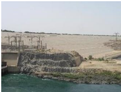
Fig. 4.11. Aswan High Dam in Egypt made of rockfill (completion in 1970).
