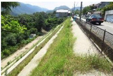
Fig. 4.43. Slope reinforcement to protect residential development from earthquake landslide (Takaradzuka, Japan).
