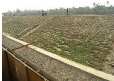
Fig. 4.57. Embankment used for cyclone shelter in the coastal area of Myanmar
