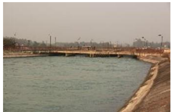
Fig. 4.7. Ganges Canal for irrigation in Uttarpradesh, northern India (construction in late 19th Century).
