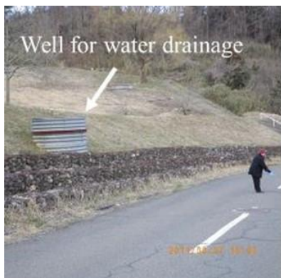
Fig. 4.42(b). Effects of drainage of ground water (removal of water) from an unstable slope during the 2011 Tohoku earthquake of Mw=9.0 in Shiroishi, Japan. Successful drainage and slope stabilization next to the damage site in (a)
