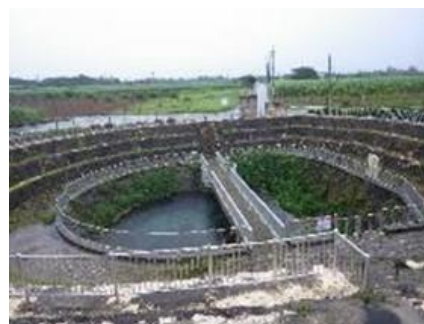
Fig. 5.10. Monitoring of underground reservoir water in Miyako Jima Island, Japan.
