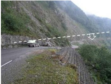
Fig. 6.7. Creeping rock slope in Bhutan.
