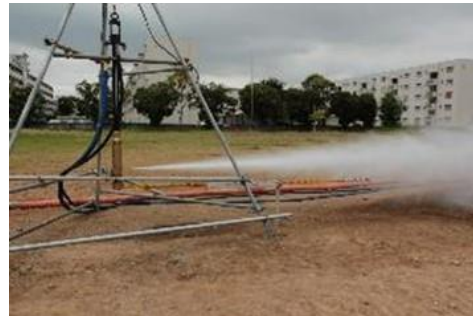
Fig. 4.46. Small jet grout machine for soil improvement in a narrow space.
