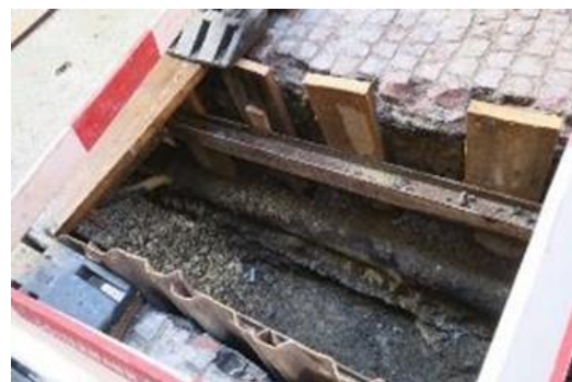
Fig. 4.8. One small piece of urban lifeline network undergoing maintenance (Zurich, Switzerland).
