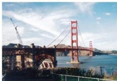
Fig. 4.24. Epoch-making Golden Gate Bridge with its central span = 1280 m (completion in 1937).
