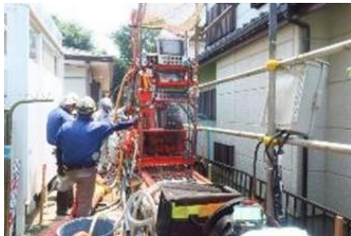
Fig. 4.47. Ongoing jet grouting in a narrow space between houses (Urayasu, Japan).
