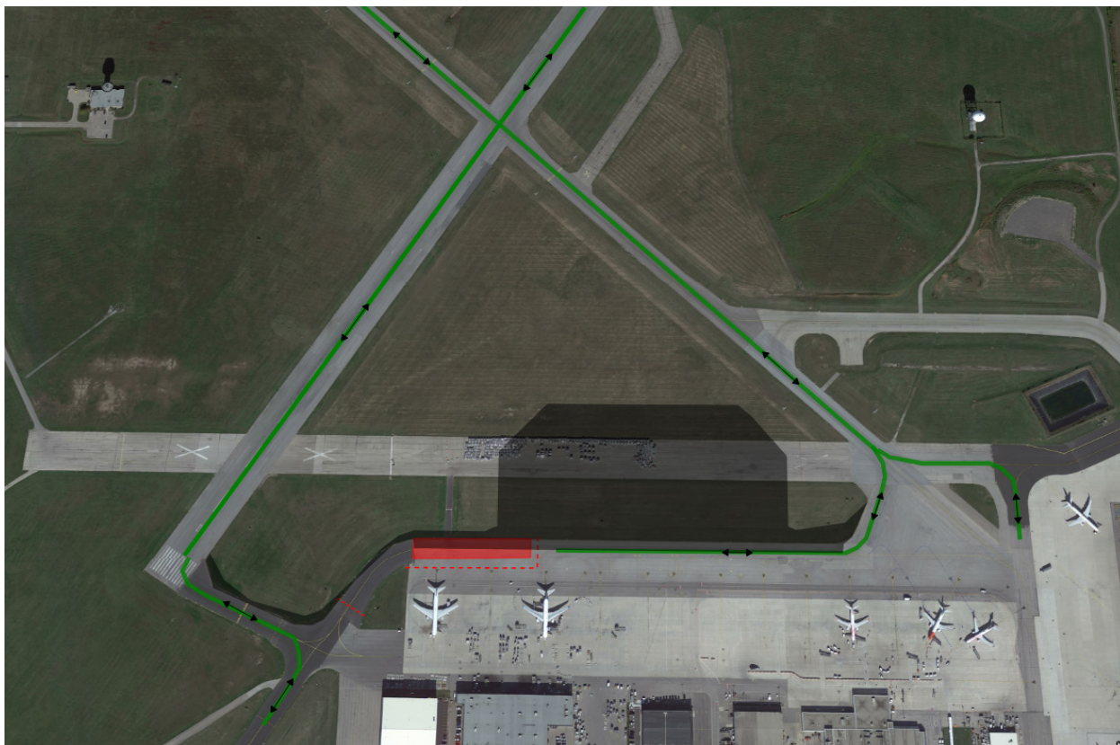
Figure 10: Apron II (Phase 7D)
