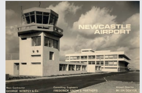
The 1960s and 1970s brought rapid growth to the Airport
