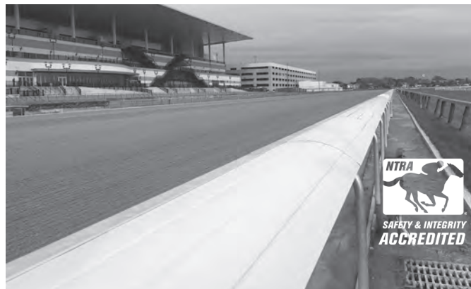
The new safety rail on the Aqueduct main track, the first of its kind at a NYRA track and one of several safety-enhancing capital improvements NYRA has undertaken since 2013.
