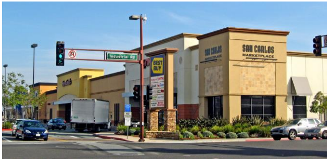
Commercial development in East Side area
