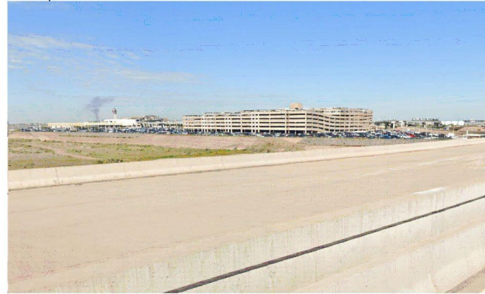
View #5: S. 44th Street bridge over the Salt River looking west towards the Airport
