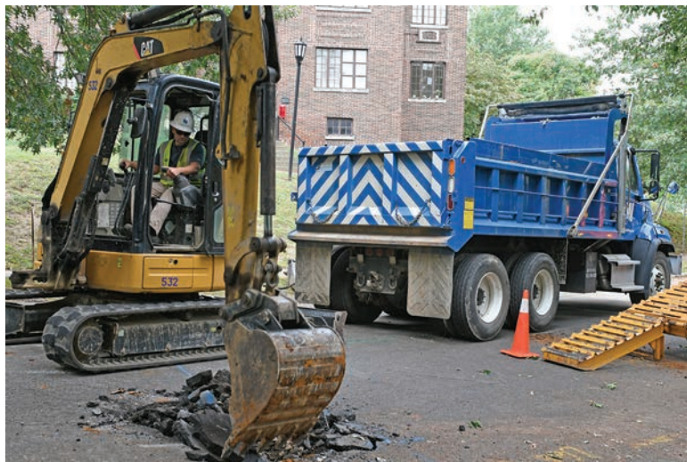
Louisville Water has systematically replaced all lead water services on the utility side of the meters.
