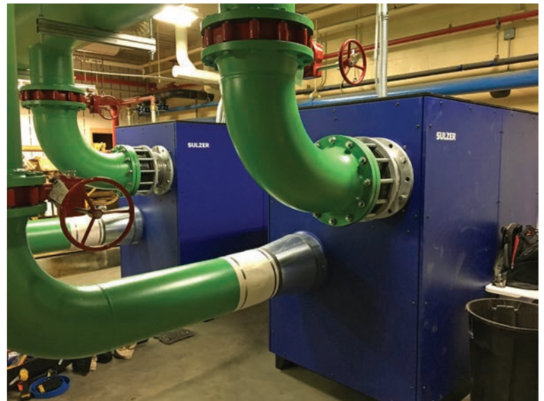
ABOVE: Two Sulzer magnetic bearing blowers replaced four old blowers at the Beaver Dam Wastewater Treatment Plant. LEFT: The biological treatment process includes extended aeration.
