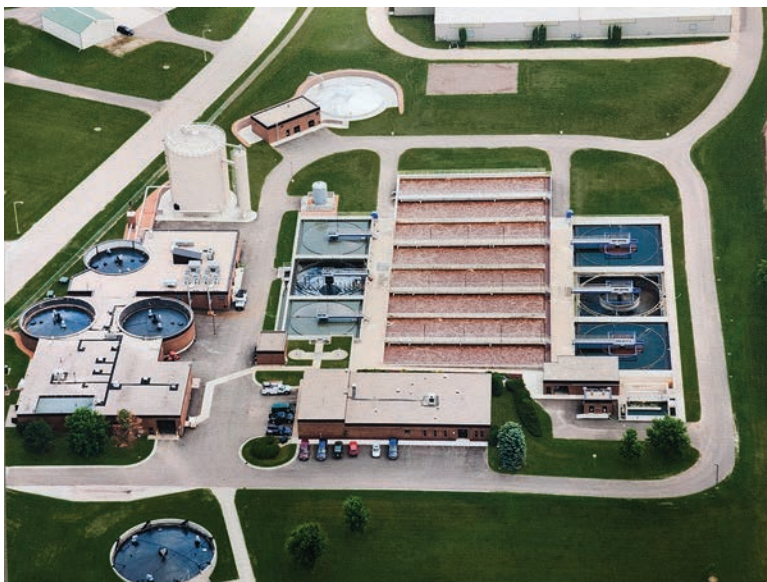
The Beaver Dam Wastewater Treatment Plant has a 5.5 mgd design flow and treats 4 mgd on average.
