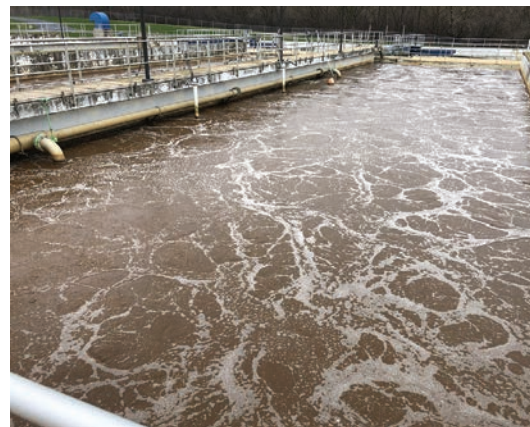
ABOVE: Two Sulzer magnetic bearing blowers replaced four old blowers at the Beaver Dam Wastewater Treatment Plant. LEFT: The biological treatment process includes extended aeration.
