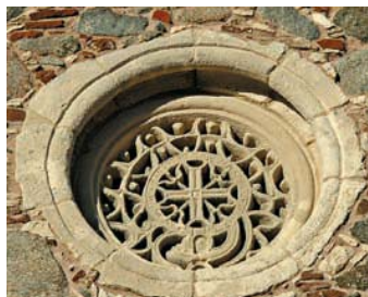
Fig. 384. Detail of window Church of Agios Georgios, Kellaki.
