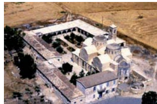
Fig. 222. Aerial view of the Monastery of Apostolos Varnavas in occupied Engomi, Ammochostos.
