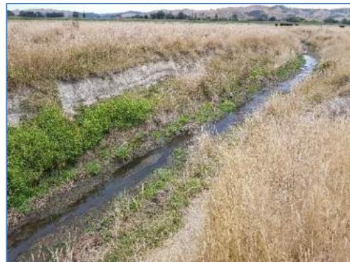
Figure 3 Existing surface drain
