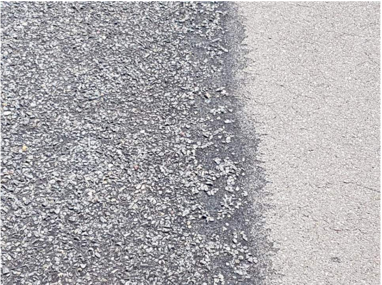
Photo showing Grade 3/5 chipseal and AC surfacing
