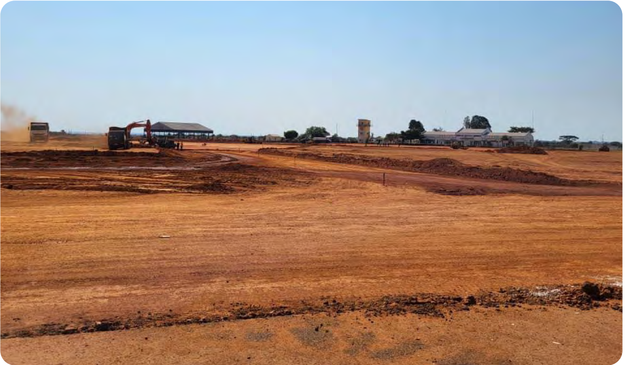
Ongoing Works on Kasama Airport Apron
