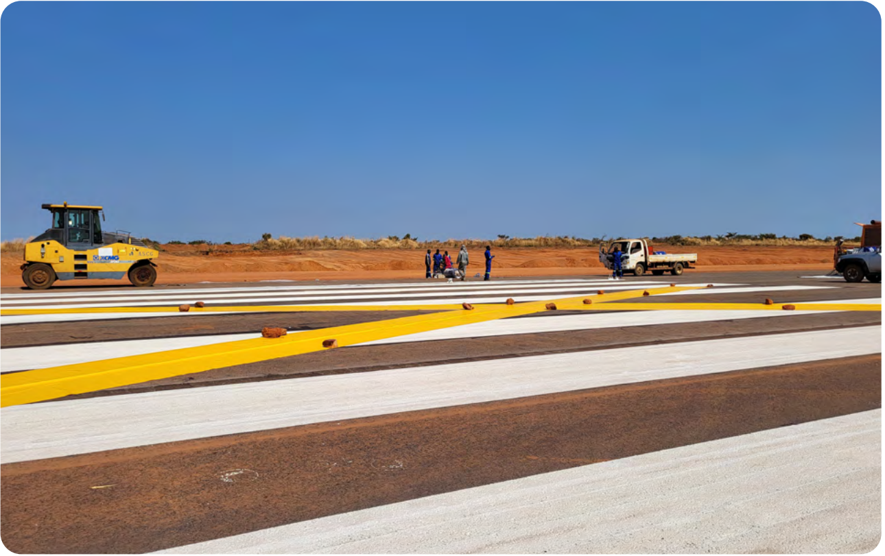
Ongoing Works on Kasama Airport Runway
