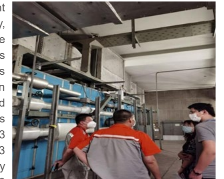
Ventilation system upgrading
